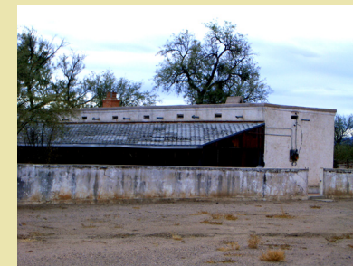
The Foreman's House, 2005
