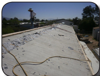
Roof Repair, Insulation
