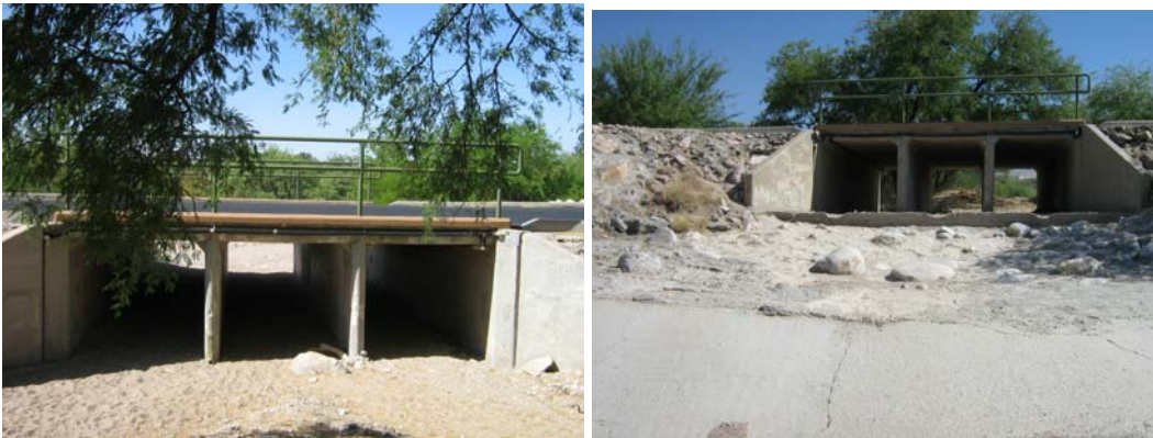
Photo 1. Culvert at Tanuri Drive (left: upstream, right: downstream)
