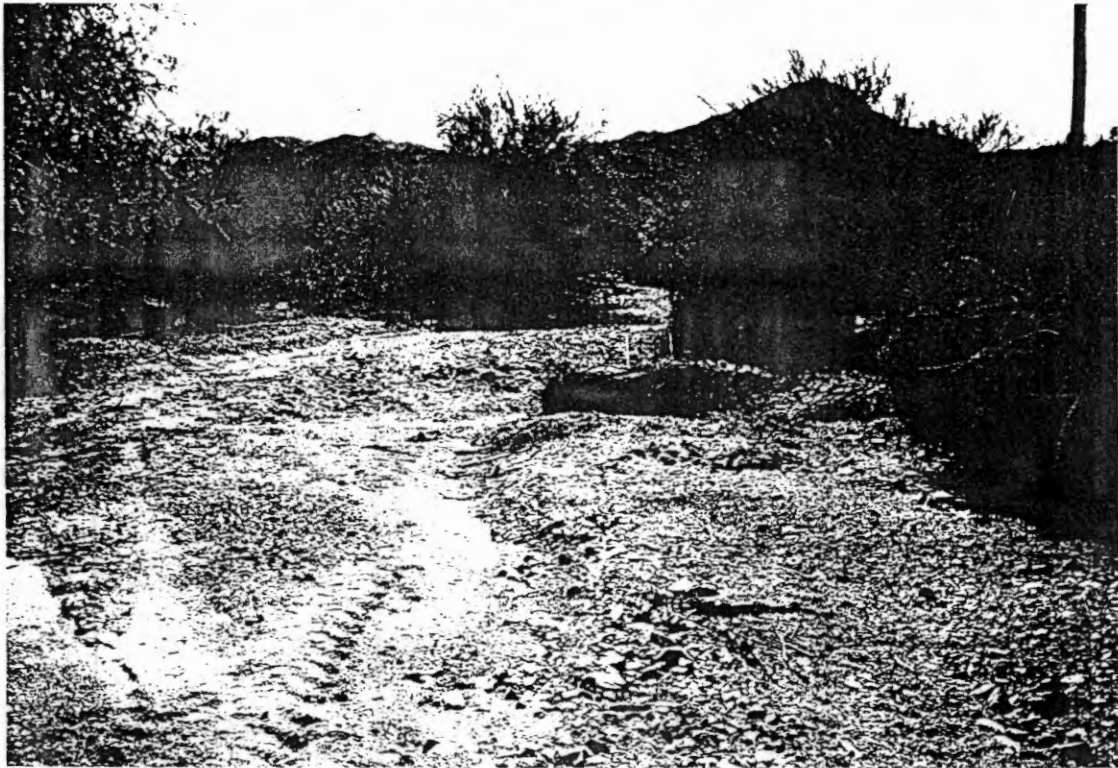
Looking upstream (southwest) along first braid east from the main channel where the braid joins the main braid or channel approximately 150 feet downstream of El Camino Del Cerro.
