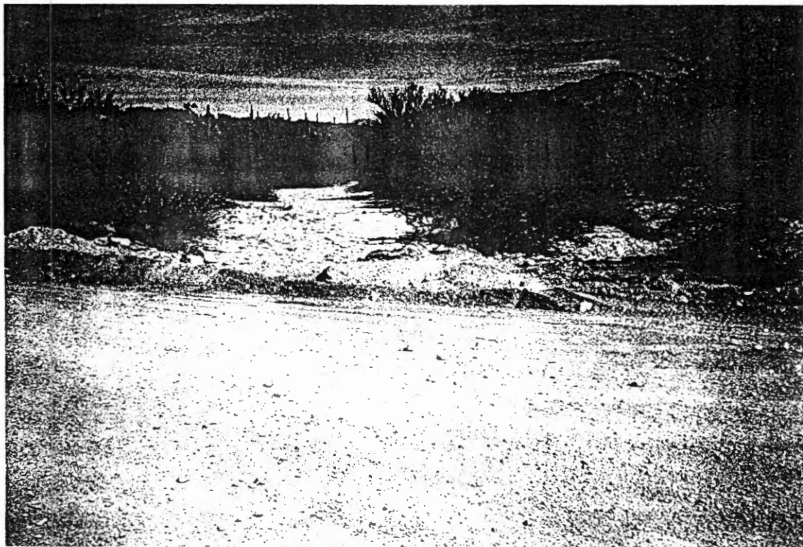
Looking downstream (east) along a tributary at Gerhart Road. The tributary drains Drainage Area E below Concentration Point 6.
