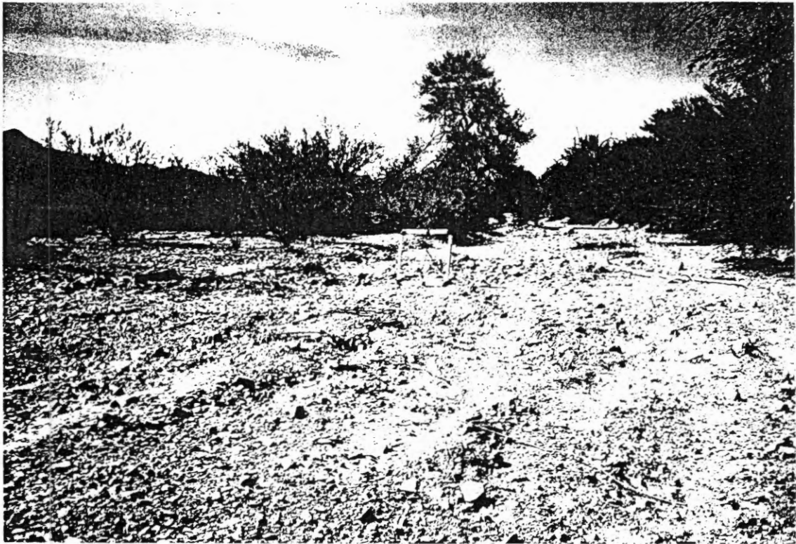
Looking upstream (west) along the main channel from approximately 150 feet upstream of the underground pipeline crossing.
