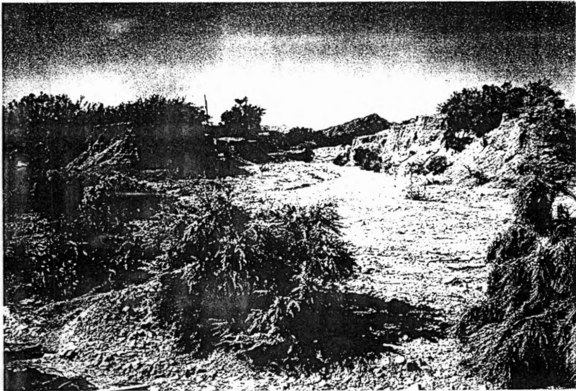
Looking upstream (west) along the breakout collector channel from approximately 650 feet downstream (west) of Silverbell Road. Photo taken standing at the west low-flow bank of the Santa Cruz river.
