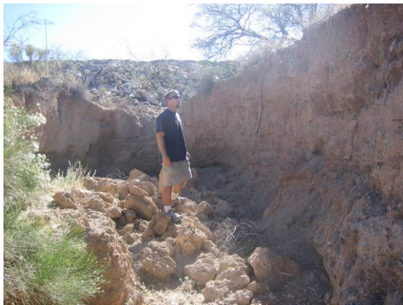
Erosion in channel, facing Rd. (LM02-46-06)
