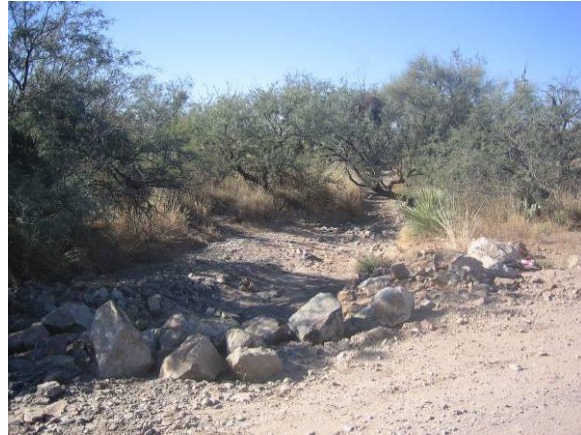
Rip rap along Salero View Road, north of Toro Bronco, Qy surface (LM02-55-01)
