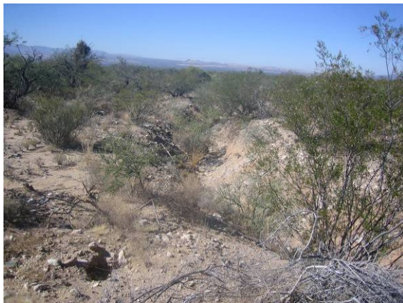
Ground view of headcut (LM01-36-01)
