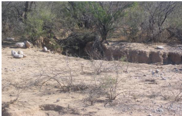
Vertical scour on Qy surface (LM03-40-01)
