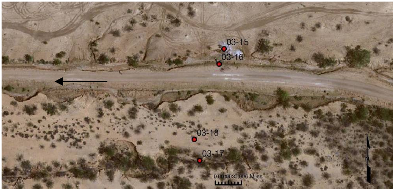
Aerial view of erosion along flow paralleling dirt road
