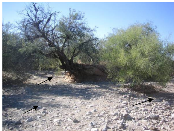
Scour on upstream end of channel island (LM01-51-02)
