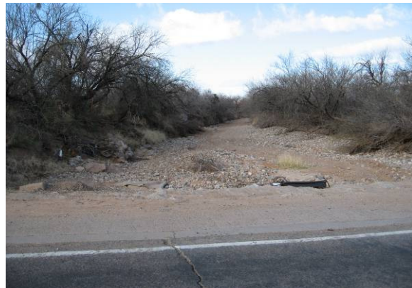
Degradation downstream of Highway, T2 surface (LM04-04-01)
