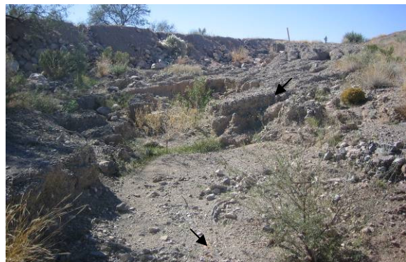
Vertical erosion downstream of Road, facing road, on QTs surface (LM02-43-05), facing southwest
