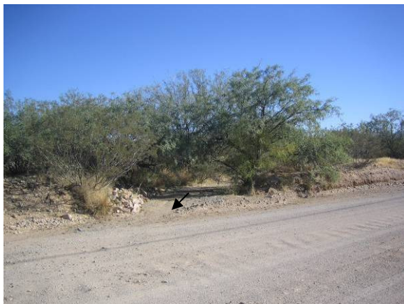
Wash upstream of Salero View Road, draining across road (LM02-52-02)
