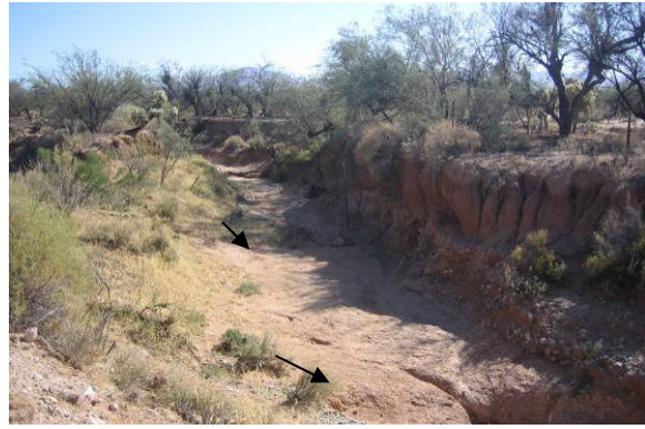
B - Upstream view of headcut, nick point in lower right of frame (LM03-59-01)
