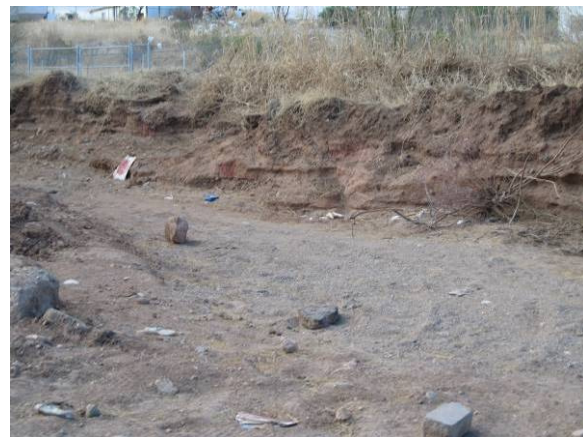
Trash and vertical scour on Franco Wash upstream of Summit Street, Qy surface (LM04-06-02)
