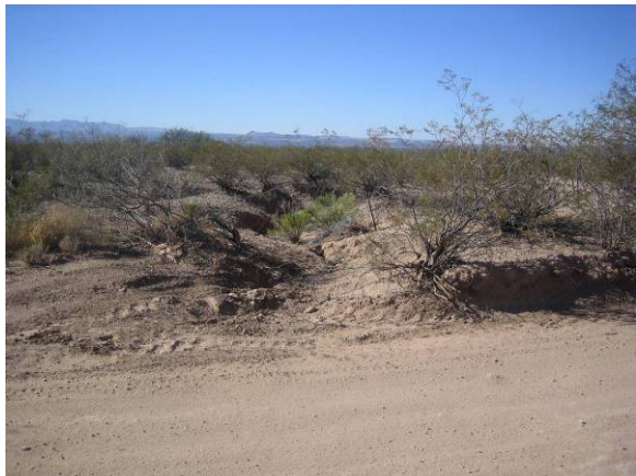
View downstream from Wilmot Road in headcutting channel on M1/M2 surface (LM01-48-04)
