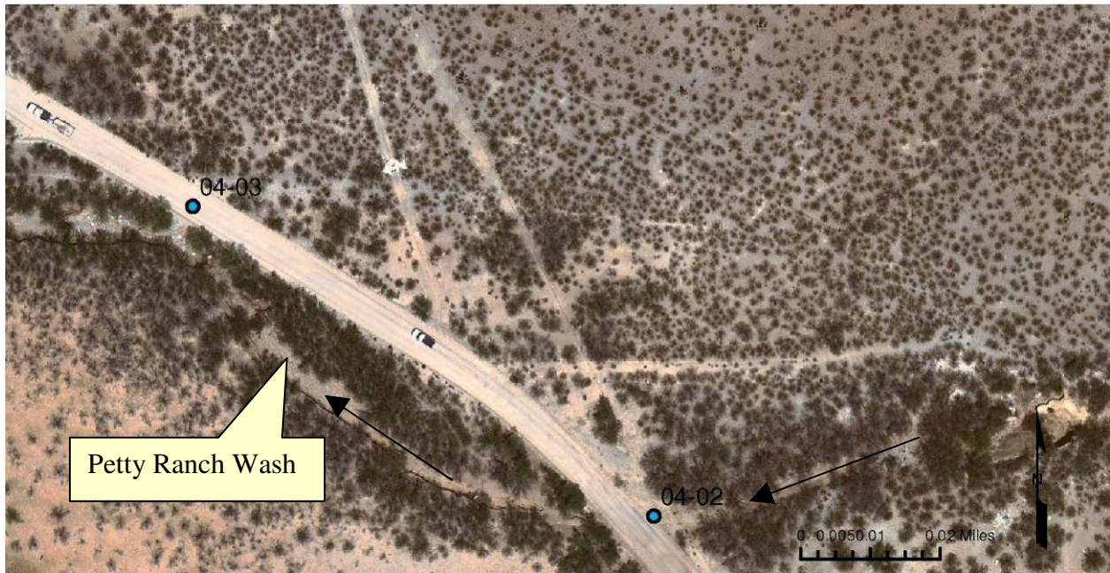
Aerial view of Petty Ranch Wash crossing of Old Nogales Highway
