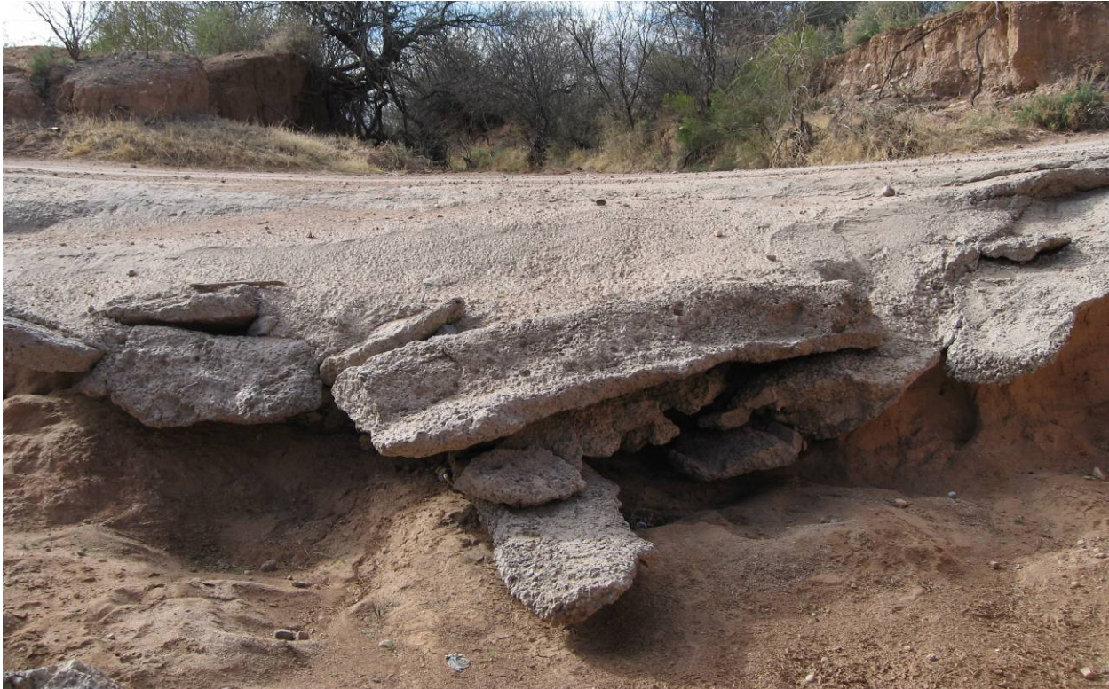
Facing south towards concrete ford crossing, (LM04-12-07)
