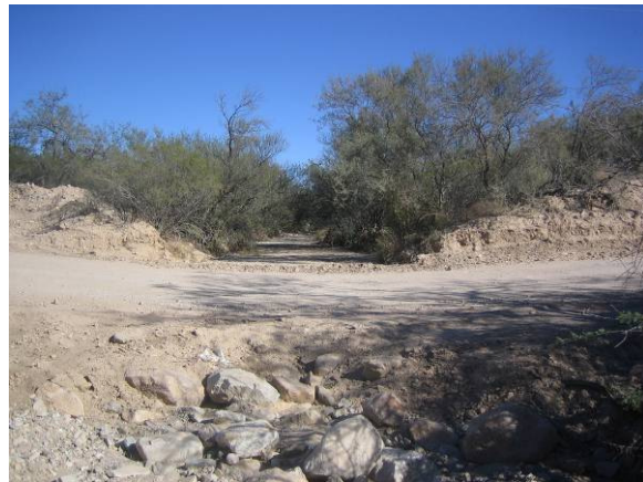
Well vegetated, sloped banks upstream of road (LM01-49-01)
