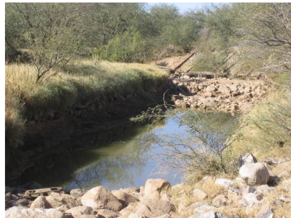
Riprap within Fagan Wash (LM03-33-02)
