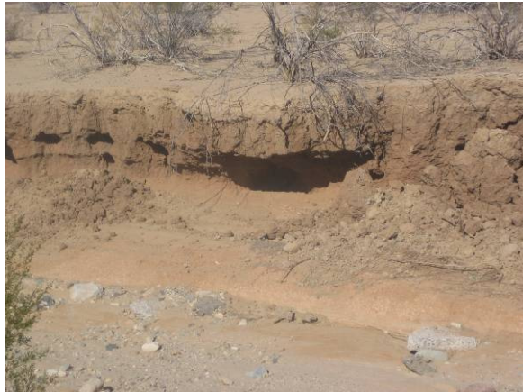
C - Widening and undercutting of terrace vegetation (LM03-51-01)
