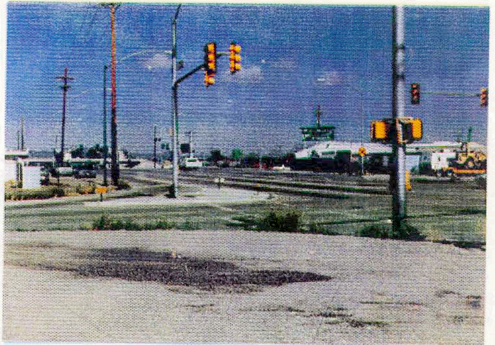
Redesigned intersection of Ruthrauff Road and Highway Drive.
