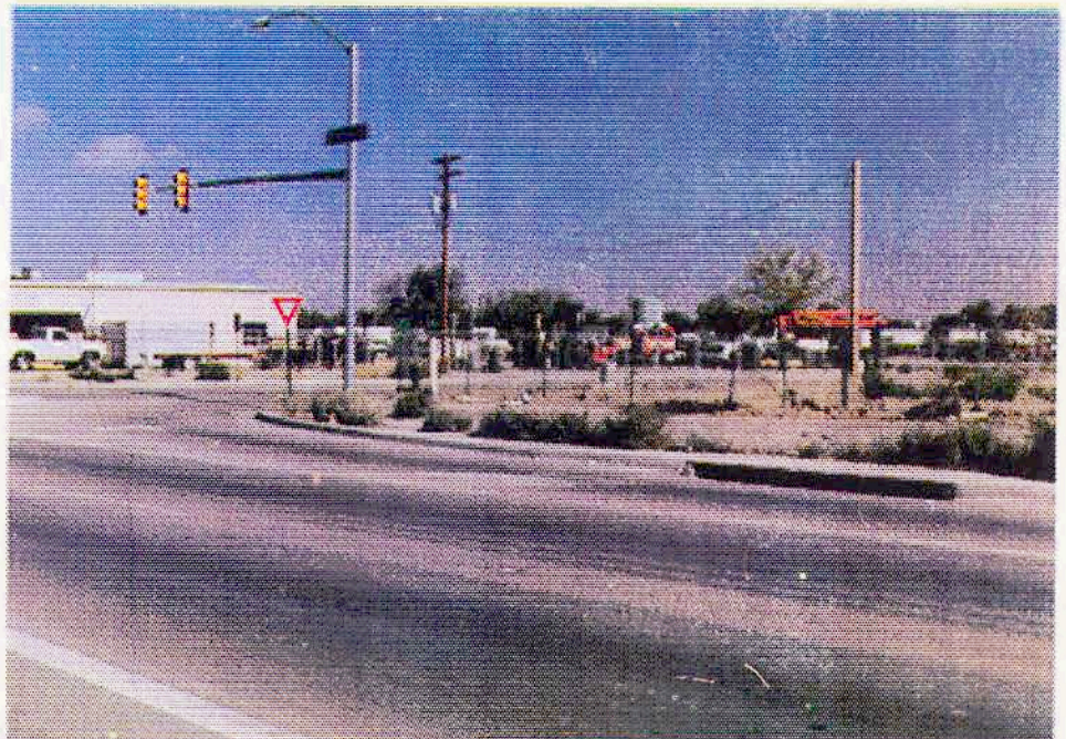
Catch basin leading to Ruthrauff Road Storm Drain.
