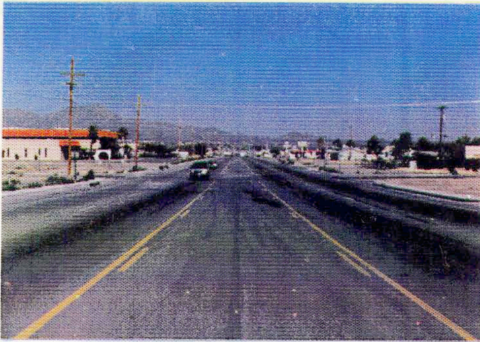
Roadway improvements and storm drain system.
