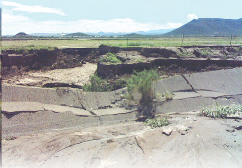
Storm damage from August 23, 2005 storm, west branch channel upstream of Valencia Road. (Left) Looking southwest towards Black Mountain. (Right) Looking south towards San Xavier Mission.
