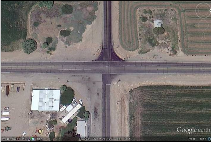
Figure 31: Aerial View of Mohave Road/Agnes Wilson Road Intersection
