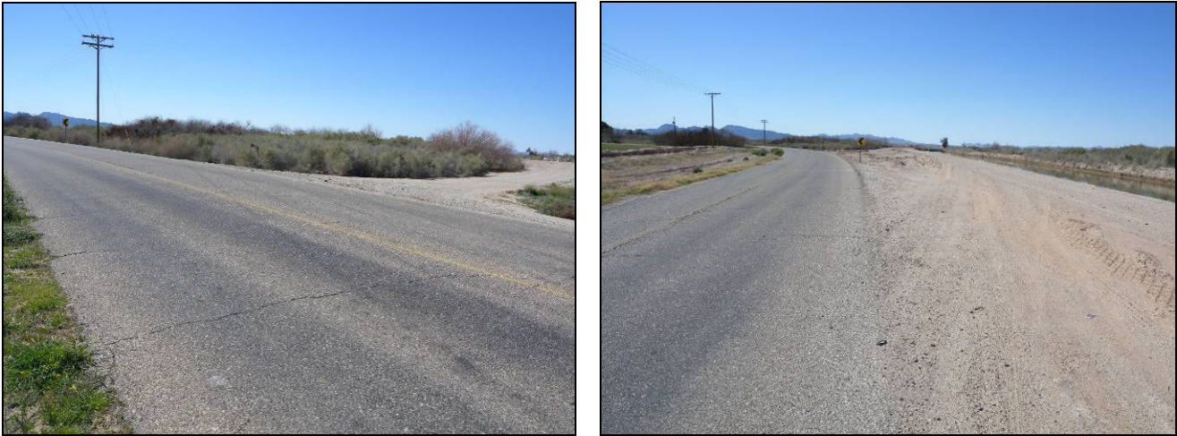
Figure 20: Unpaved Accesses Leading from 4th Avenue/Booth Road to Canal Roads
