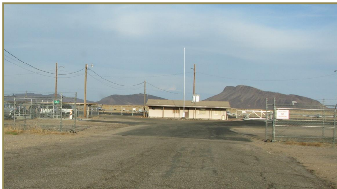
Entrance to the Avi Suquilla Airport- note pavement improvement needs in foreground
