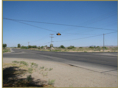
Flashing beacon at Mohave Road / 2 nd Avenue
