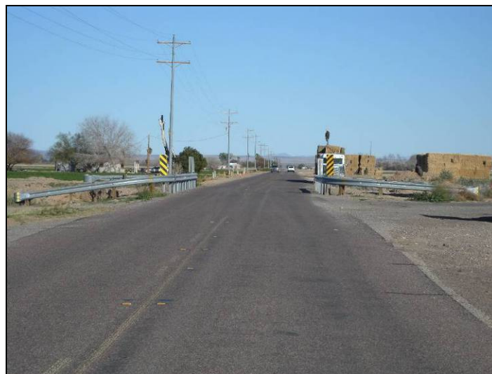
Figure 14: Narrow Bridge Near 12 th Avenue
