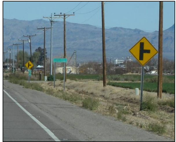
Figure 32: Closely Spaced Intersection Warning Signs for Eddy Road and 9 th Avenue
