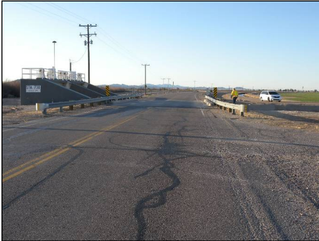
Figure 29: Southbound Mohave Road Approach to Patrick Road Canal Crossing
