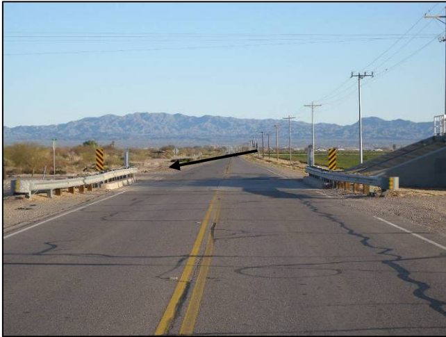
Figure 25: Northbound Approach to Patrick Road Intersection
