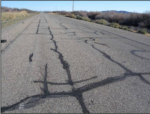
Figure 3: No Pavement Markings on Mohave Road near Milepost 1
