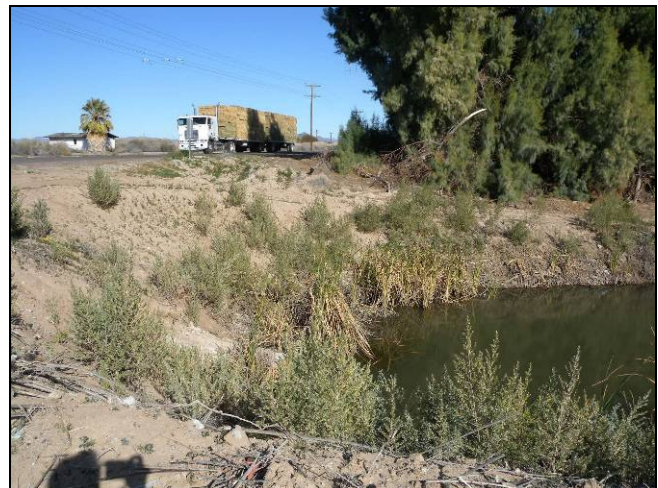
Figure 10: Drainage Ditch Just East of 4 th Avenue
