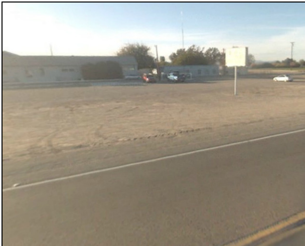
Figure 35: Undefined Access at Head Start
