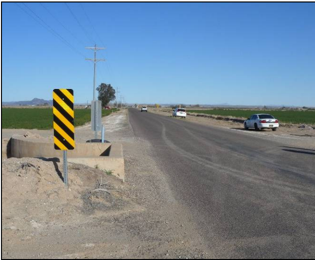
Figure 13: Object Markers East of 13 th Avenue Should Be Located at Edge of Headwall Closest to Road
