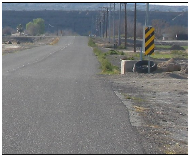
Figure 13: Object Markers East of 13 th Avenue Should Be Located at Edge of Headwall Closest to Road
