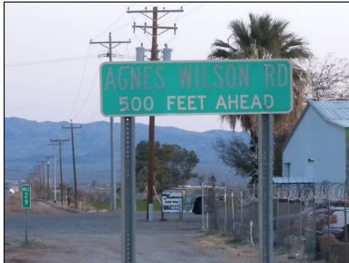
Figure 6: Advance Street Name Sign for Agnes Wilson Road
