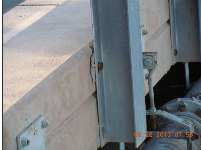
Figure 26 Continued: Damaged Guardrail at Canal Crossing near Patrick Road
