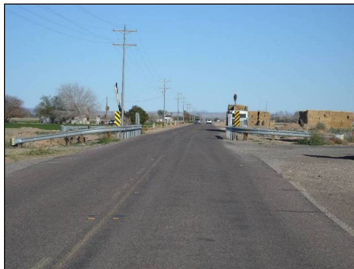
Figure 14: Narrow Bridge Near 12 th Avenue
