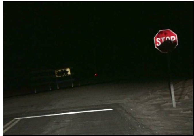
Figure 17: Graffiti on Stop Sign and Large Arrow Sign Diminish Visibility of the Signs
