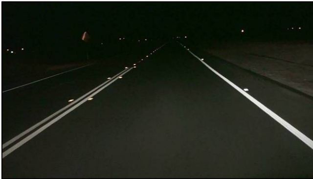
Figure 5: Sections of Burns Road With and Without Pavement Markings and RPMs
