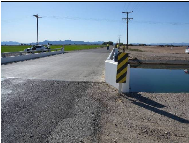
Figure 9: Burns Road Canal Crossing East of 4 th Avenue
