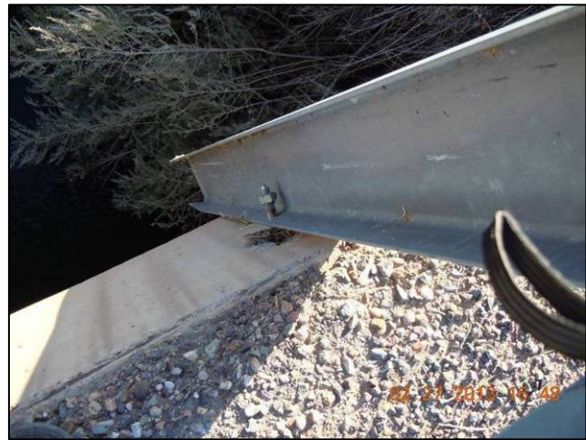
Figure 12: Inadequate Connections of Guardrail Posts to Concrete at 12 th Avenue Bridge
