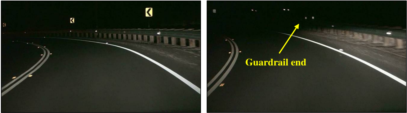
Figure 15: Curve at 2 nd Avenue and Agency Road. Note the Guardrail and Chevrons Do Not Extend Through the End of the Curve.
