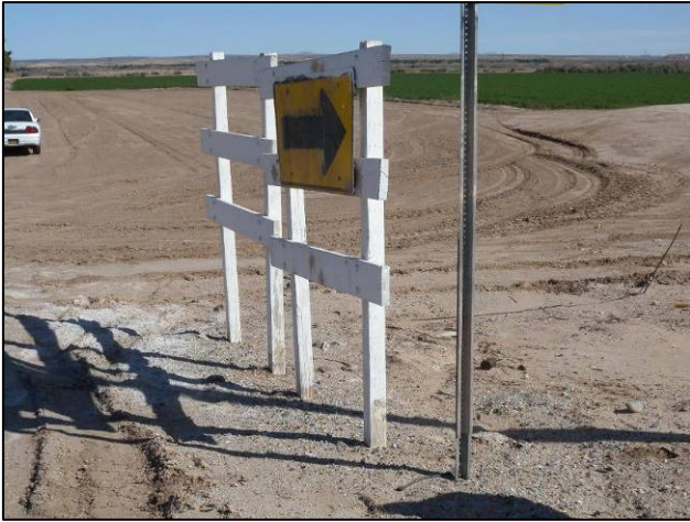
Figure 16: Wooden Barricades on Outside of Curve at 4 th Avenue and Indian School Road Create a Fixed Object Hazard
