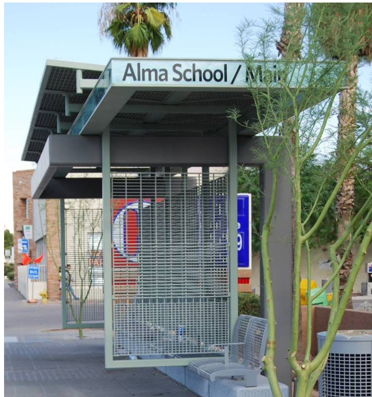
Figure 5 - Main Street LINK Station
