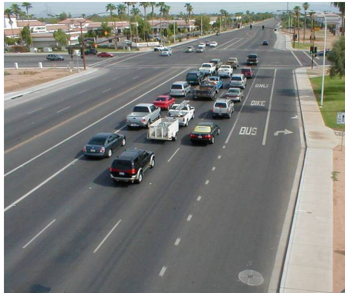
Figure 3 - Queue Jump, Transit Signal, and Far-side Bus Stop in City of Chandler
