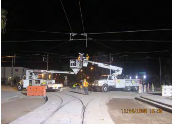
11 th Street Loop – Installing Headspans
