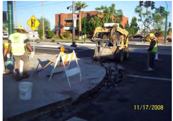
Punch List Curb and Gutter Replacement
