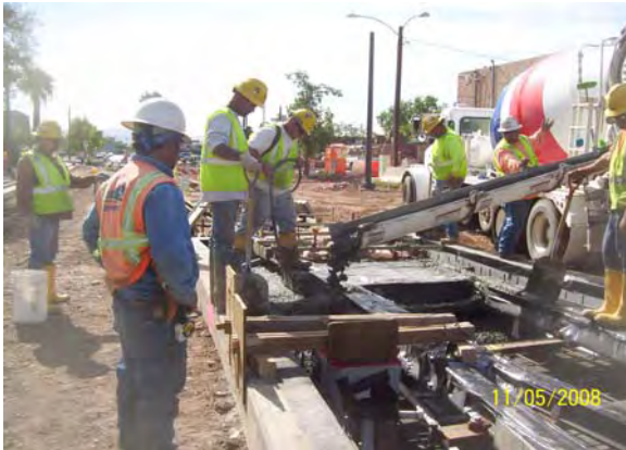
Concrete Placement at 11 th St. Loop Equilateral Bathtub
