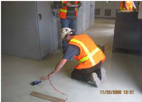
TPSS No. 10 – Dielectric Floor Testing
