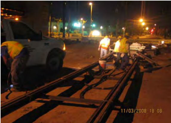
11th Street Loop Cable Installation
