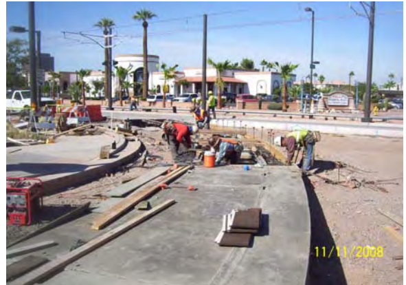
11th St. Loop Guideway Placement
