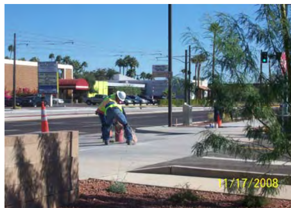
Cutting a Control Joint Central/Camelback Park and Ride Facility
