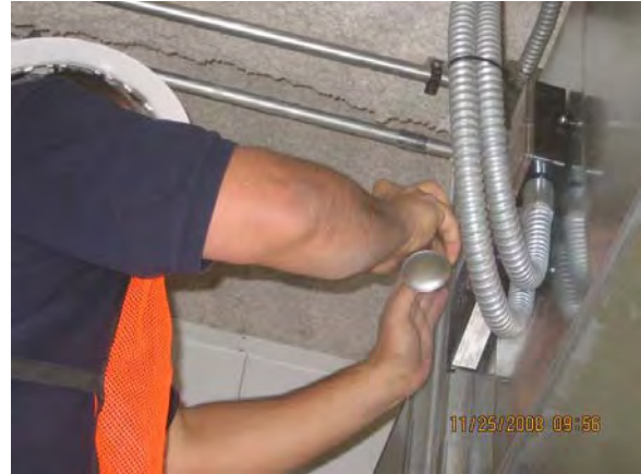
TPSS No. 2 – Duct Detector Testing
