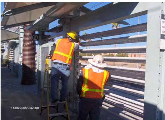
Ambient Noise Sensor Testing at Sycamore and Main Station
