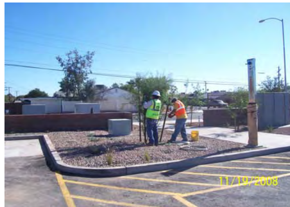
Staking Trees Sycamore/Main Park and Ride Facility
