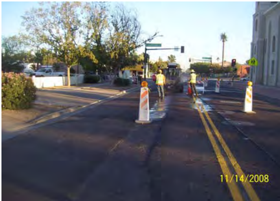
Punch List Pavement Repair at Trench
