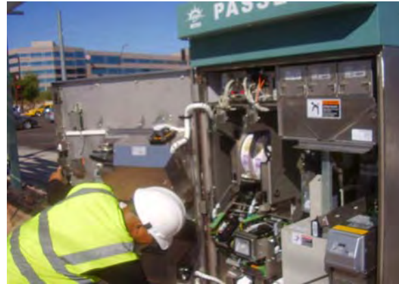
Acceptance Testing at Priest and Washington Station
