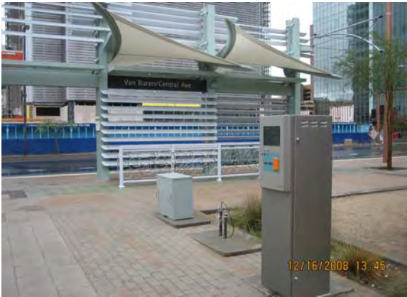
Standalone Smartcard Ticket Validator Installation at Central and Van Buren Station
