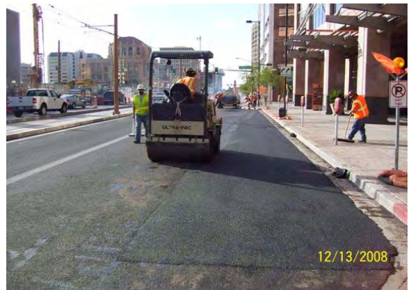
Rubberized AC Punch List Replacement
