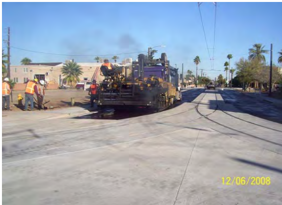
11 th Street Loop Rubberized AC Paving
