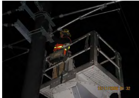
Installing Bonding Jumpers for Downguys
