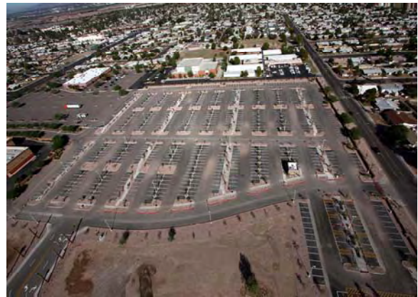
Parking Lot Overview Sycamore/Main Park-and-Ride Facility
