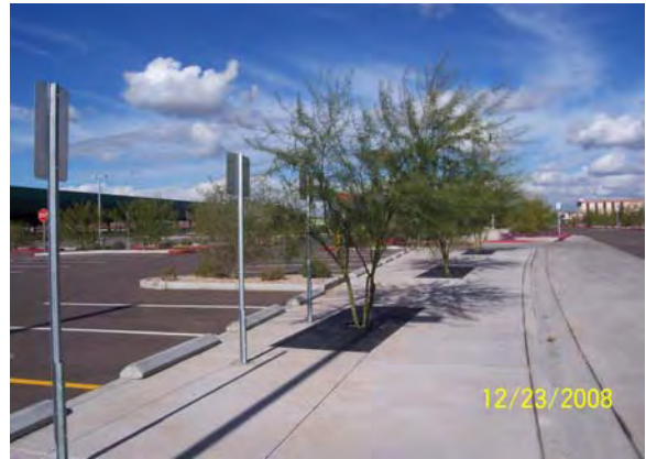
Completed Parking Lot 38 th Street/Washington Park-and-Ride Facility
