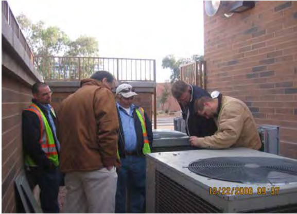
TPSS No. 10 – HVAC Troubleshooting
