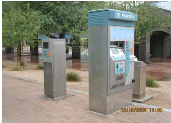
Standalone Smartcard Ticket Validator Installation at Central and Van Buren Station
