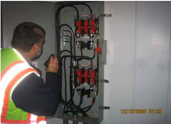
City of Phoenix Electrical Inspection at Signal Building No. 1
