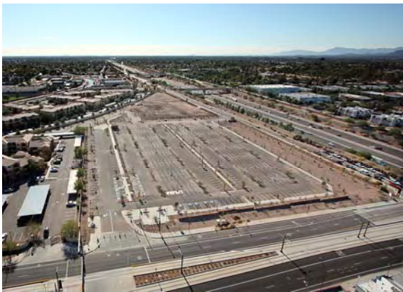
Parking Lot Overview Price/Apache Park-and-Ride Facility
