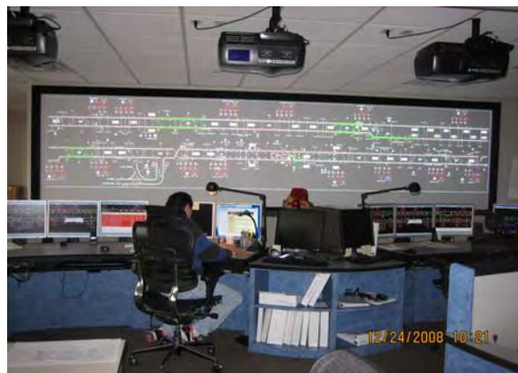
Final Adjustments at Operations Control Center in Preparation for Opening Day
