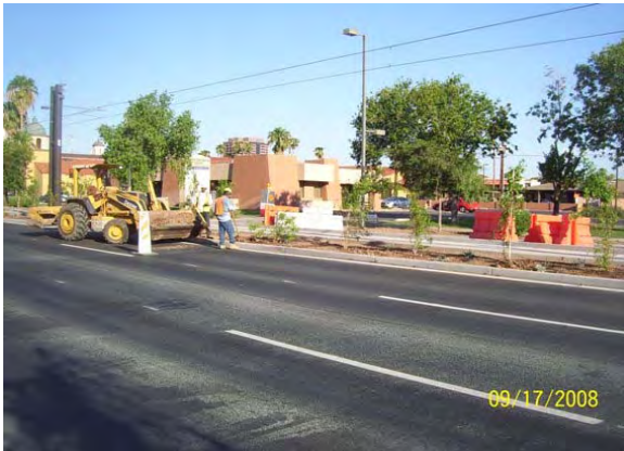
Landscape Planting and DG installations
