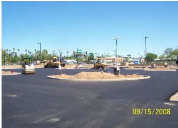
Paving West of 3 rd Avenue Central Ave/Camelback PNR Facility
