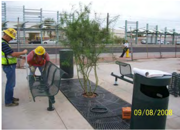
Site Furnishings Installation 19 th Avenue/Camelback PNR Facility
