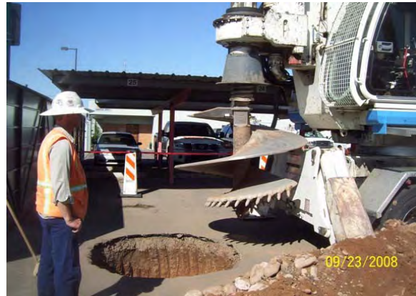
Dry Well Installation for Parking Lot Drainage
