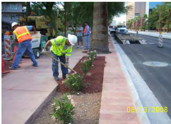
Placing Landscaping Decomposed Granite
