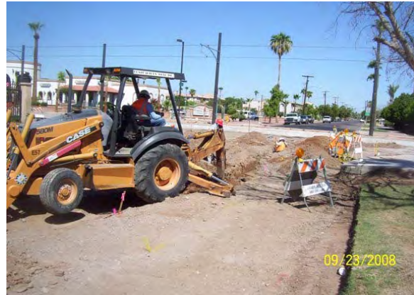
Combined Systems Duct Bank Installation for 11 th Street Loop
