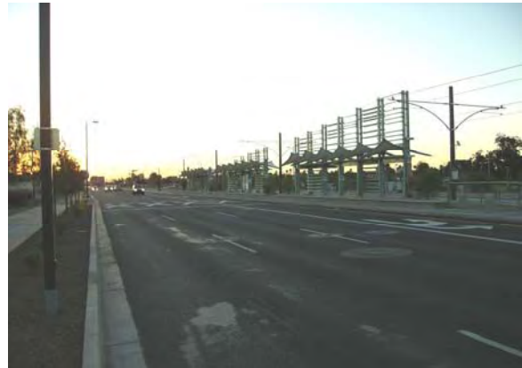
Completed Work on Camelback Avenue
