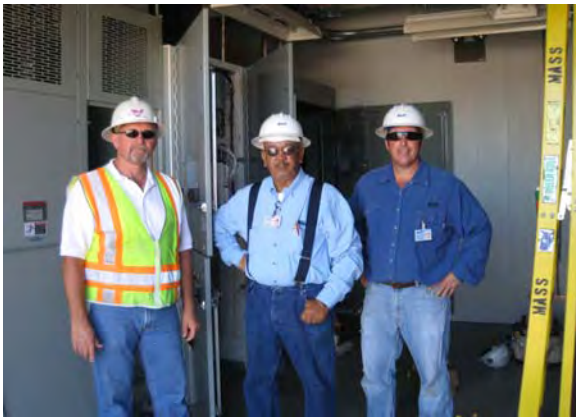
SRP onsite preparing TPSS No.1 to be energized
