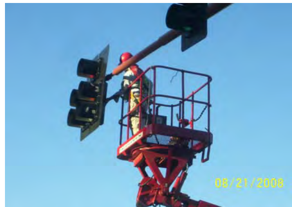
Adjusting Traffic Signal heads
