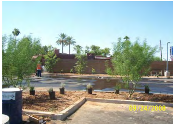
Landscaping Installation Central Ave/Camelback PNR Facility
