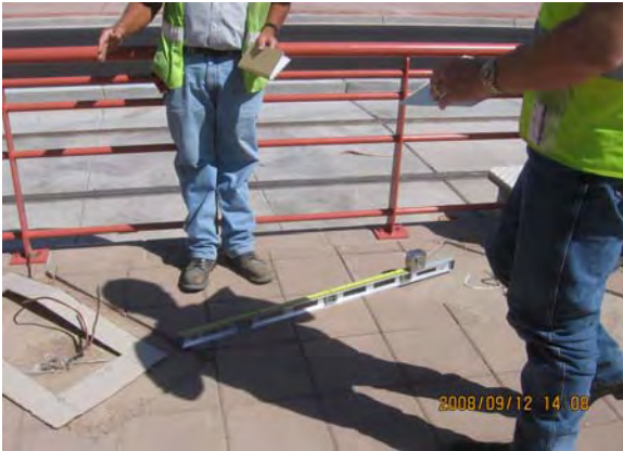
Station Inspection at Thomas and Central Station
