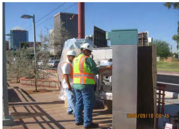
Testing In-Progress at Central and Indian School Station
