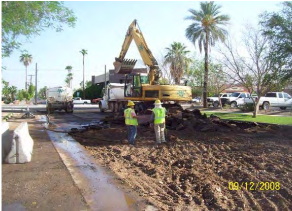
11 th Street Loop Roadway Demolition in progress
