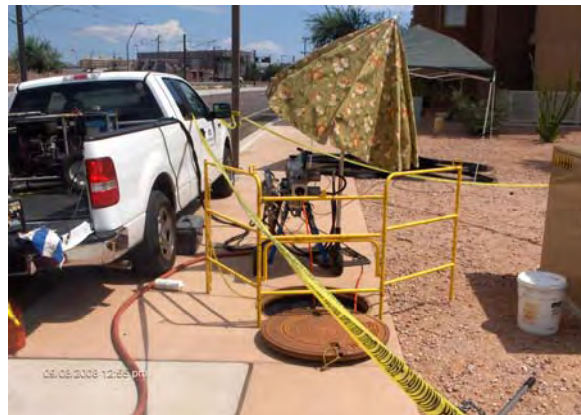
Installation of ASU Fiber Near Center Parkway
