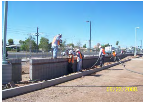
Screen Wall Construction 19 th Avenue/Montebello PNR Facility
