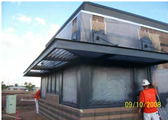
Painting Metal Work 19 th Avenue/Montebello PNR Facility
