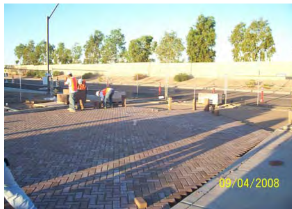
Brick Paver Installation Price Road/Apache Park and Ride
