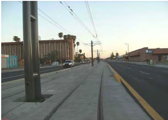
Completed Guideway on 19 th Avenue
