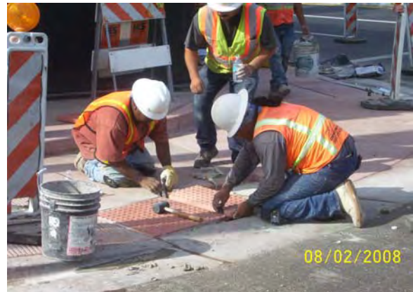
Replacing tactile pavers at sidewalk ramps
