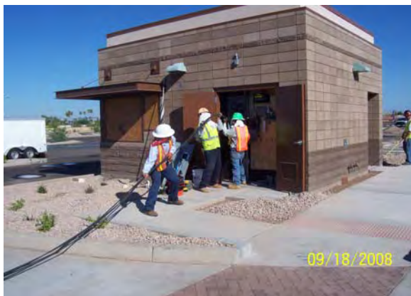
Pulling Wire for Electrical Service Price Road/Apache Park and Ride
