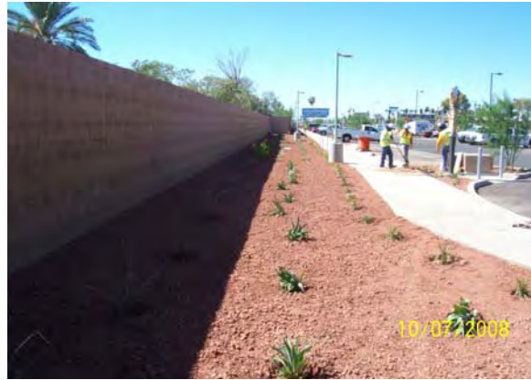
Final Cleanup Central/Camelback PNR Facility
