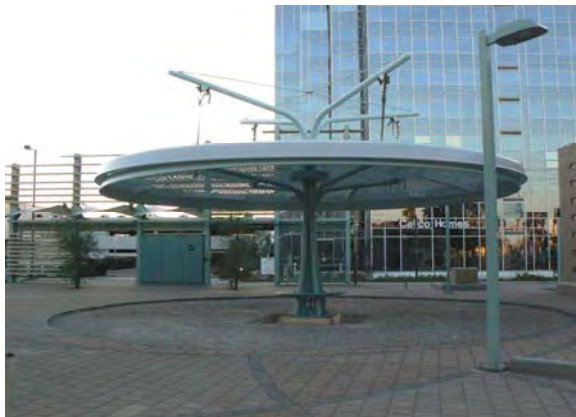
Central/Roosevelt Station Shade Canopy by Peter Richards
