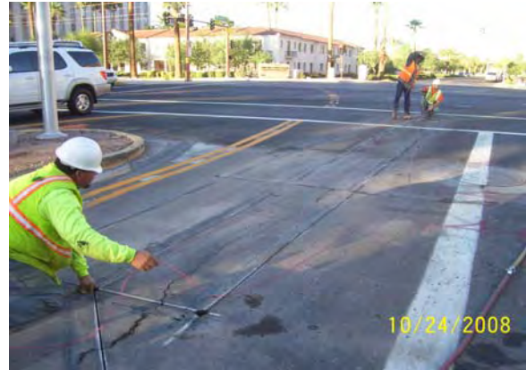
Replacing Traffic signal loop
