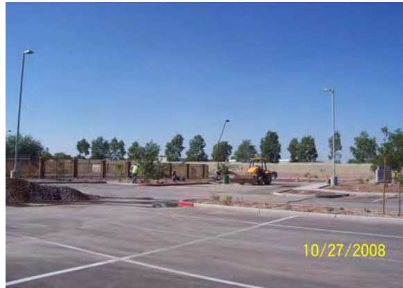
Placing Finishing Touches on Landscaping Price / Apache PNR Facility
