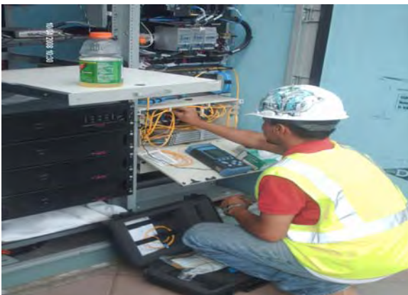
Street Traffic Fiber Testing between McDowell and Montebello
