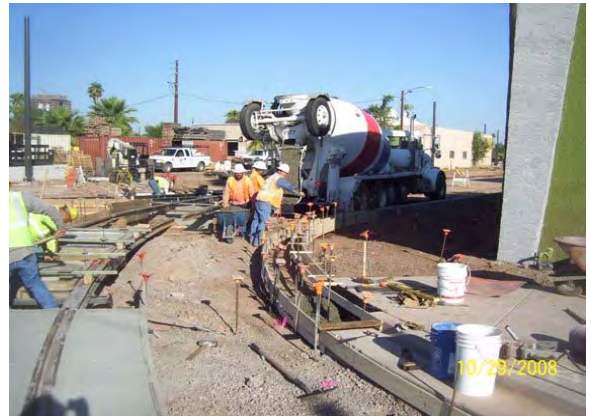
Curb and Gutter Placement for the 11th Street Loop
