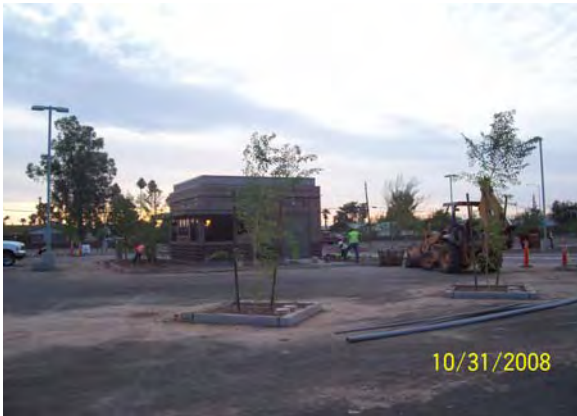
Landscaping Installation Sycamore / Main PNR Facility
