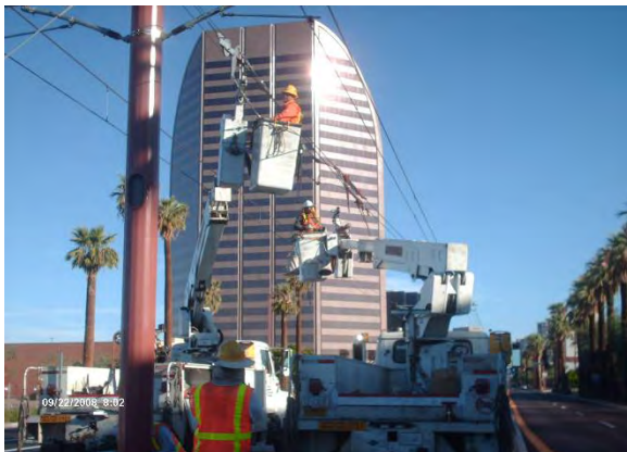
Line Section 2 – Balance Weight Adjustments
