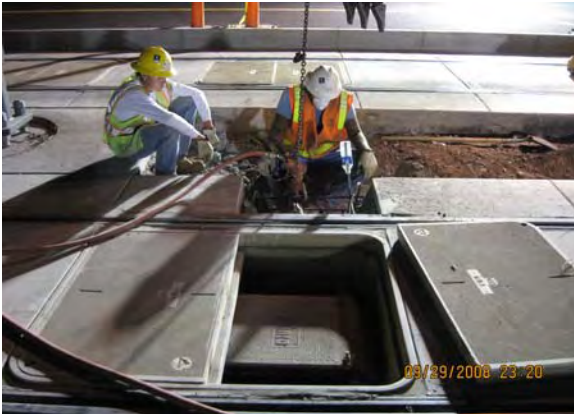
Demolition Work at Yard Entrance Interlocking
