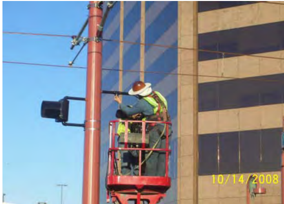
Installing Traffic signal
