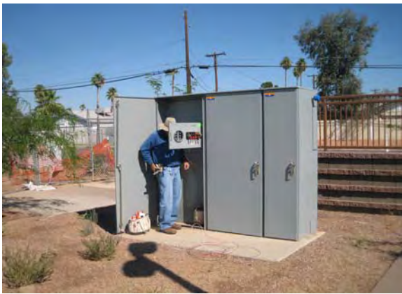
SRP onsite preparing Sycamore and Main Street for energizing
