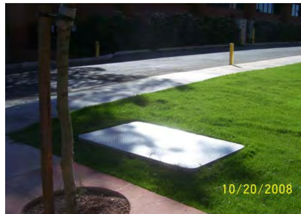
Replacing vault lid, Punch List item
