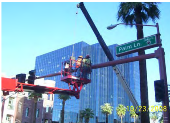
Replacing Mast arm
