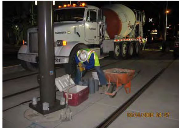
Concrete Testing at Yard Entrance Interlocking
