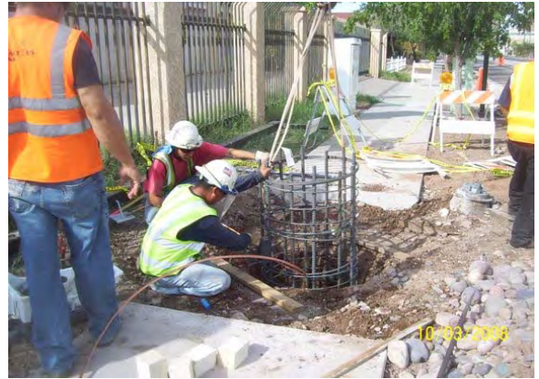
OCS Foundation Preparation for the 11th Street Loop
