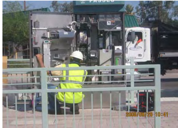
Testing In-Progress at McClintock and Apache Boulevard Station
