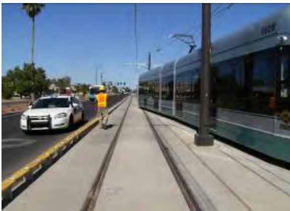
Test Train Going Through Switches on 19 th Avenue
