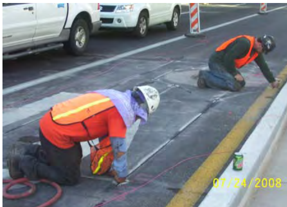
Installing Traffic Loops
