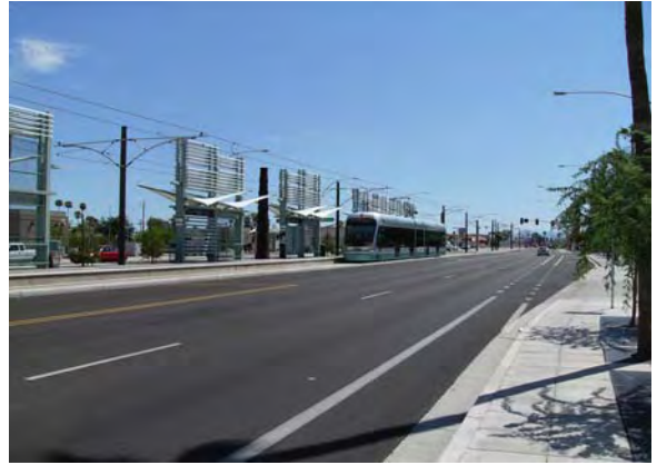
LRV at Sycamore Station
