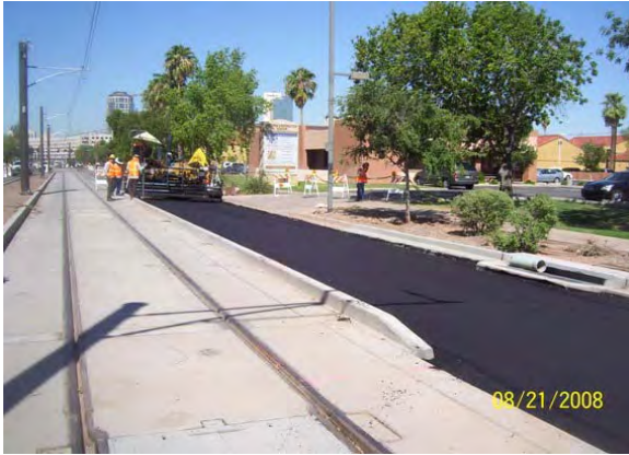
Leveling slip lane on Jefferson in between 11 th and 12 th Streets
