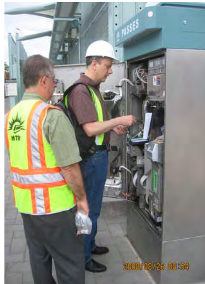
Pilot Testing In-Progress at 3 rd and Mill Station
