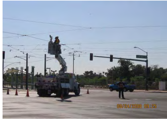
Line Section 1 – Installing Headspans at 19 th Ave. and Camelback Rd. Intersection
