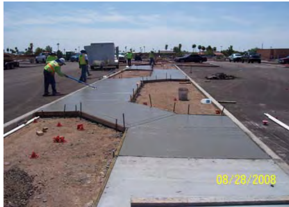
Placing Sidewalk in Median Islands Sycamore/Main Street Park and Ride
