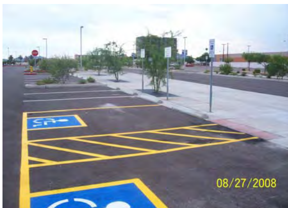
Finished Striping 38 th Street and Washington Facility
