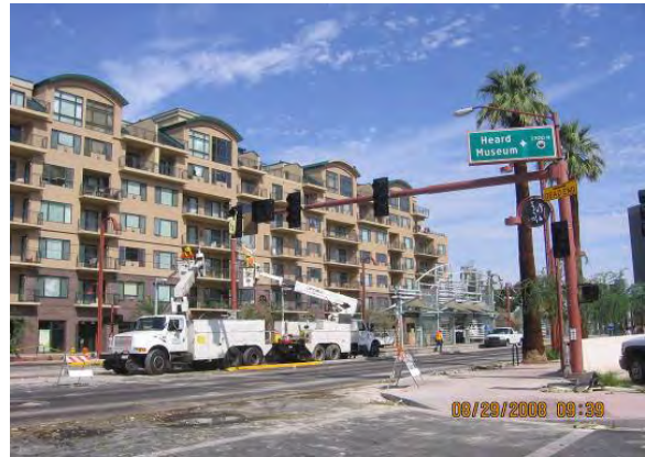
Line Section 3 – Repairing Damaged OCS at Encanto/Central Station
