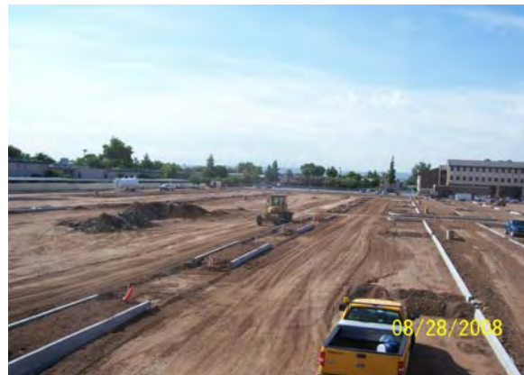
Subgrade Preparation 19 th Avenue/Montebello PNR Facility
