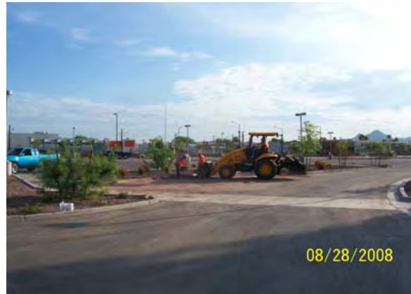
Landscape Installation 19 th Avenue/Camelback PNR Facility
