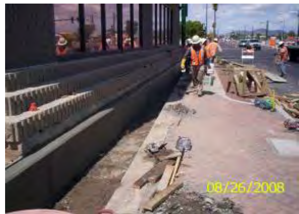
Property Transition Change Work on 19 th Avenue
