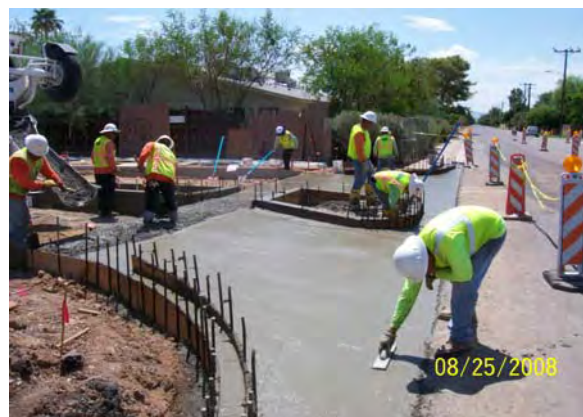
Placing Driveway East of 3 rd Ave. Central Ave/Camelback PNR Facility
