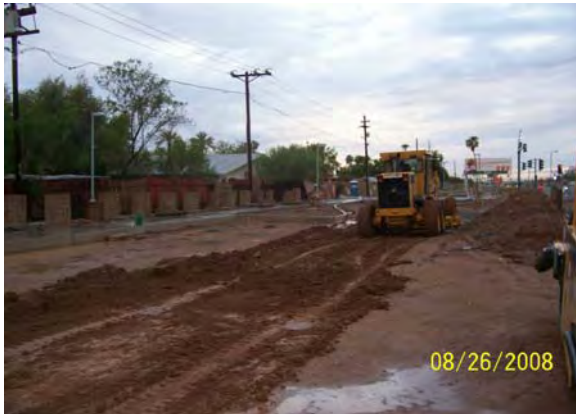
Grading East of 3 rd Ave. Central Ave/Camelback PNR Facility
