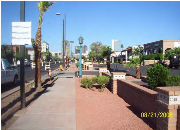
Landscape Planting and DG installations at 11 th Street and Washington
