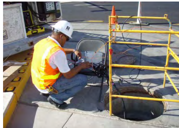
Fiber Splicing at 19th Avenue and Camelback Road
