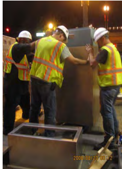
TVM Installation at 3 rd and Mill Station
