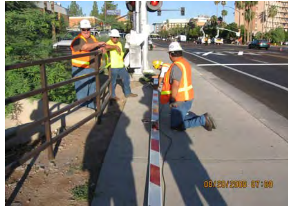
Gate Arm Installation at University Grade Crossing
