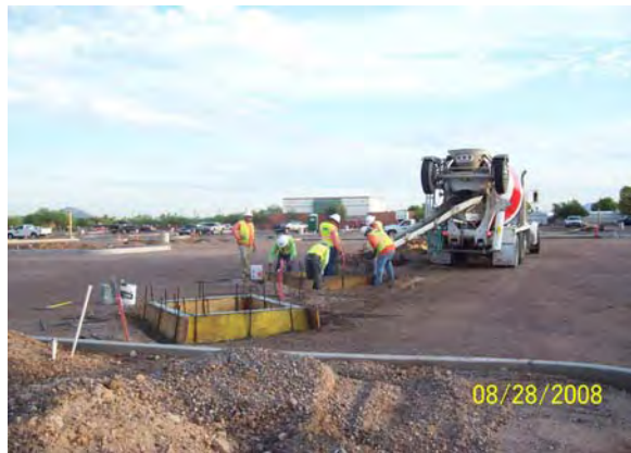
Placing Median Diamonds Sycamore/Main Street Park and Ride
