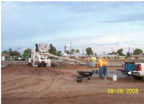
Placing Concrete for Bull Noses 19 th Avenue/Montebello PNR Facility
