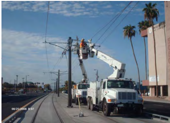
Line Section 1 – Messenger Wire Installed for Wire Runs 1 and 2
