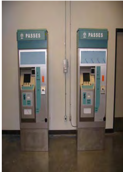
Workstation TVM Installation in Operations and Maintenance Center
