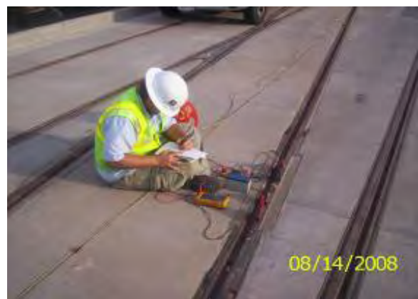
Rail to Earth Resistance Testing at 19 th Avenue
