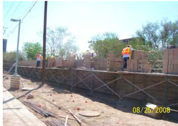
Placing Screen Walls Central Ave/Camelback PNR Facility
