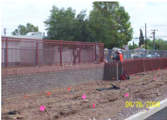
Installing View Fencing Sycamore/Main Street Park and Ride
