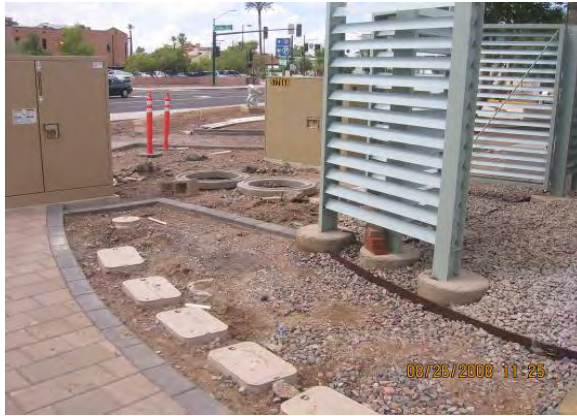
TPSS No. 5 – Metal Fence Louvers Installed
