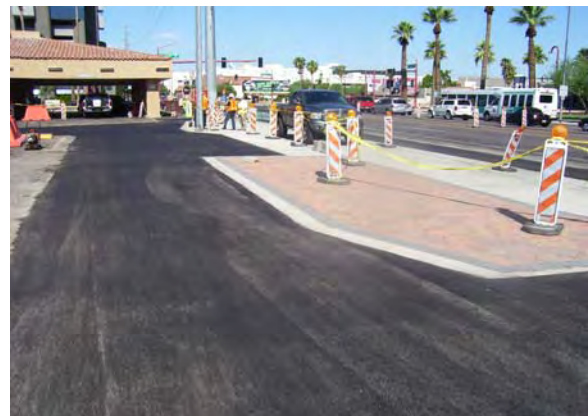
Installed Bus Stop on Thomas and new AC Pavement
