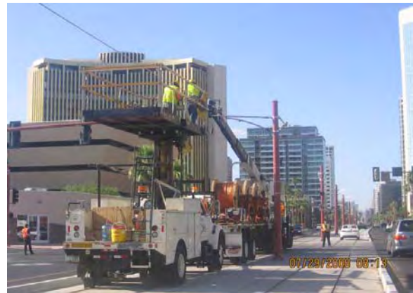
Line Section 2 – Installing Messenger Wire (WR 9)
