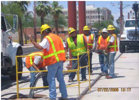
TPSS No. 3 – Installing Feeder Cable
