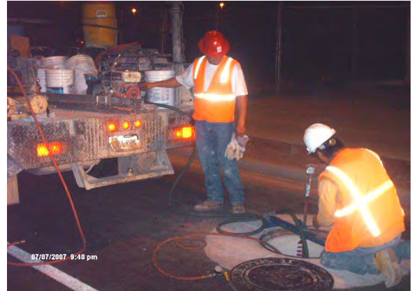
Manhole Testing on 19 th Avenue
