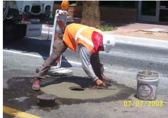
Raising Valves in new AC Pavement
