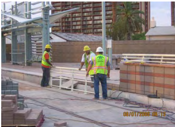
Central Avenue / Camelback Station Handrail Installation
