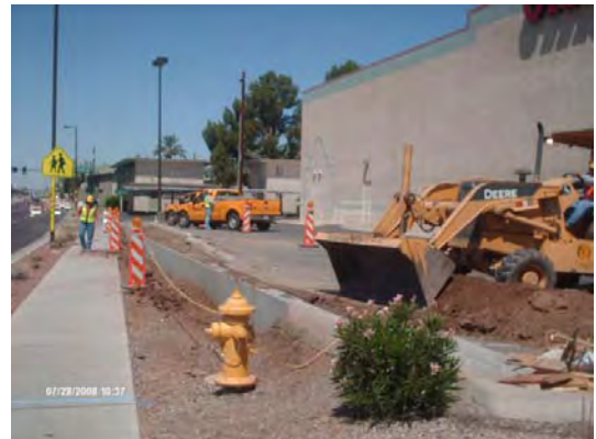
Back of Sidewalk Grade Transition at Office Max
