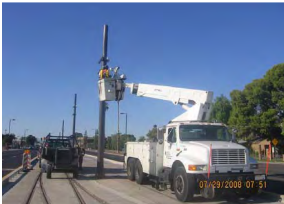
Line Section 1 – Installing OCS Hardware
