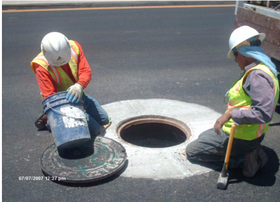
Adjusting manholes after Rubber Asphalt Paving
