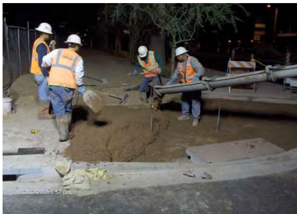
Replacing Sidewalk ramps
