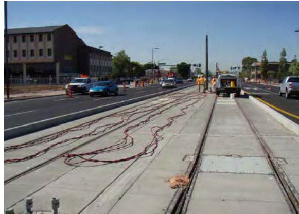
Installing Track Circuit Cable at Montebello Interlocking
