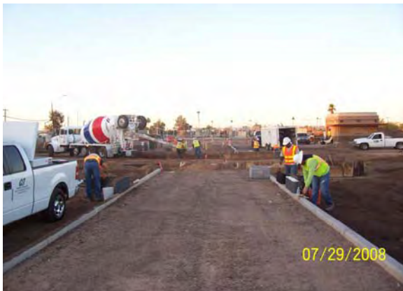
Curb Installation – Sycamore and Main
