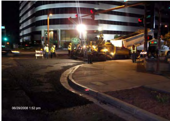
Laying Rubberized Asphalt at Camelback
