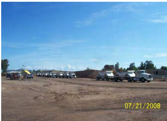
Mass Excavation - Montebello and 19 th Avenue
