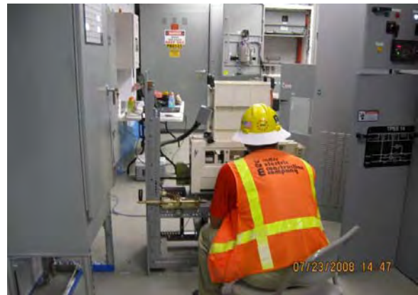
TPSS No. 14 – Testing and Commissioning
