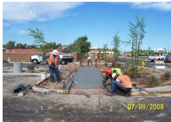
Sidewalk - Camelback and 19 th Avenue
