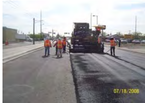
Leveling on Jefferson just West of 18th Street
