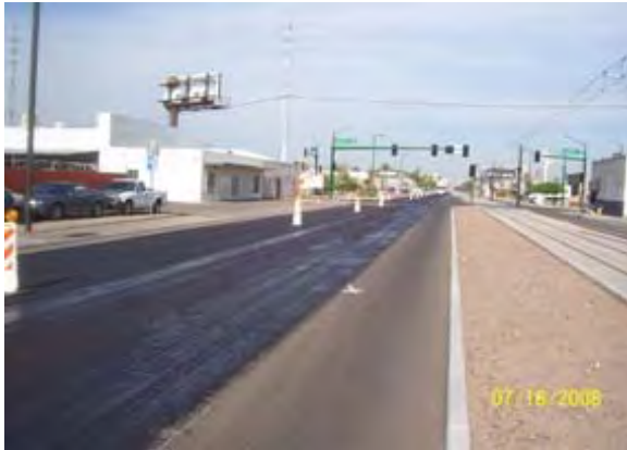
Milling operations at 18th Street and Jefferson
