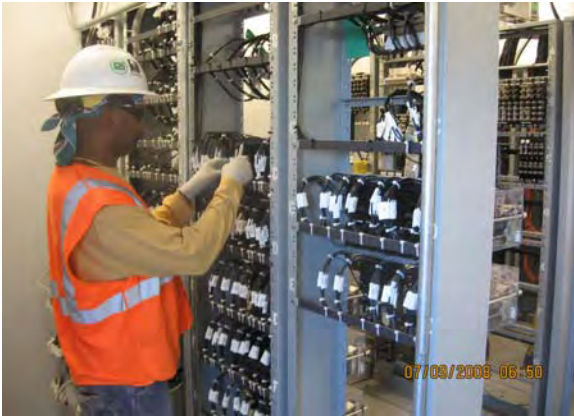
Static Testing at Pierson Interlocking Signal Building
