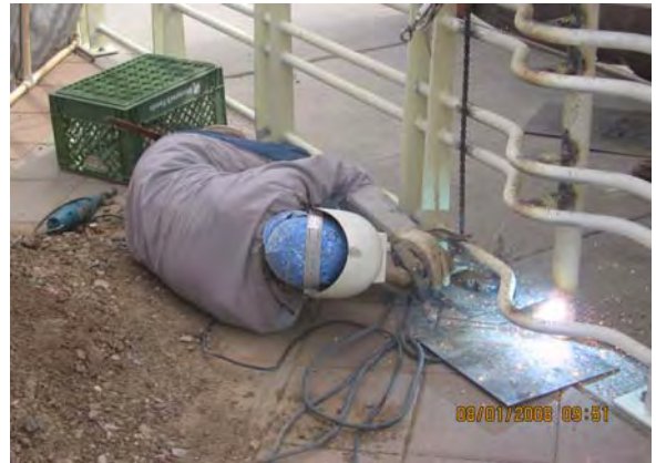
McDowell / Central Avenue Station Handrail Installation
