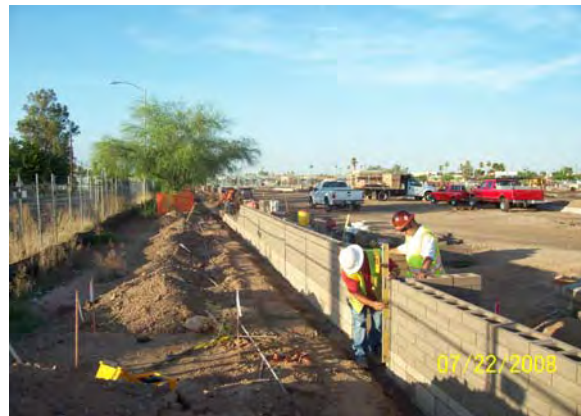
Screen Wall Construction – Sycamore and Main
