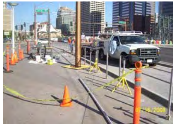
Hand Rail Installation at the US Airways Center
