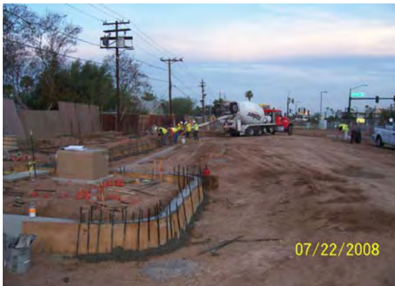
Curb Placement - Central and Camelback
