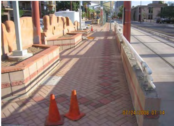
Encanto / Central Station Artwork, Handrail, and Pavers
