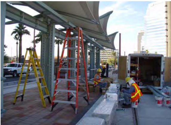
Installing Variable Message Boards at Central and Thomas Station
