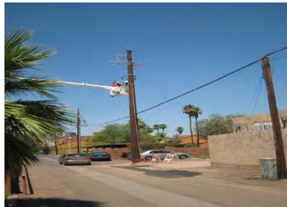
11 th Street Turn – Around – APS overhead to underground conversion
