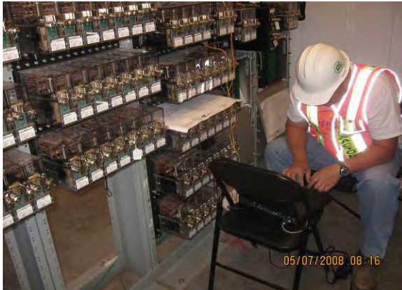
Performing Signal Acceptance Testing at Mill Pocket Interlocking
