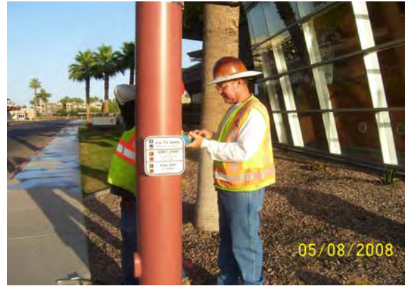
Traffic Signal installation
