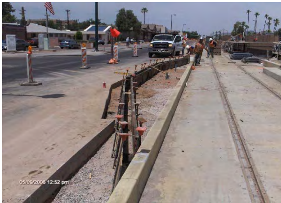
Forms for curb for Traffic Type A poles
