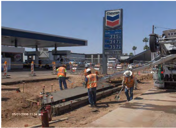
Placing driveway in front of Chevron gas station
