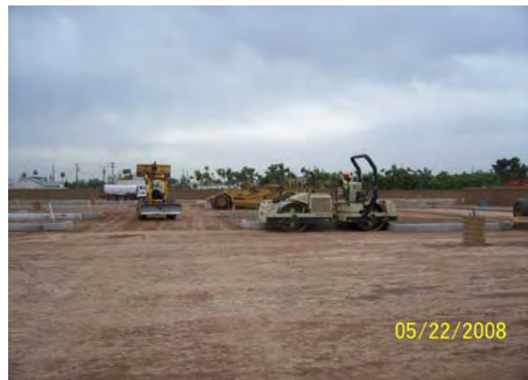
Subgrade Preparation Camelback and 19 th Avenue
