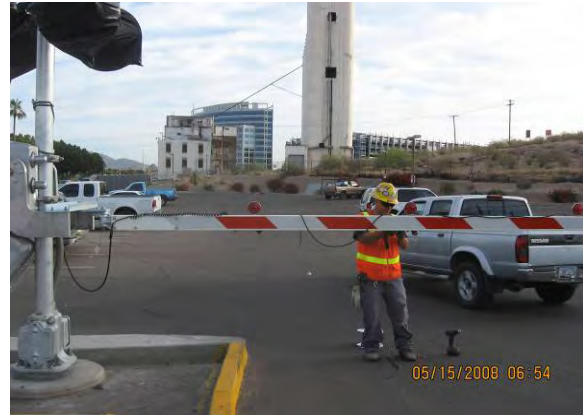
Testing Gate Crossing Mechanisms at Mission Palms Crossing
