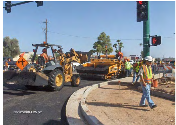
Paving at Montebello and 19 th Avenue
