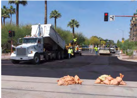
AC Paving at Palm Lane
