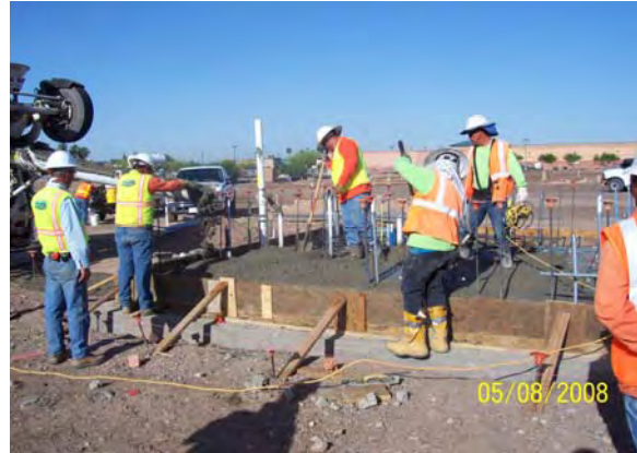
Security Building Slab – Sycamore and Main
