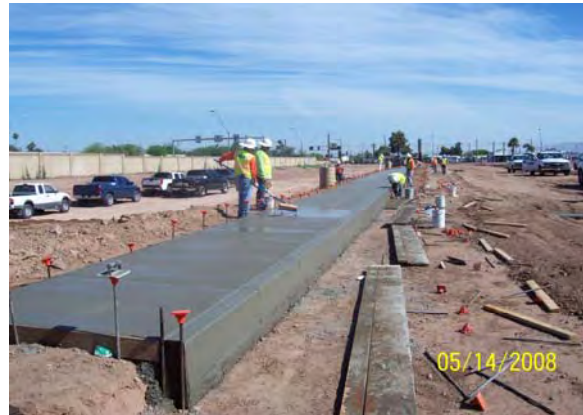
Sidewalk Installation - Price and Apache
