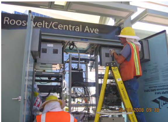
Terminating Communication Cable at Roosevelt/Central Station
