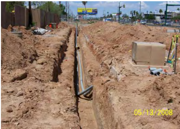
APS Conduit Relocation - Central and Camelback
