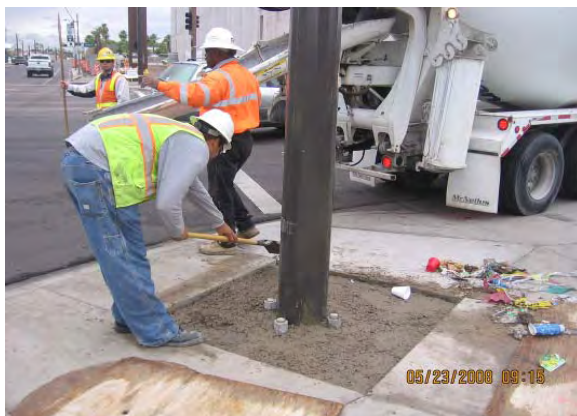
Line Section 5 – Restoring OCS Pole Foundations
