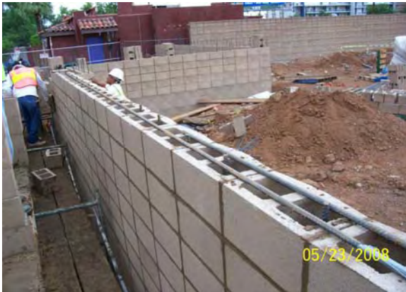
Retaining Wall Installation - Central and Camelback
