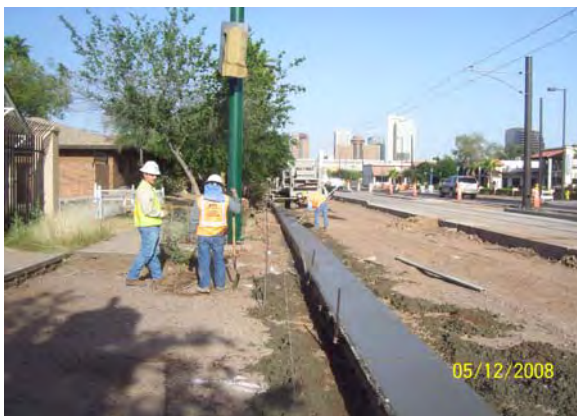
Preparing frontage road subgrade on Washington
