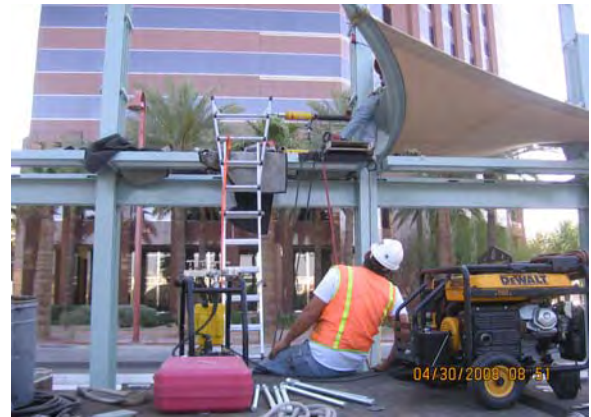
Thomas/Central Avenue Station Canopy Installation
