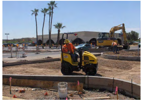
Preparing grade for paving
