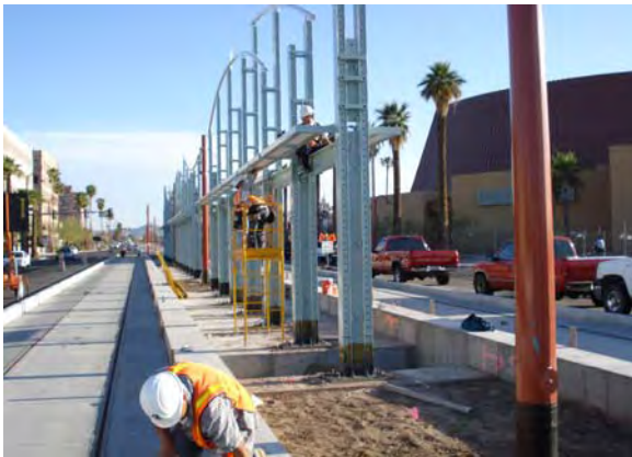
Campbell/Central Avenue Station Electrical Installation
