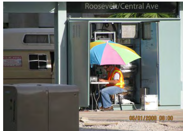
Performing Backbone Fiber Splices at Roosevelt/Central Station
