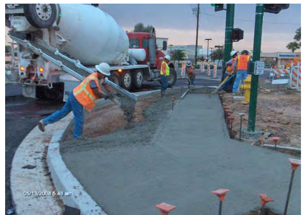
Placing concrete for pedestrian ramps & sidewalk
