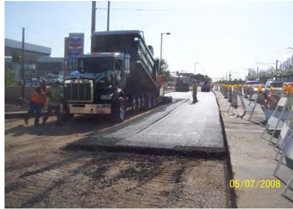
Placing asphalt base at Washington and 24 th Street
