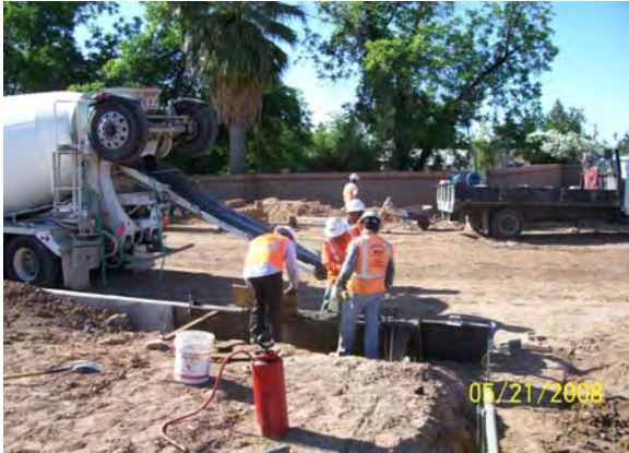
Curb Installation - Camelback and 19 th Avenue
