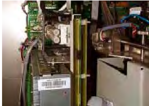
Witnessing Cable Retrofits as a result of Electro Magnetic Interfere Testing
