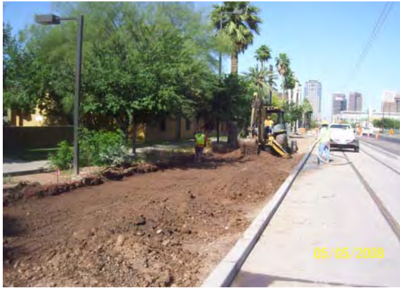
Frontage road subgrade preparation on Washington
