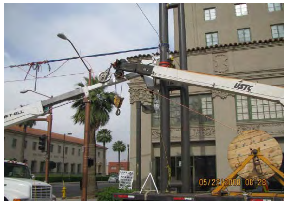
Line Section 3 – Stringing Contact Wire for Wire Run 19
