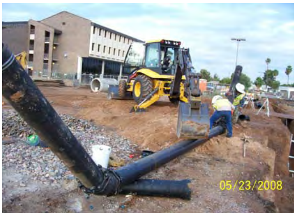
Fire Line Installation Montebello and 19 th Avenue
