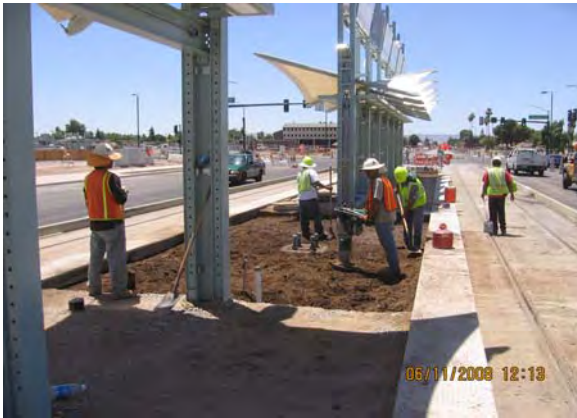
19 th Avenue / Montebello Station Construction
