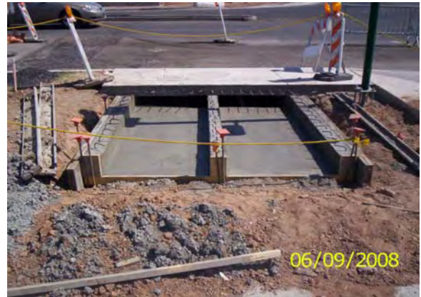
Placing concrete scupper on Montebello Avenue
