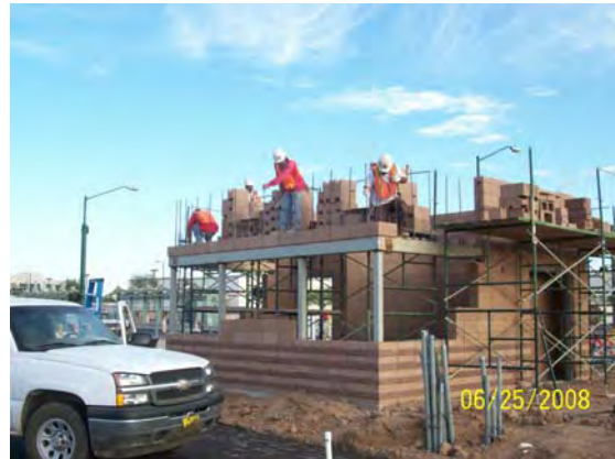
Security Building – Camelback and 19 th Avenue
