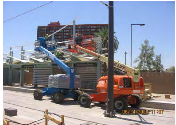
Louver Installation at Central / Camelback Station
