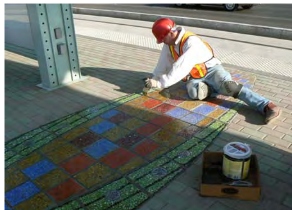
Benson Shaw installing pavers at McClintock
