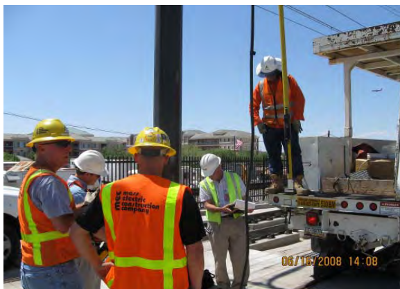
Electromagnetic Interference Tests over Town Lake Bridge
