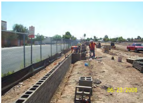
Screen Wall Installation - Sycamore and Main
