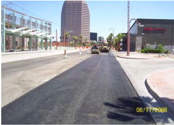
Placing asphalt paving on Central Avenue
