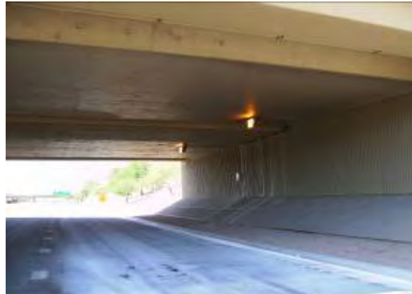
Completed Underdeck Lighting Replacement for ADOT at the Apache/Loop 101 Bridge
