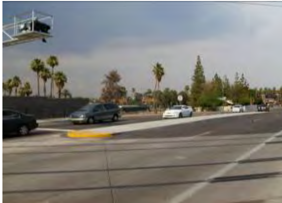
Completed Extra Work at University Crossing, Milestone H
