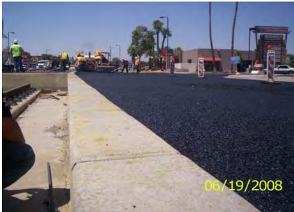
Placing final rubberized AC on 19 th Avenue
