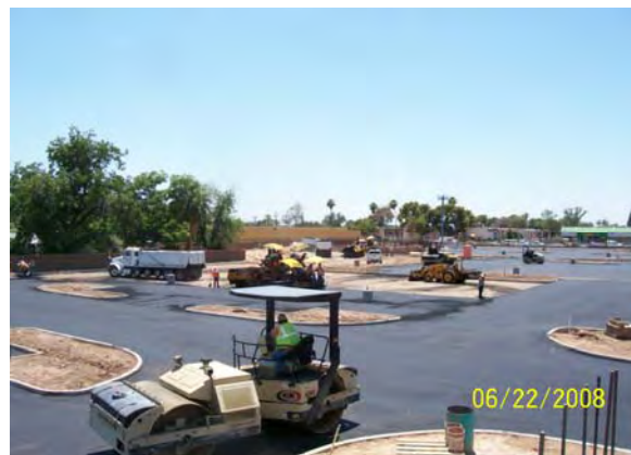
Paving - Camelback and 19 th Avenue
