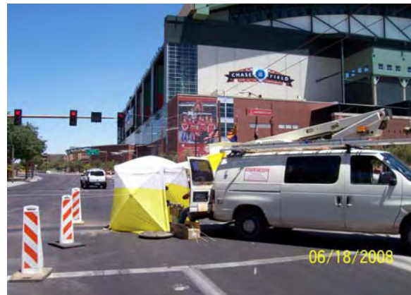
Street Traffic Fiber Optic Cable Splicing at 4 th Street
