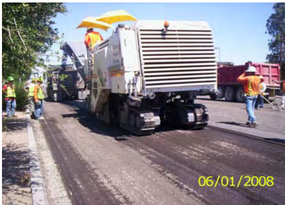
Grinding AC prior to final paving
