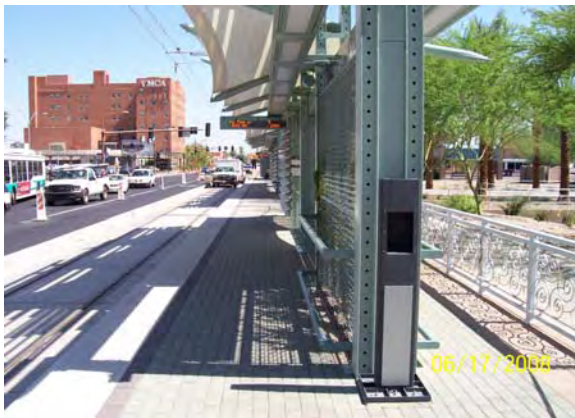
Communications System Testing at Van Buren and 1 st Avenue Station
