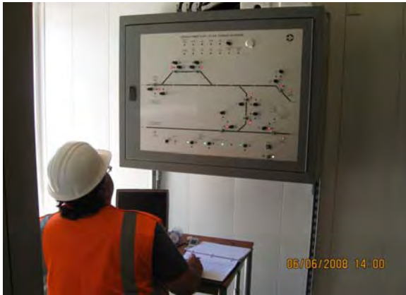
Performing Signal Acceptance Testing at McKinley Loop Interlocking
