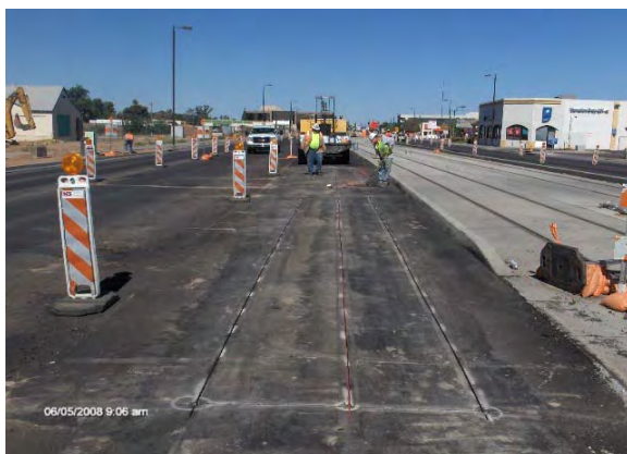
Installing Traffic loops on 19 th Avenue
