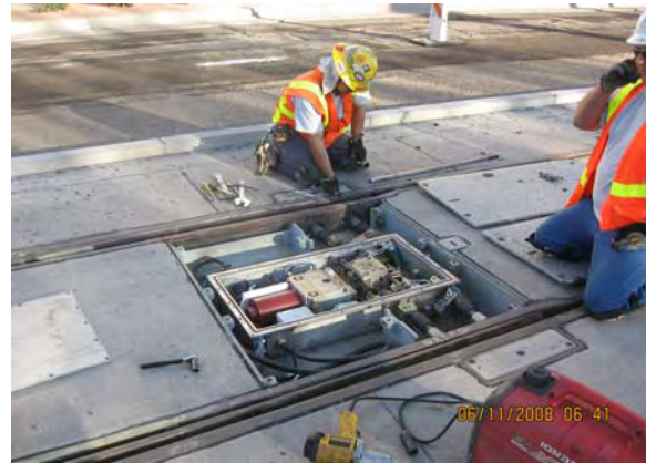
Final Switch Machine Adjustments at Culver Interlocking
