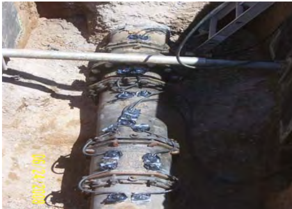
Installing Cathodic Protection on 12" DIP
