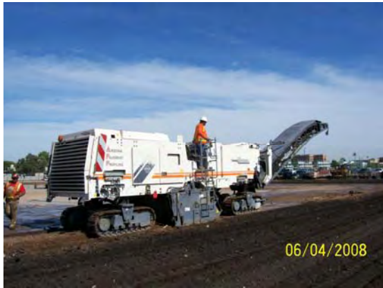
Asphalt Pulverization - Montebello and 19 th Avenue
