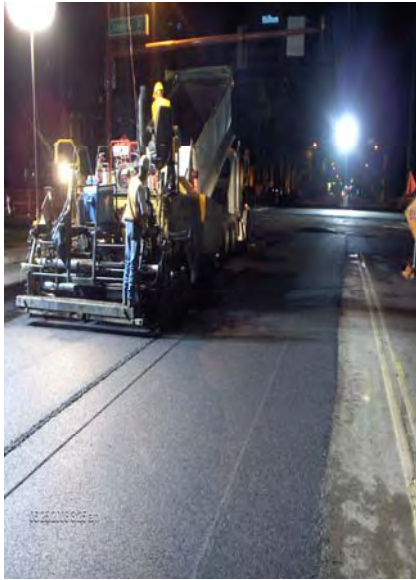
Laying Rubberized Asphalt at Thomas
