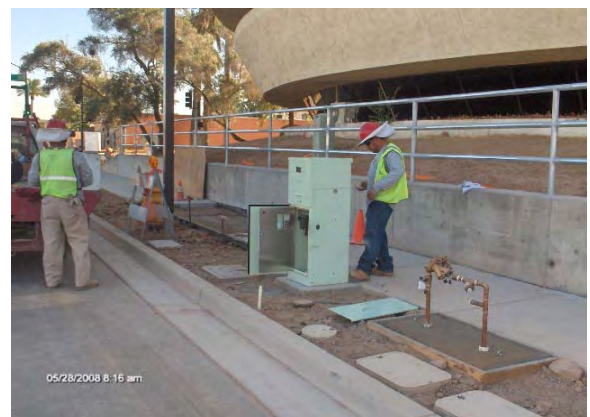
Installing meter box for irrigation controllers
