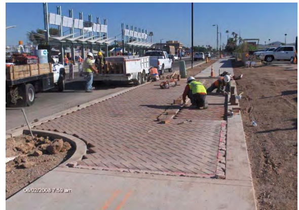
Placing pavers for bus stop on 19 th Avenue
