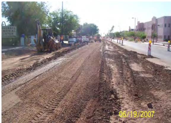
Preparing frontage road subgrade on Washington
