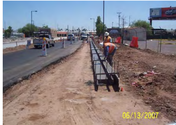
Placing curb and gutter on Jefferson
