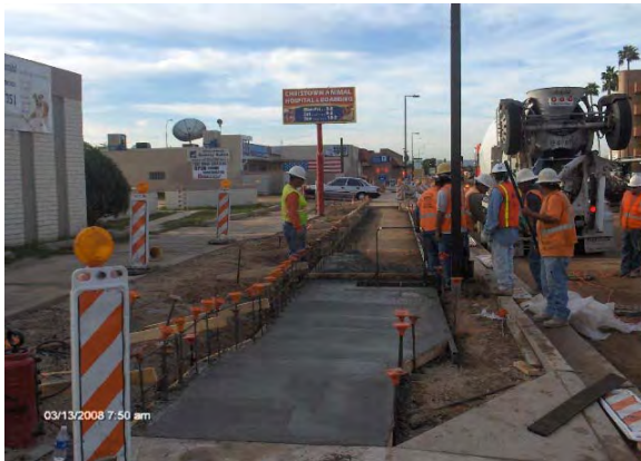
Placing Concrete for sidewalk
