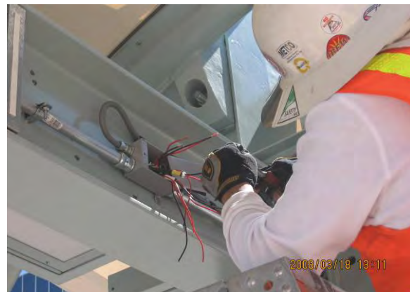
Terminating Speaker Cables at Roosevelt/Central Station
