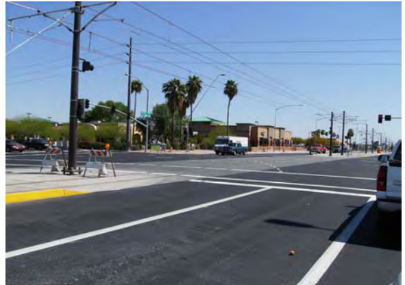
Completed Pavement Work, Mesa, Milestone H
