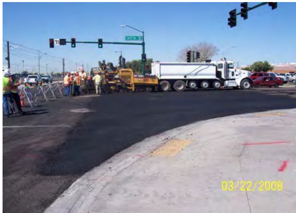
Rubberized AC Paving Punch-List Work at 40 th Street
