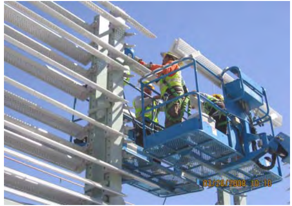
Louver Installation at Smith Martin/Apache Station
