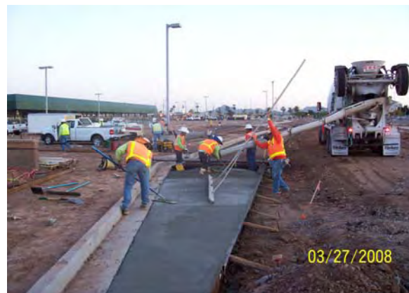
Concrete Paving for Bus Bay 38 th and Washington
