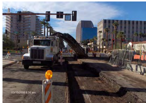
Milling roadway for widening
