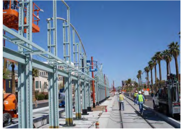
Installation of Structural Steel Accents at Central Avenue / Campbell
