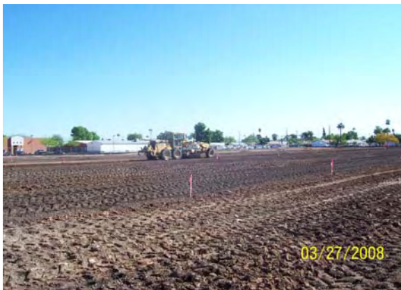
Subgrade Preparation Sycamore and Main
