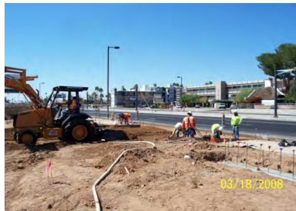
Driveway Construction Central and Camelback
