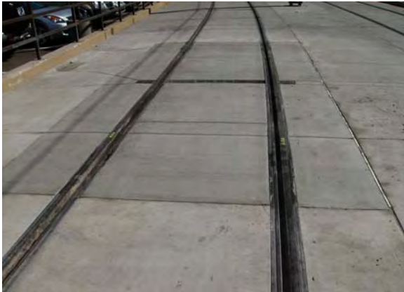
Completed Rail Repair, Milestone A
