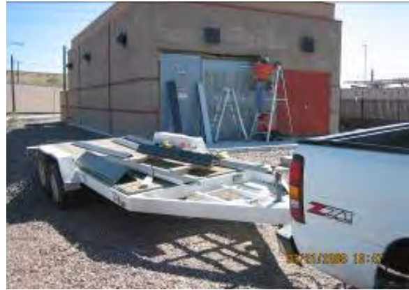
TPSS No. 15 – Installing AC Switchgear Opening Enclosure
