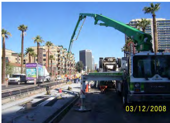
Placing Guideway South of Encanto Intersection
