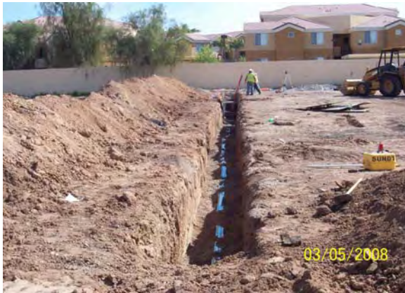
Water Line Installation Price and Apache
