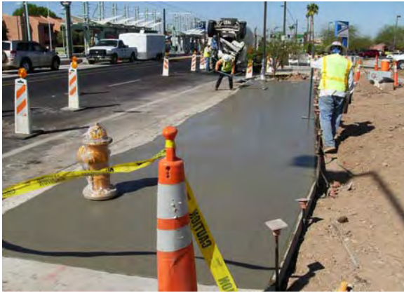
Change Work for COT, Milestone H
