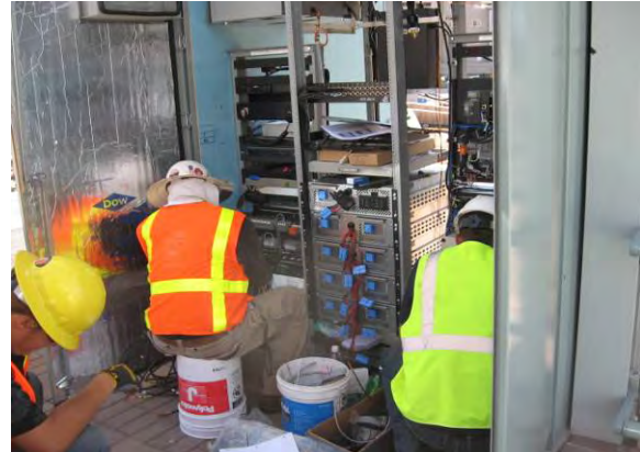
Terminating Communications Cable to Equipment at 5th/College Station
