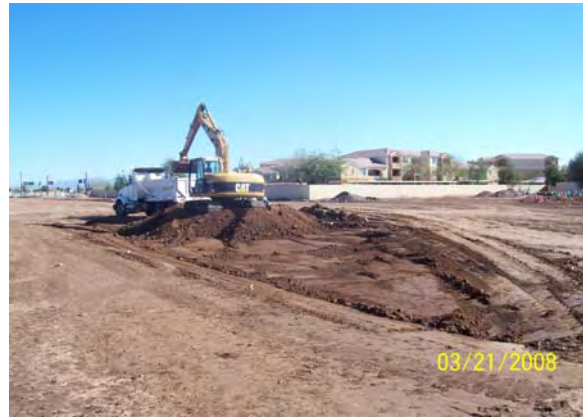
Retention Basin Excavation Price and Apache
