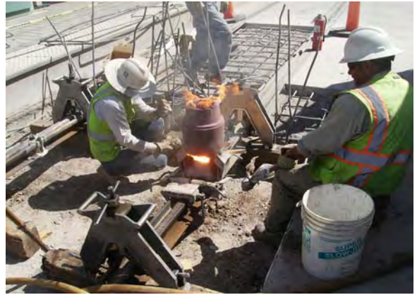
Rail Repair Work, Milestone A
