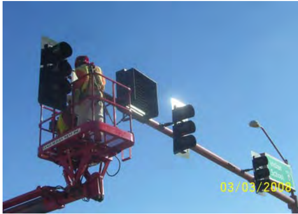
Installing Traffic Signals at Indian School
