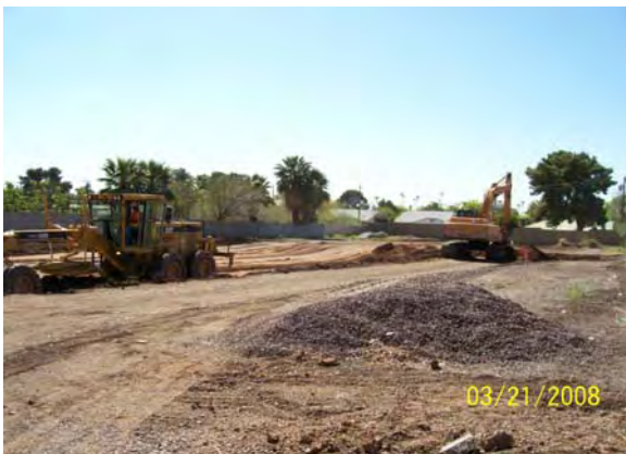
Subgrade Preparation Camelback and 19 th Avenue
