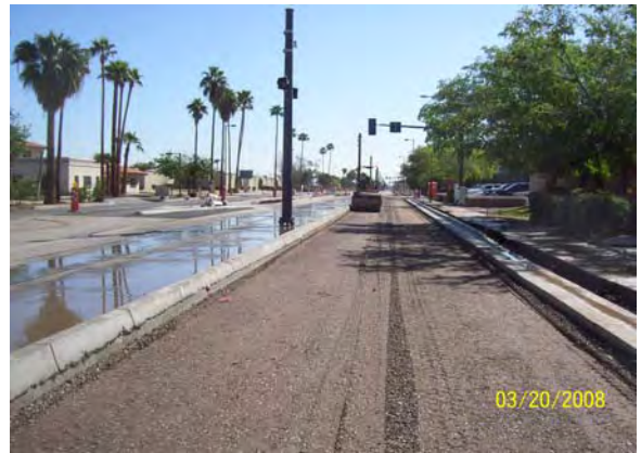
Frontage road subgrade preparation on Washington
