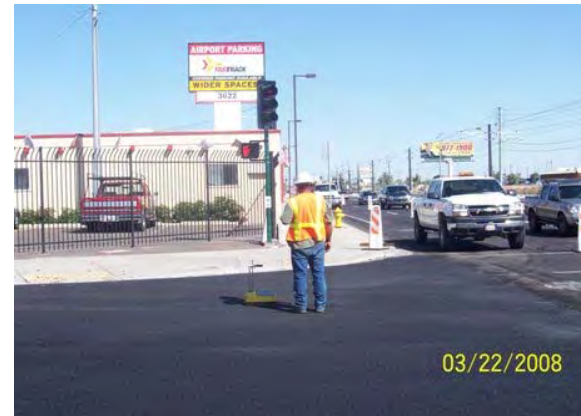
Density Test for the Rubberized AC Paving Punch-List Work
