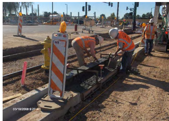
Placing concrete for Guideway curb
