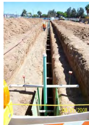
Sanitary Sewer Installation Montebello and 19 th Avenue
