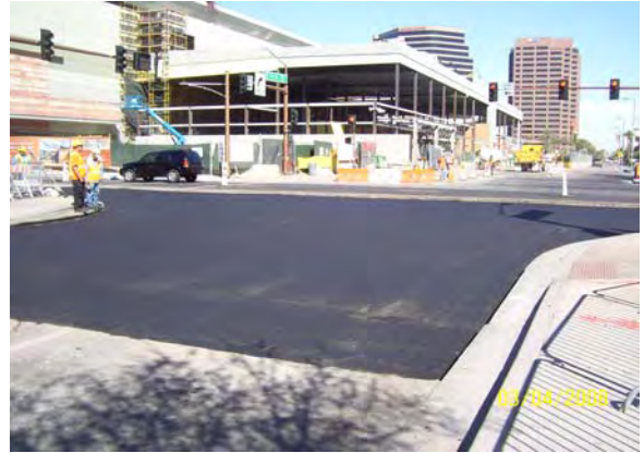
Base asphalt replacement at Washington and 5 th Street
