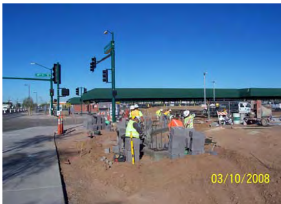
Monument Wall Installation 38 th and Washington
