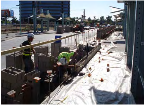
Planter Wall Construction at Central Avenue/Camelback Station
