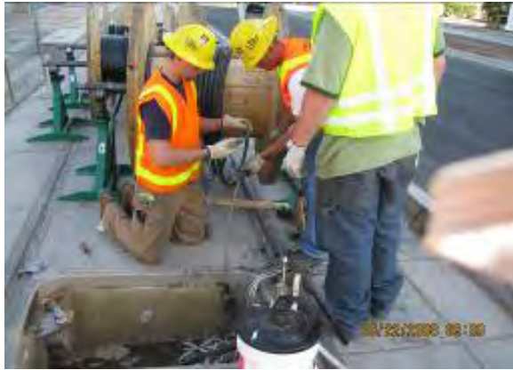
TPSS No. 5 – Pulling Feeder Cable
