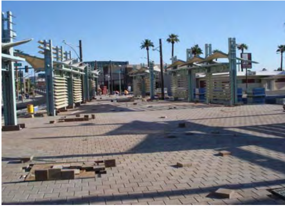
Paver Installation at Roosevelt / Central Station
