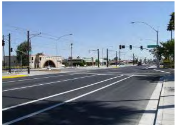
Completed Work at Sycamore Street, Milestone H
