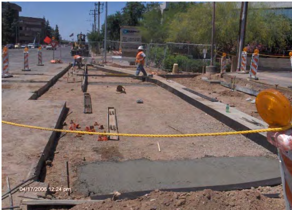
Forming up the Bus Bay at 19 th and Camelback Road
