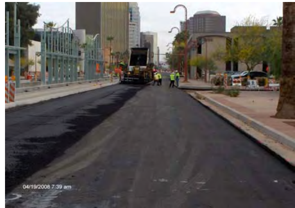
AC Paving North Bound
