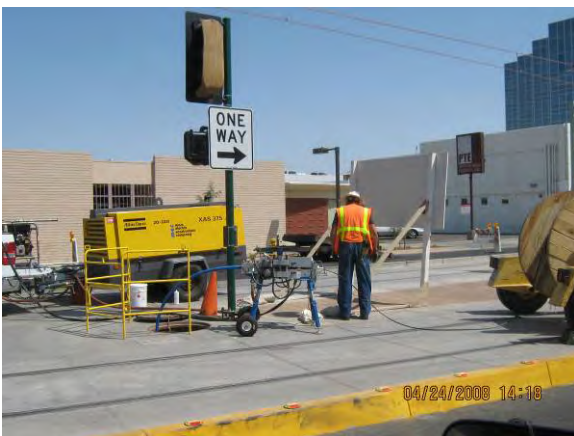
Blowing Fiber at Line Section 3
