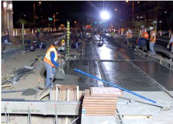
Placing Guideway
