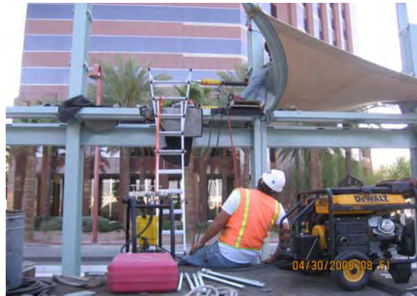
Thomas/Central Avenue Station Canopy Installation
