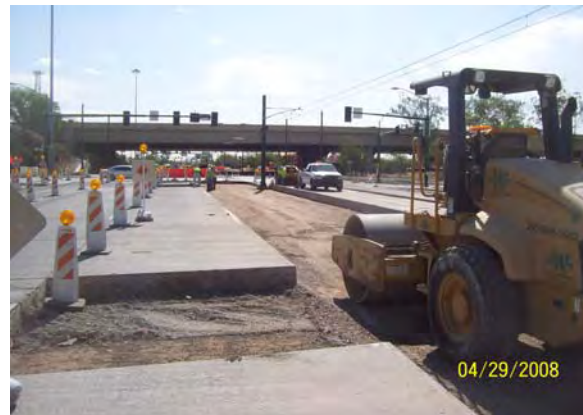
Placing concrete paving at I-10
