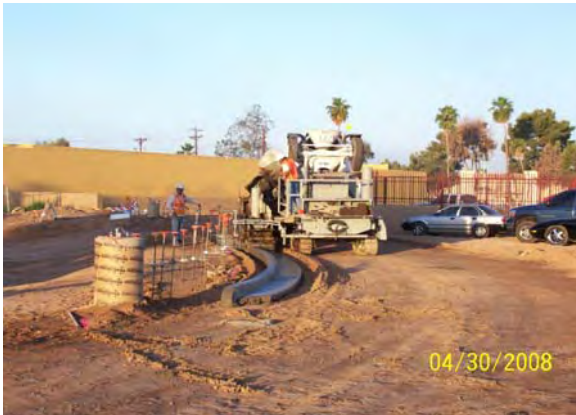
Curb and Gutter Installation Camelback and 19 th Avenue
