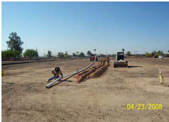
Irrigation Sleeve Installation - Sycamore and Main
