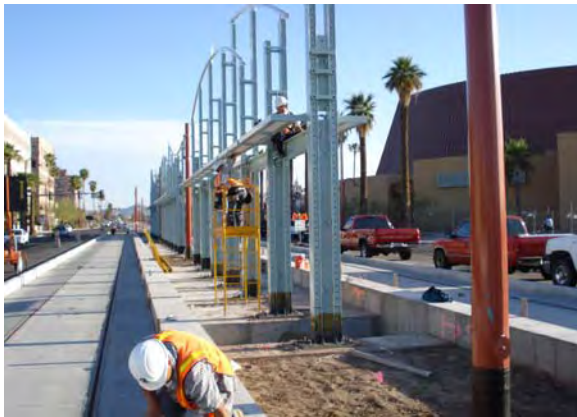
Campbell/Central Avenue Station Electrical Installation
