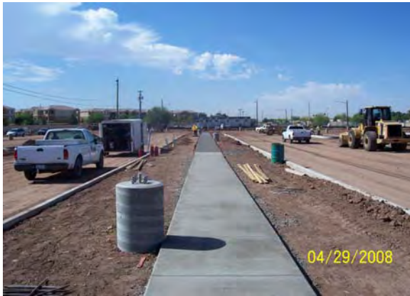
Sidewalk Installation - Price and Apache
