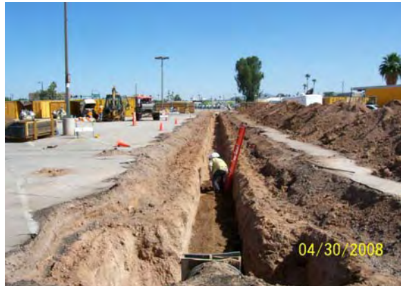
Storm Sewer Installation Montebello and 19 th Avenue
