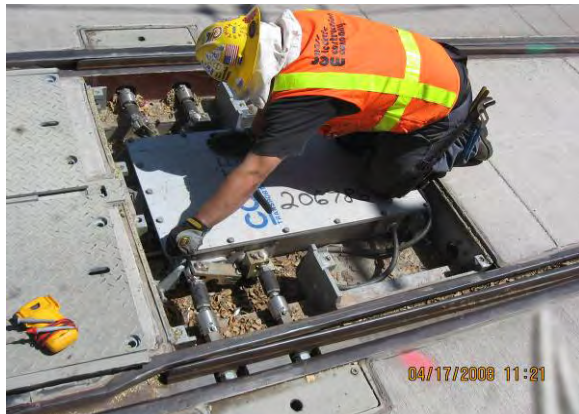
Adjusting Mainline Switch Machines at Mill Pocket Track
