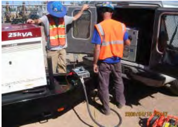
TPSS No. 12 – Testing Auxiliary AC Breaker
