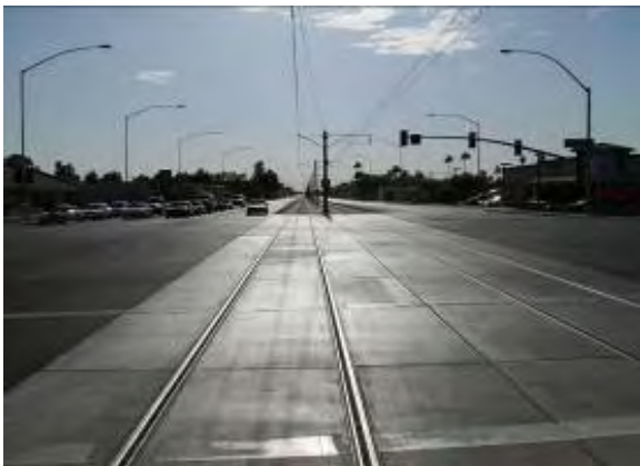
Completed Work at Dobson Road, Milestone H
