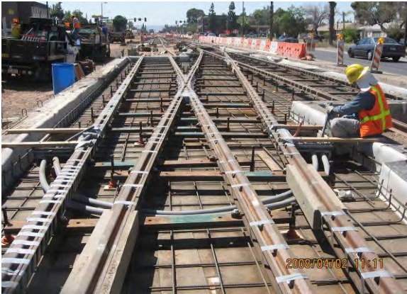
Installing Power Bonds at Montebello Interlocking
