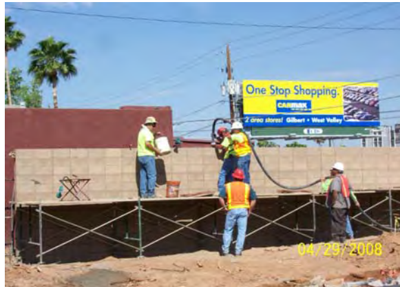
Screen Walls - Central and Camelback
