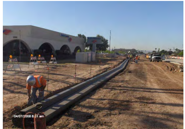
Placing Curb and Gutter on 19 th Avenue
