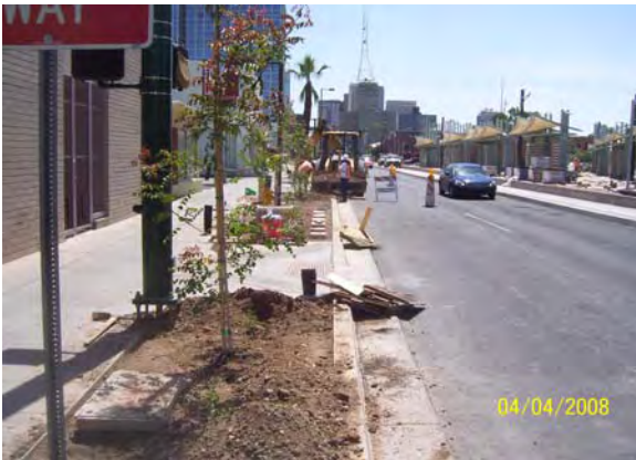
Placing landscape areas on Central Avenue
