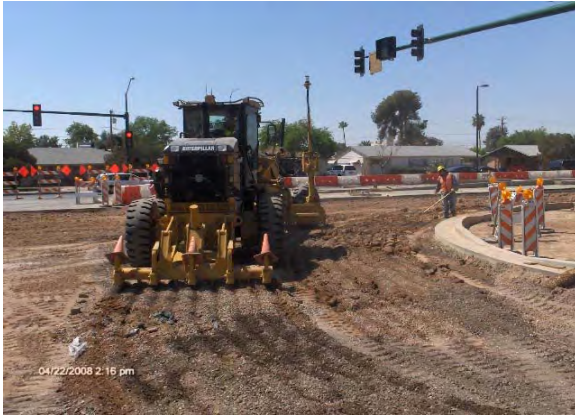
Scarifying the roadway subgrade for compaction
