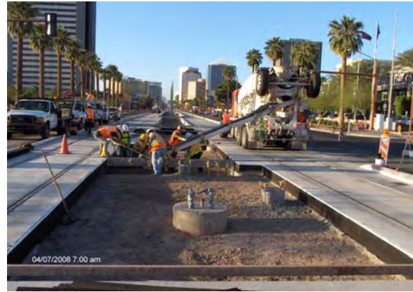
Placing Devil Strip
