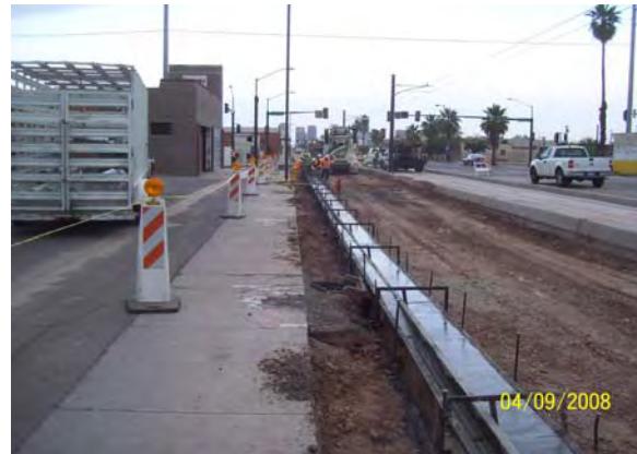
Placing curb and gutter on Washington
