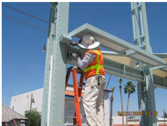
Terminating Public Address Speakers Cables at McClintock/Apache Station
