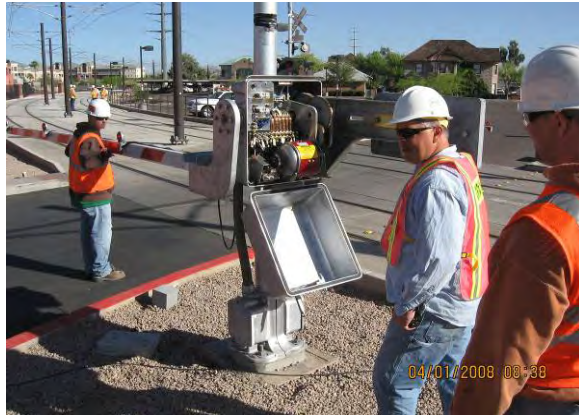
Testing Gate Crossing Mechanisms at Macayo's Crossing
