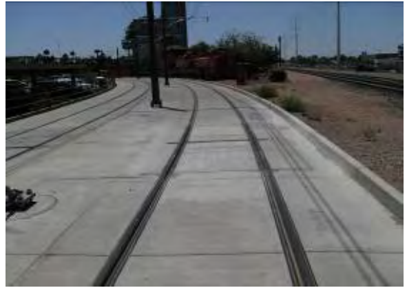
Completed Rail Repair, Milestone A
