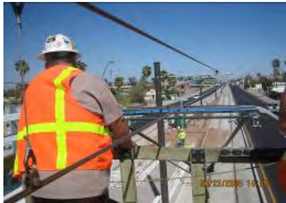
Aerial Inspections for OCS along Line Section 5
