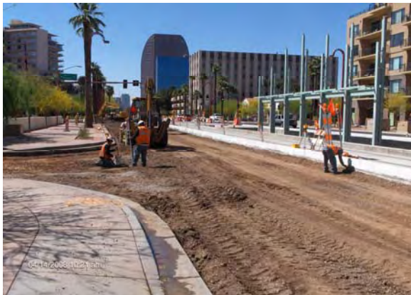
Sub-grade preparation Hoover Intersection
