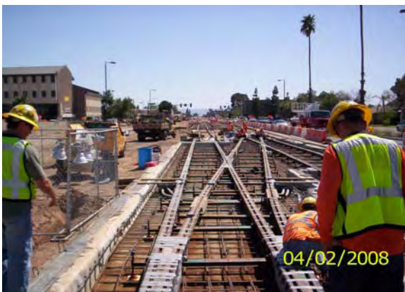
Installing special trackwork
