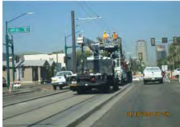
Line Section 3 – Stringing Messenger Wire for Wire Run 23
