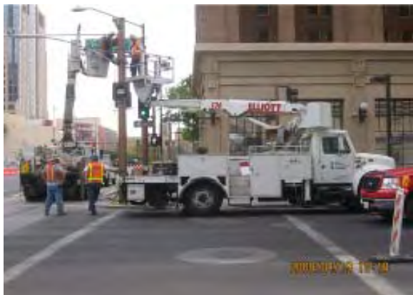
Line Section 3 – Installing Cantilever Arms for Wire Run 20
