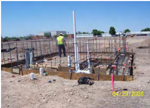
Security Building Footings - Sycamore and Main
