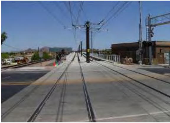
1 st Street, Ready for LRT Testing
