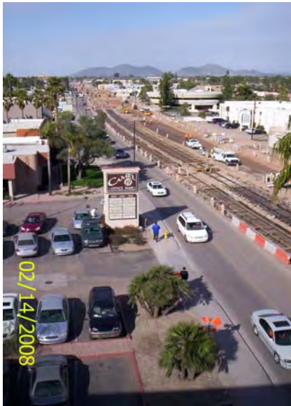
Guideway on 19 th Avenue ready to be poured
