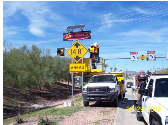
Solar Flasher Installation at SR 143
