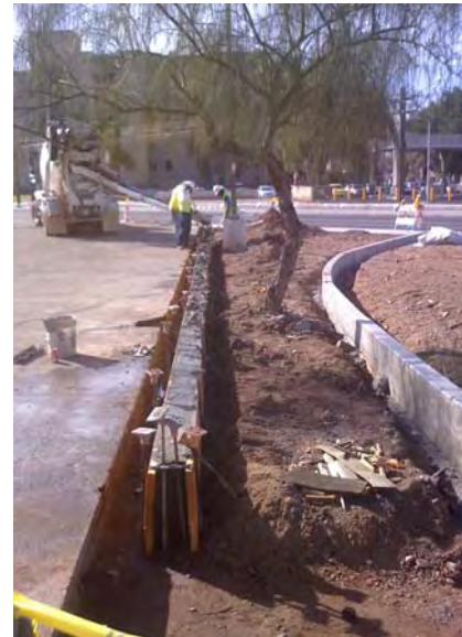
Parking Lot Mitigation Change Work, Milestone H
