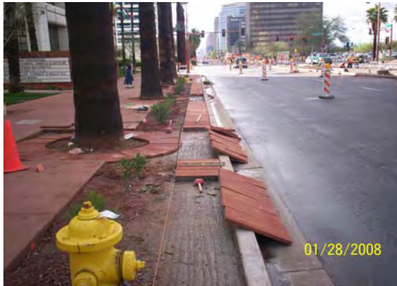
Installing Sandstone Pavers
