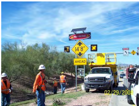
Solar Flasher Installation at SR 143
