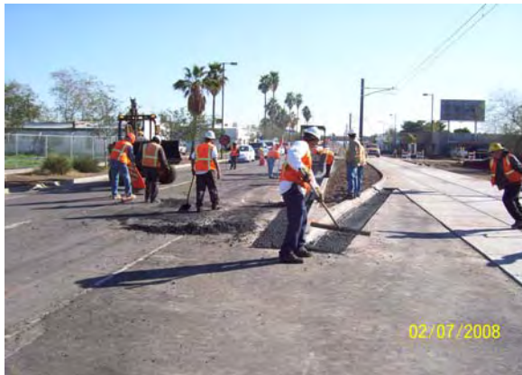
Paving at frontage road slip ramps
