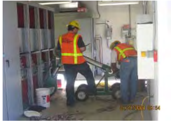
TPSS No. 11 – Pulling Positive Feeder Cables
