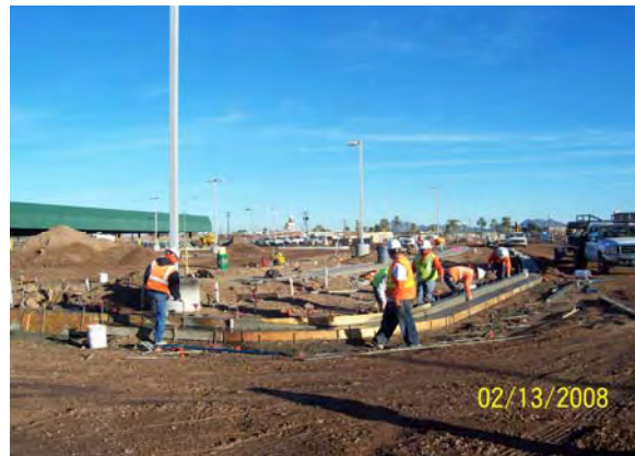
Curb and Gutter Installation 38 th and Washington
