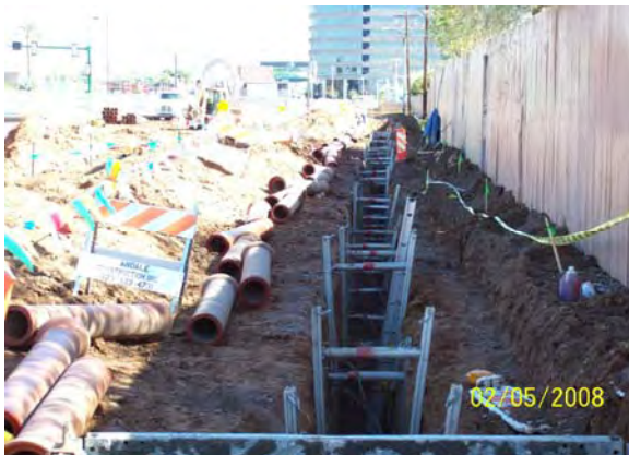
Sanitary Sewer Installation Central and Camelback
