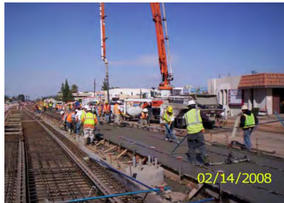
Guideway being poured
