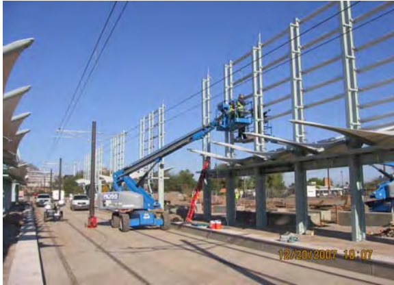
Louver Installation at University and Rural Station
