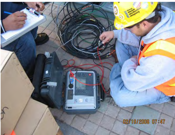
Performing Communications Cable Testing at 12th/Jefferson Station
