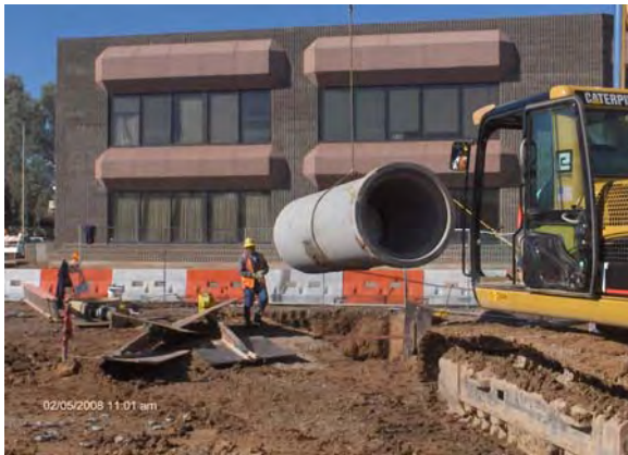
Installing 48" RCP pipe for offset Manholes
