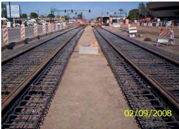
Guideway ready for Concrete
