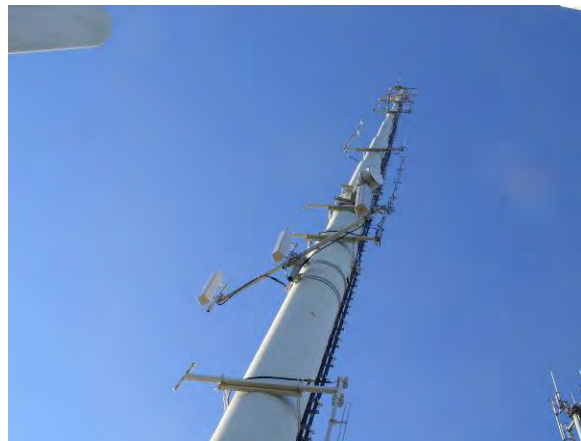
Installation of Data Radio Tower Equipment at South Mountain Tower
