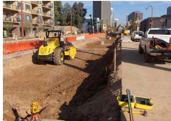
Compacting Encanto Station Foundation
