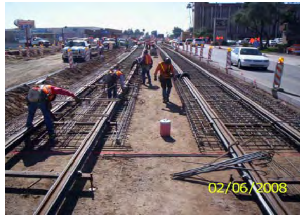
Crews placing Rebar for guideway on 19 th Avenue
