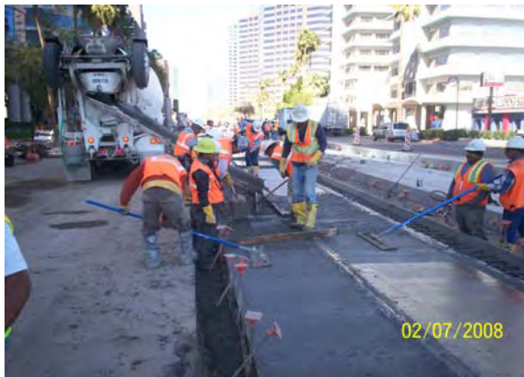
Placing Guideway Virginia to Roanoak
