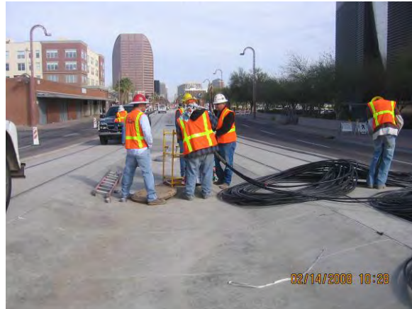
Pulling Signal Cable at Culver Interlocking
