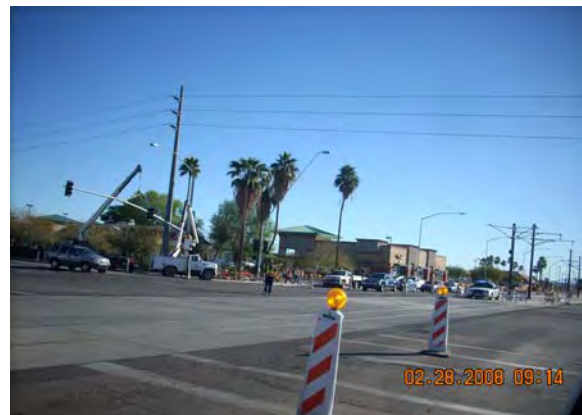
Traffic Signal Punchlist Work, Mesa, Milestone H
