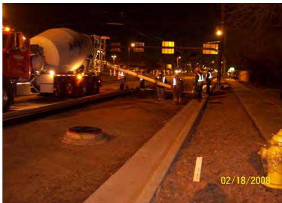
I-10 and Washington Concrete Paving
