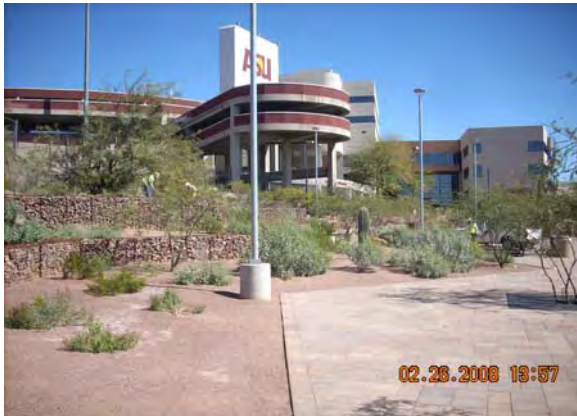
Landscaping Punchlist Work, ASU Promenade, Milestone G
