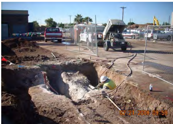
Ductbank Punchlist Work, Tempe, Milestone C
