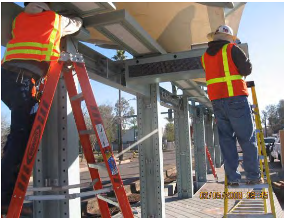
Installation of Visual Message Boards at 12th/Washington Station
