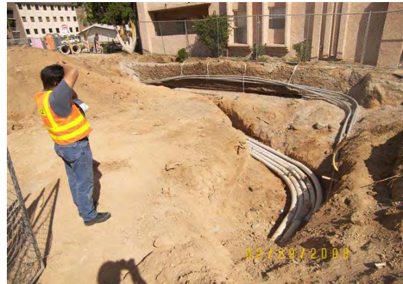
LS1 – Utility relocation done
