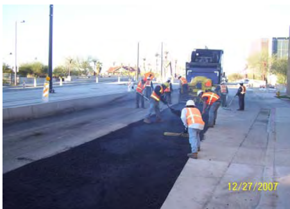
Frontage Road Subgrade
