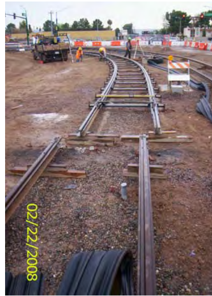
Crews lining track in curved section
