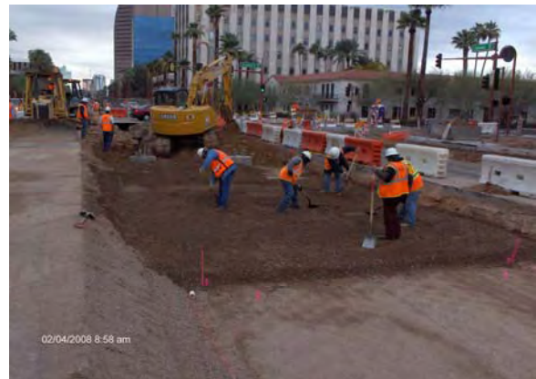
Encanto Station OCS Poles placed Grading for Ground Grid
