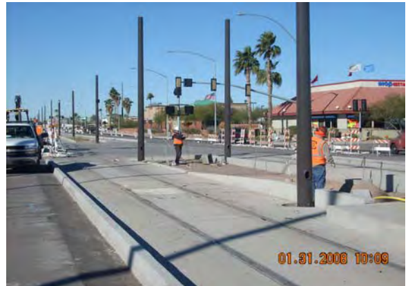
Traffic Signal Work, Mesa, Milestone H
