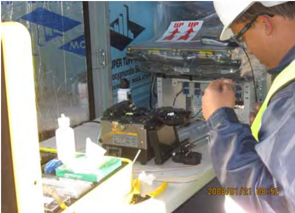
Splicing Communications System Fiber Optic Cable at 3 rd and Mill Station
