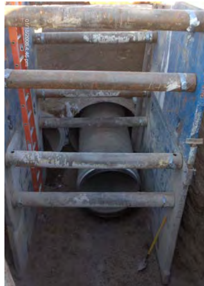
48" waterline Tie-in to existing 45-inch waterline
