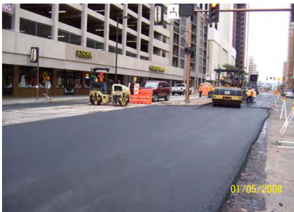
Rubberized Asphalt Paving on 1 st Avenue
