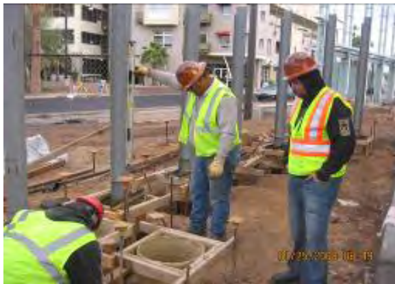
TPSS No. 5 – Installing Louver Posts
