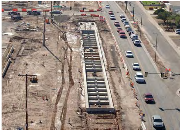
Montebello Avenue Station Foundation Complete
