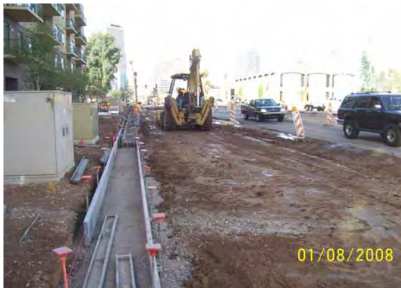
Forming Curb and Gutter
