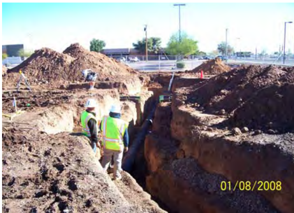
Storm Drain Installation 38 th and Washington
