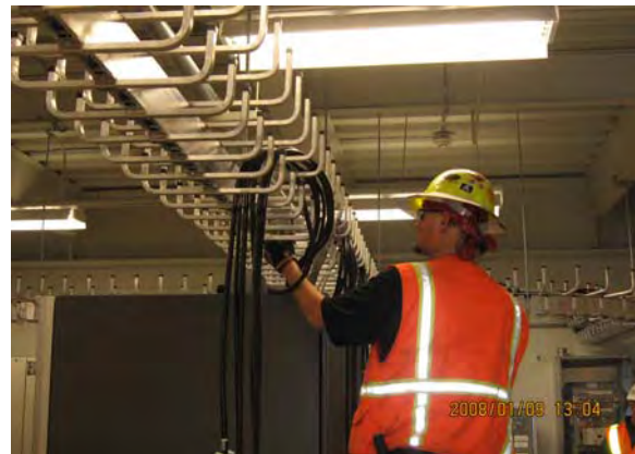
Installation of Communication System Fiber Optic Cables at MOE
