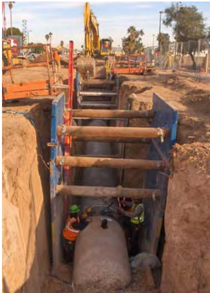
Installing 48-inch waterline
