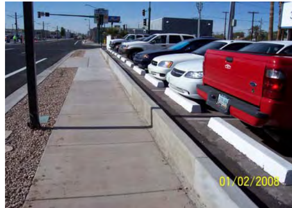
TCE back of walk restoration
