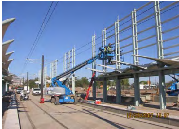
Louver Installation at University and Rural Station
