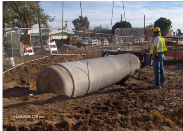
Installing new 48-inch waterline
