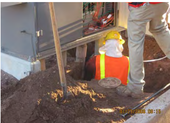
Infrastructure for Signal System Installation at Mission Palms Case
