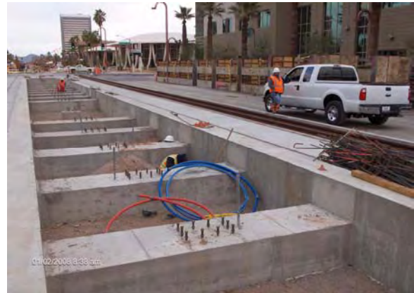
Completed Osborn Station Foundation
