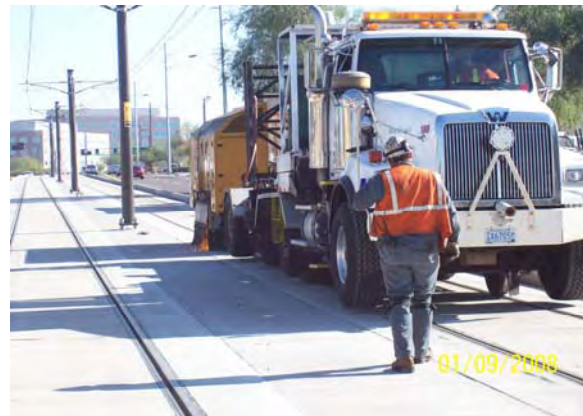
Rail Grinding at 54 th Place
