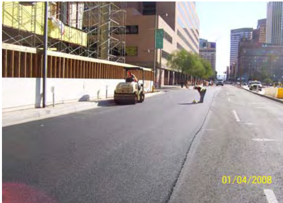
Placing rubberized paving on Central Avenue
