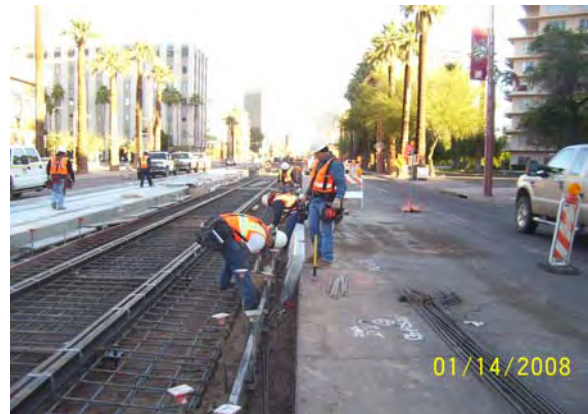
Installing Guideway Holly to Encanto
