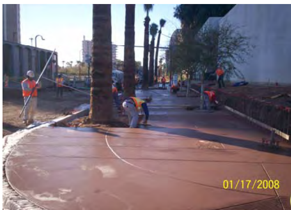
Placing colored sidewalk
