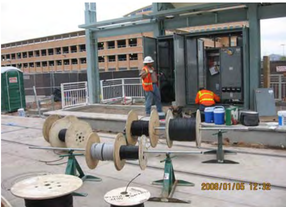
Communication System Fiber Optic Cable Installation at 3 rd and Mill Station
