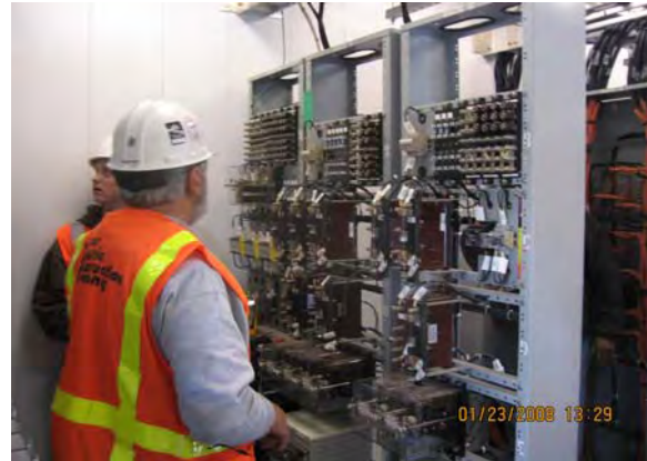
Performing Signal System Testing at Combined TPSS No. 7 (27 th Street Interlocking)
