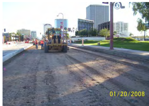
Prepare Sub-Grade for AC Paving
