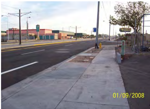
TCE back of walk restoration
