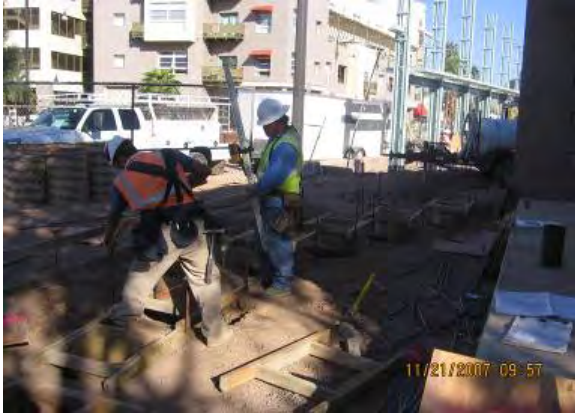
TPSS No. 5 – Setting Louver Posts
