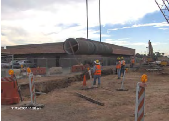
Laying 48-inch water line on 19 th Avenue
