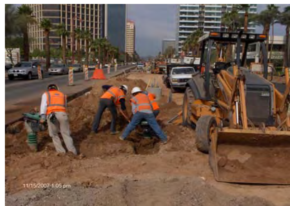
Installing Track Drains
