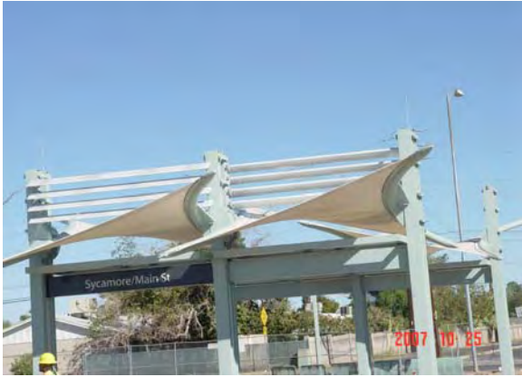
Louver Installation at Sycamore & Main Transit Center
