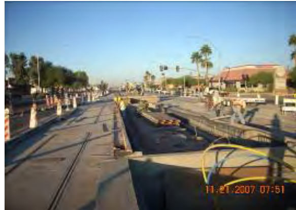
Sycamore Station Foundation, Milestone F
