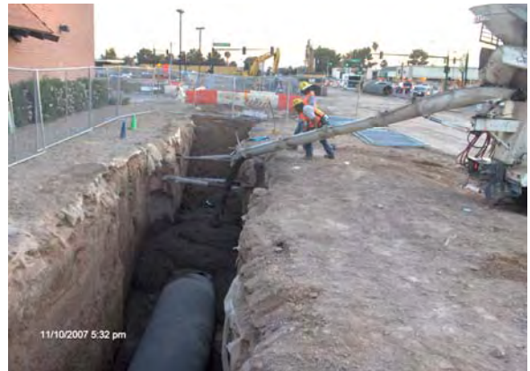
Placing slurry backfill above the 48-inch water line
