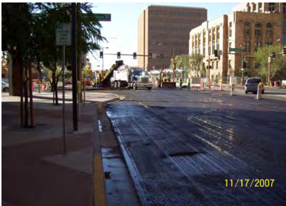
Milling of 1st Ave for Rubberized Paving
