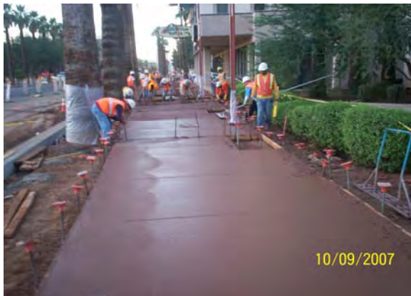
Placing Colored Sidewalk
