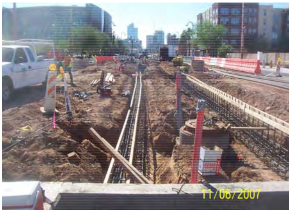
McDowell Foundation Ramps
