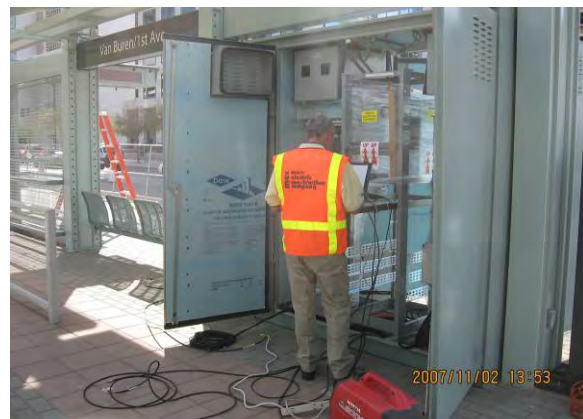
Internal Testing of Installed Communication Devices at 1st Avenue/Van Buren Station
