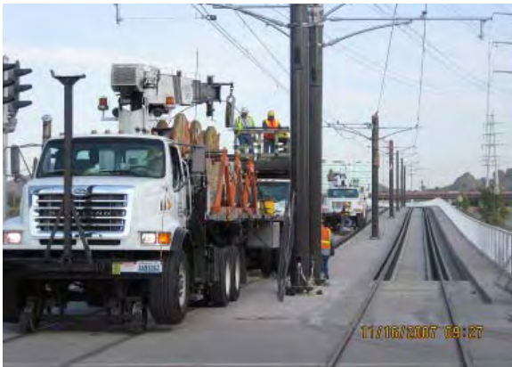
Stringing Contact Wire over Town Lake Bridge
