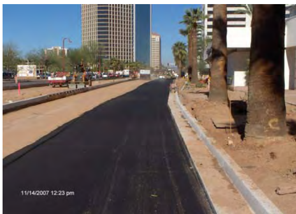
Placing AC Pavement Thomas to Osborn
