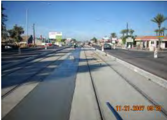
Station Platform at Dorsey Road, Milestone B
