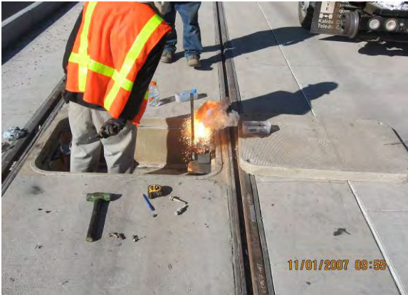
Installing Rail Bonds 27th Street Interlocking
