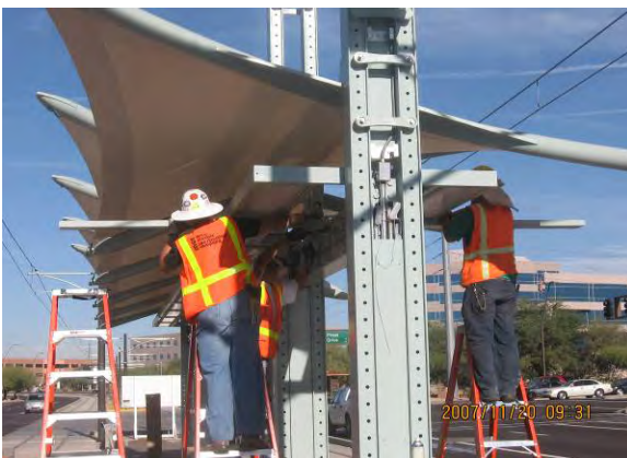
Mounting Cantilever Supports for Variable Message Boards at Priest/Washington Station
