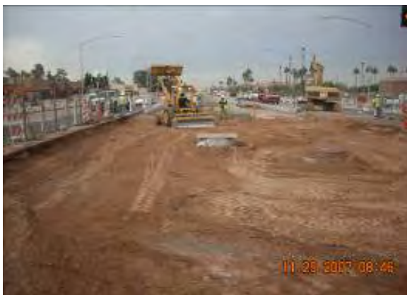
Sycamore Grade Crossing Work, Milestone F
