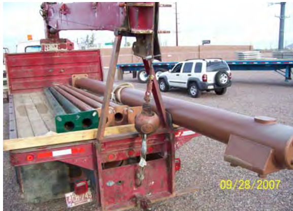
Signal Poles being issued to the LS3 Contractor
