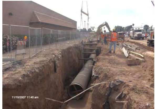
Laying 48-inch water line on 19 th Avenue
