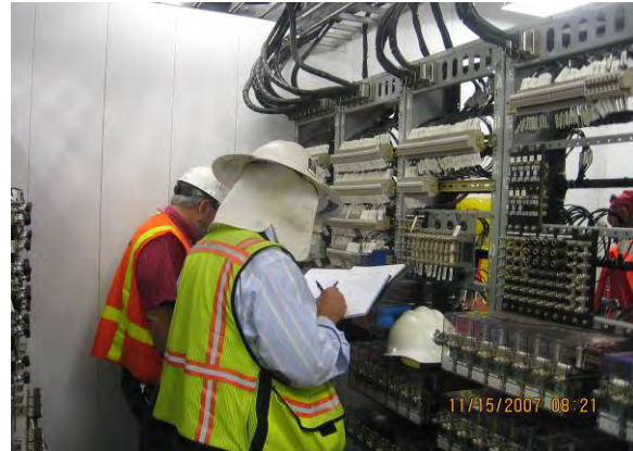
Performing Field Acceptance Testing at Signal Building No. 4
