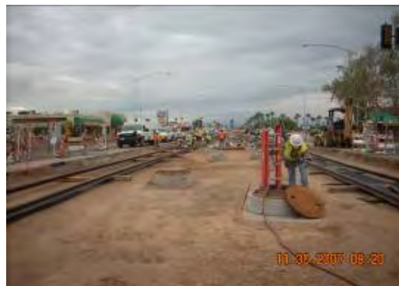
Guideway Work at the End of the Line, Milestone F
