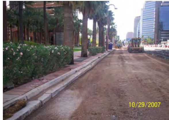
Checking Sub Grade prior to AC Paving
