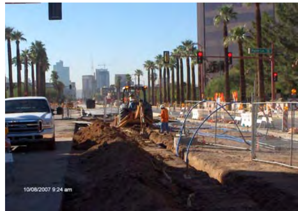
Installing Communication Duct Bank
