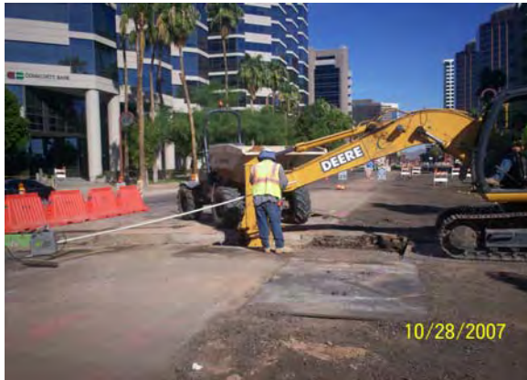
Placing Sanitary Sewer Virginia to Roanoke
