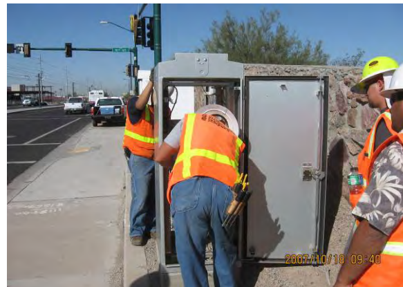
Installing Gator Patch for Street Traffic Controllers at 51st St./Washington Intersection
