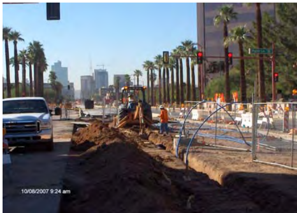
Excavating and placing duct bank
