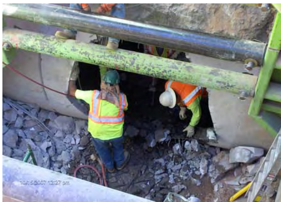
Installation of 54" offset man hole
