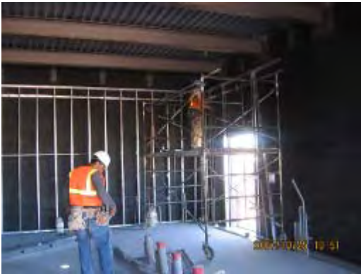
TPSS No. 12 – Installing Metal Stud Framing
