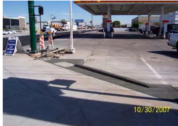
TCE Restoration at 30 th Street
