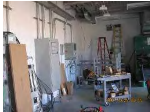
TPSS No. 13 – Installing Wall Mounted Equipment
