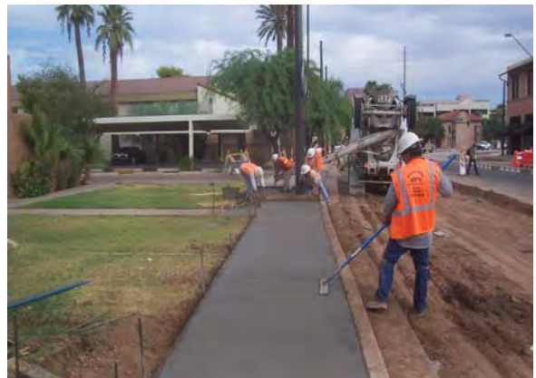
Sidewalk placement on 1st Avenue
