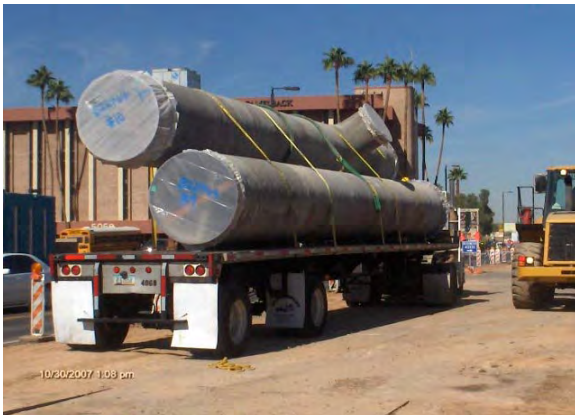
KWC's 48-inch water line joints 9 and 10 being delivered
