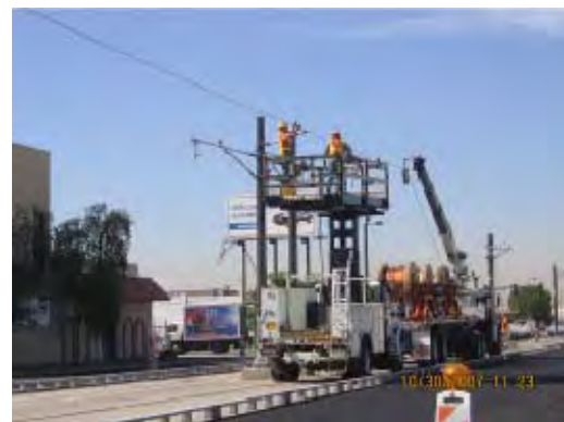
LS4 – Stringing Messenger Wire for WR 31
