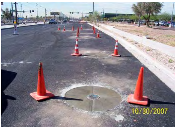
Raising Manholes and Valves Boxes
