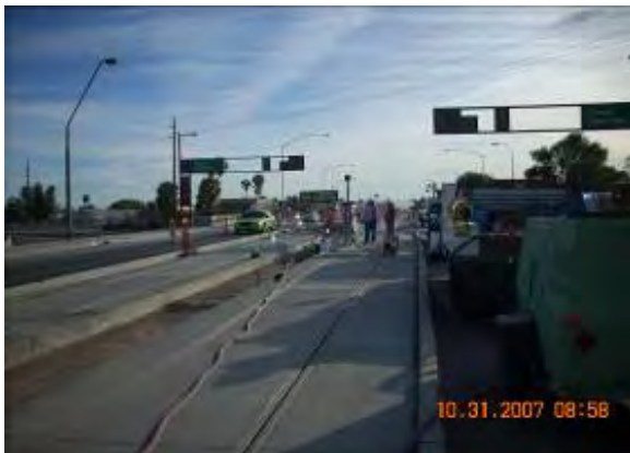
Trackway at Tempe Canal Bridge, Milestone D
