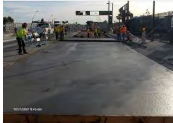
Pavement Replacement at Price Road, Milestone C
