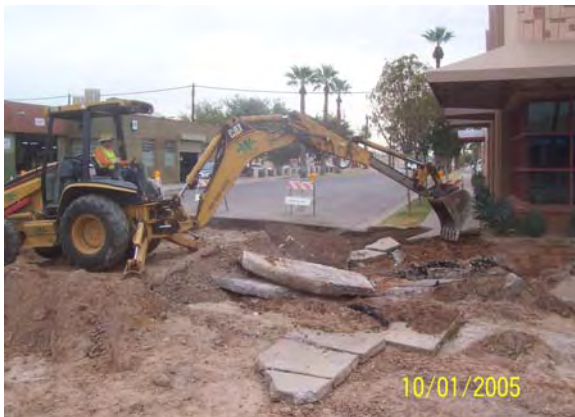
Roadway removal on Central Avenue
