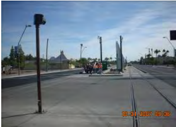
Station Platform at Dorsey Road, Milestone B
