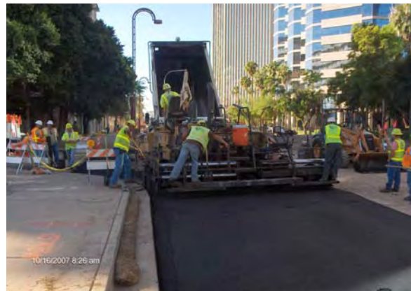
Placing AC Pavement base coarse
