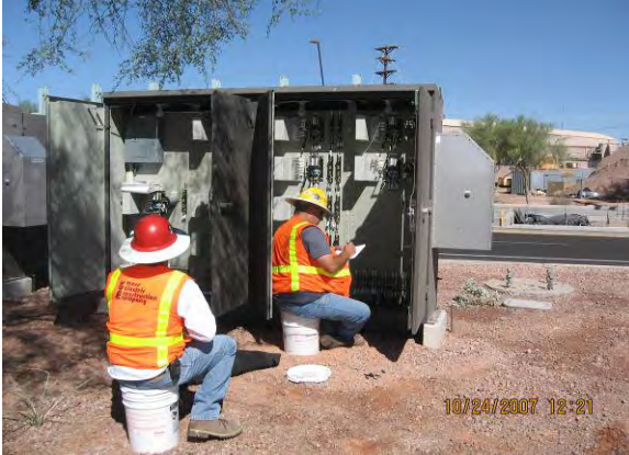
Terminating Signal Cables at Washington Grade Crossing Signal Case
