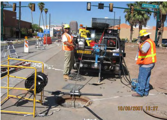
Pulling Signal Cable at McKinley Street Loop Interlocking
