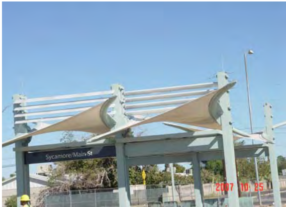
Louver Installation at Sycamore & Main Transit Center
