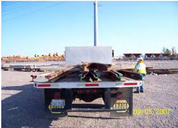
Issuance of the frogs for Turnout 3-1, 3-2, 3-3, 3-4 to the LS3 Contractor
