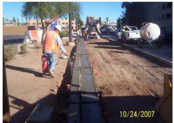
Curb and Gutter install on 1st Avenue
