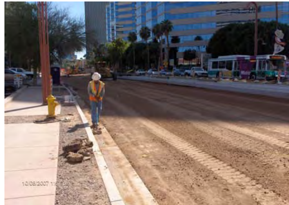
Checking Sub Grade prior to AC Paving
