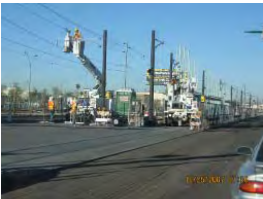
LS4 – Pre-Regulating Cantilever Arms for WR 31 and 32
