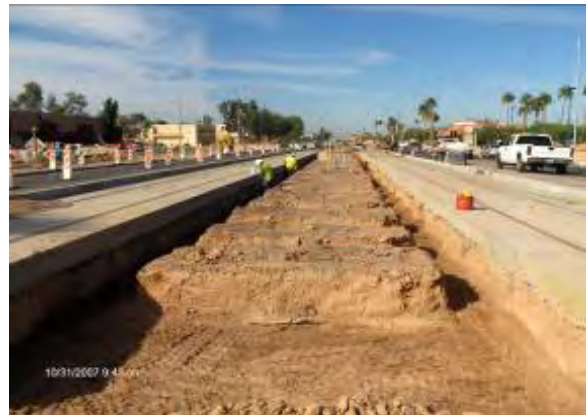
Sycamore Station Foundation, Milestone F
