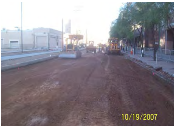
Roadway subgrade prep on Central Avenue
