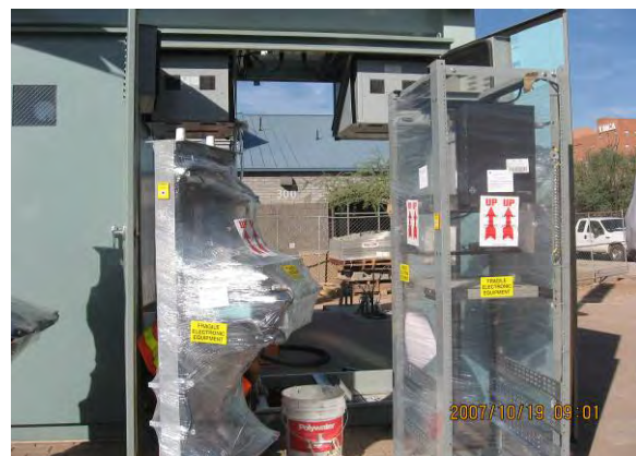
Setting Communication Rack Equipment at Central/Van Buren Station
