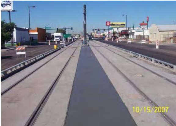
Concrete Devil Strip Placement east of 32 nd Street
