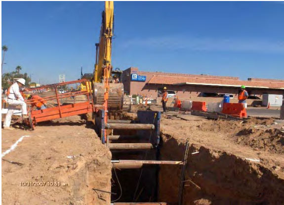
KWC continues to excavate for the new 48-inch water line
