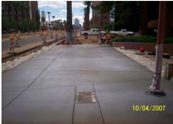
Placing Driveway at Cypress
