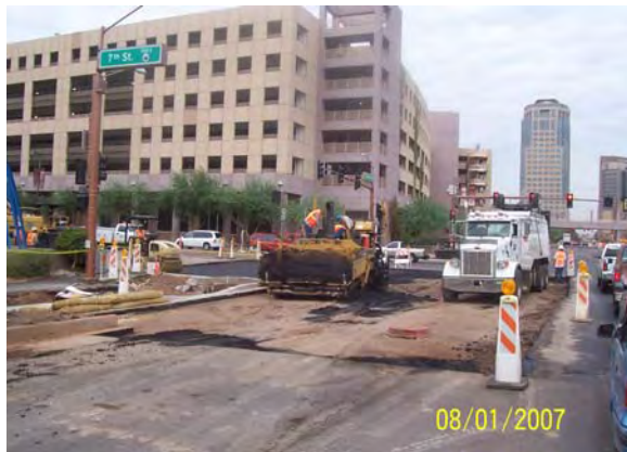
Asphalt paving Placement at 7th Street/Washington
