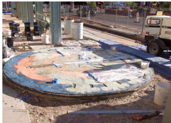
1 st Avenue/Jefferson Station Artwork Installation
