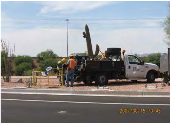
Washington Signal Case Pulling Cables to Signal Case
