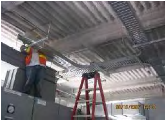
TPSS Number 7 – Installing Cable Tray Covers
