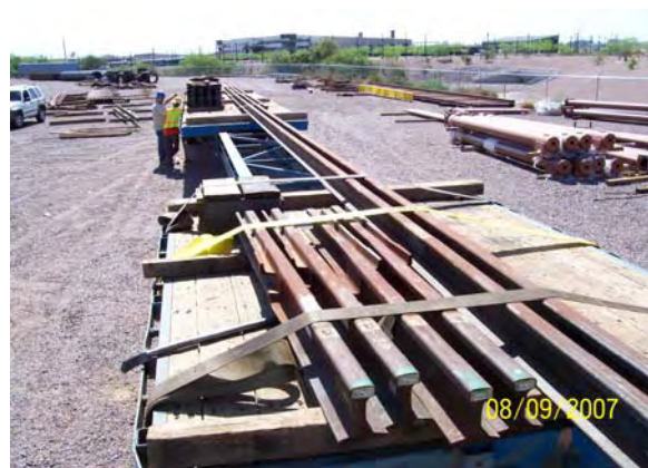
Issuance of Direct Fixation Rail for Northern Termination Point
