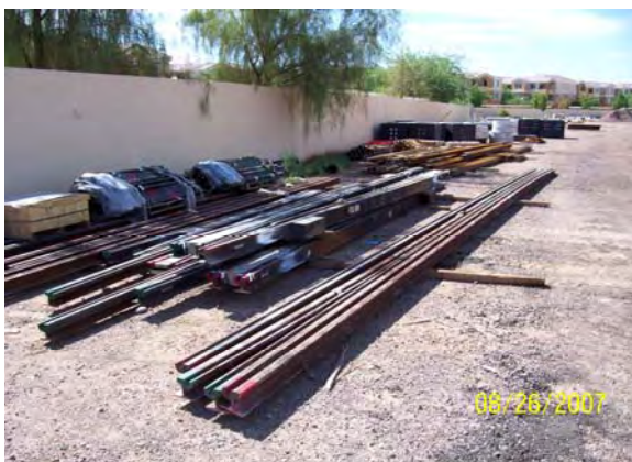
Delivery of two 100-Meter Crossovers to the Contractor's Storage Yard at LS5
