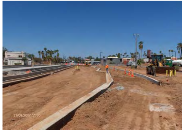
Central/Camelback Transit Center Sitework
