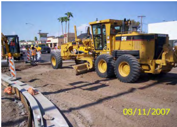
KWC preparing the Roadway Subgrade
