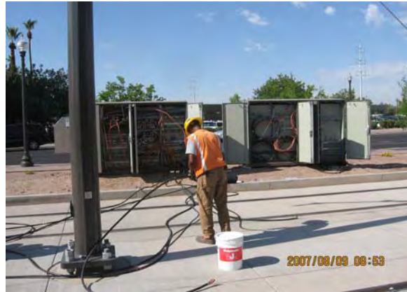
University Signal Case Preparing to Pull Cables at Signal Case
