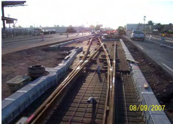
Crossovers 4-1/4-2 Track Work at 27 th Street
