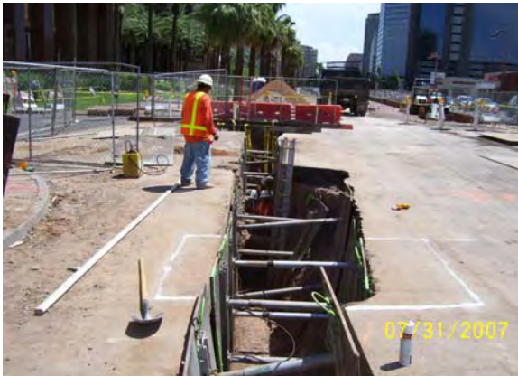
Installing Sanitary Sewer
