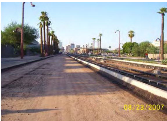
Sub-grade preparation for AC Paving
