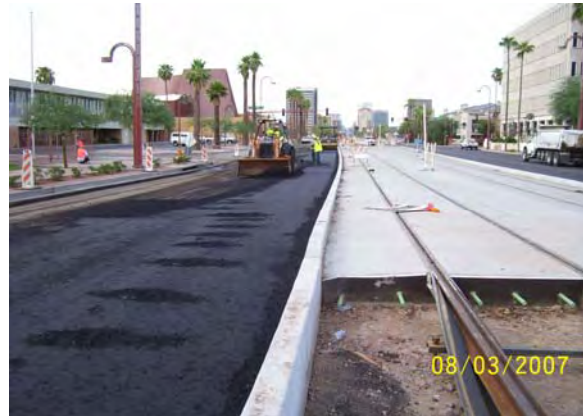
AC Paving North Bound at Central High
