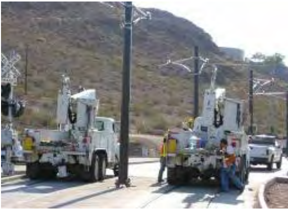
LS5 – Installation of Cantilever Arms
