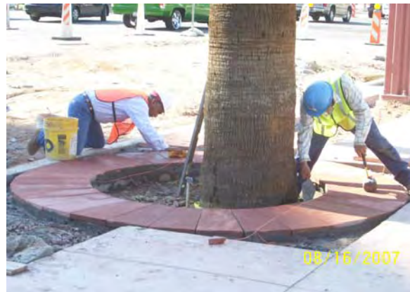
Placement of Tree Well Sandstone pavers
