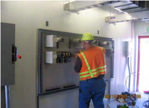
Signal Room Number 1 Installing Wall Mounted Signal Equipment
