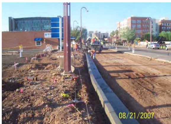
Curb placement for realigned ROW on Central Avenue
