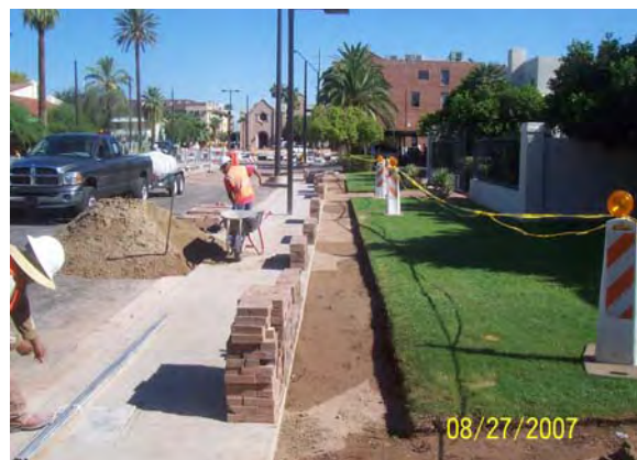
Sidewalk installation on 1st Avenue
