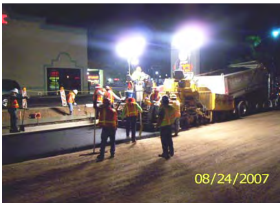
AC Paving - Crews placing AC on Camelback Road near 11th Avenue.
