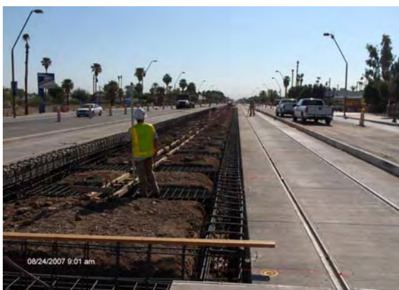
Foundation and Track at Smith-Martin Station
