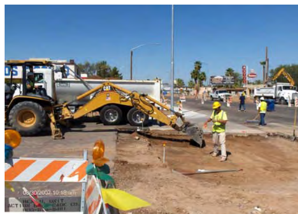
Roadway Work in Mesa
