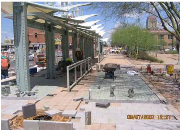
1 st Avenue/Van Buren Paver Installation
