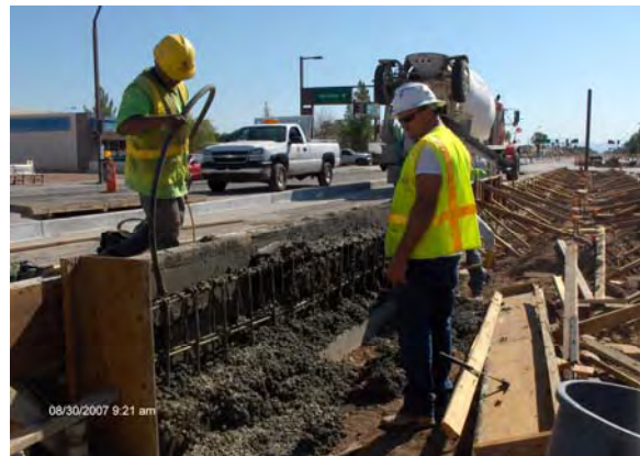
East Ramp Wall Placement at McClintock Station
