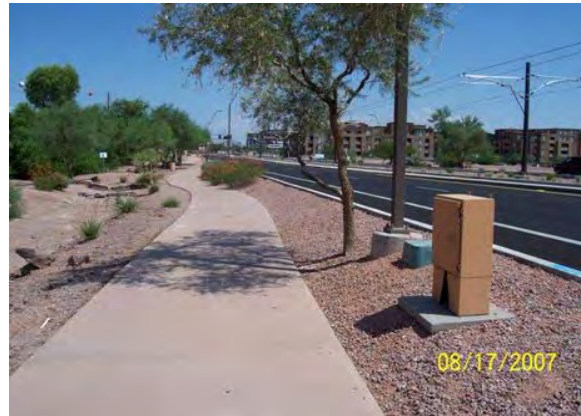
Completed Work West of Center Parkway
