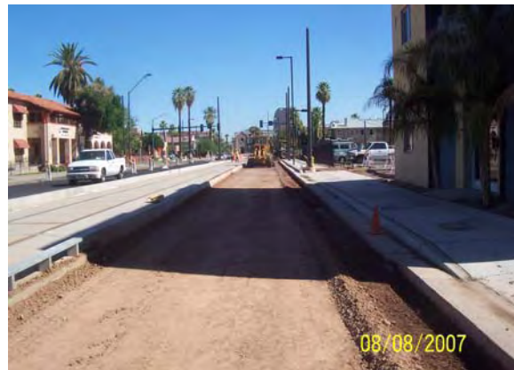
Subgrade preparations on 1st Avenue
