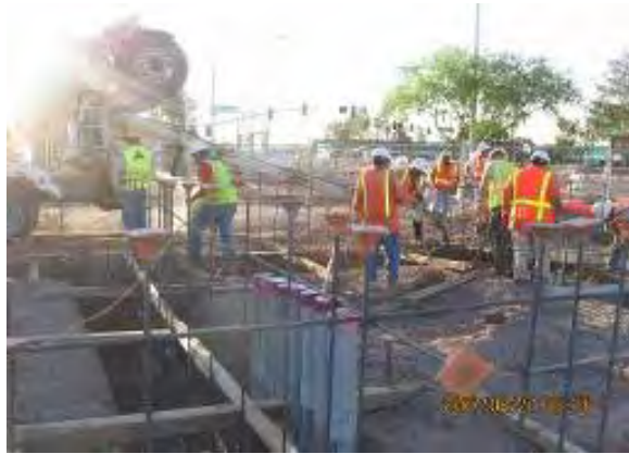
TPSS Number 14 – Concrete Placement for Footings
