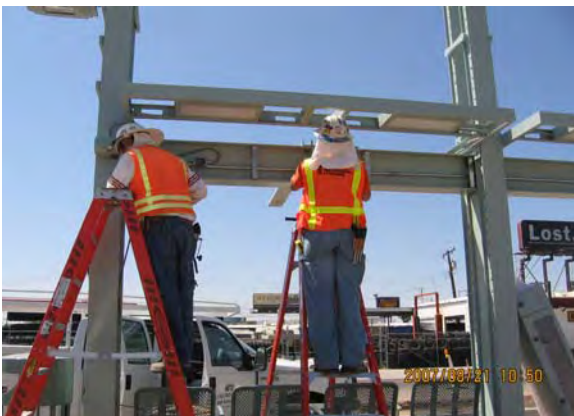
Mounting Public Address Speakers at 24th/Jefferson Station Platform
