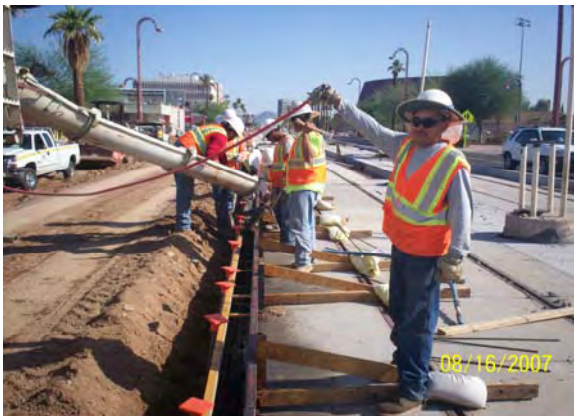
Placing Guideway Curb
