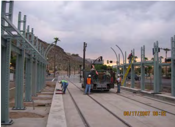
3 rd /Mill Avenue Structural Steel Installation
