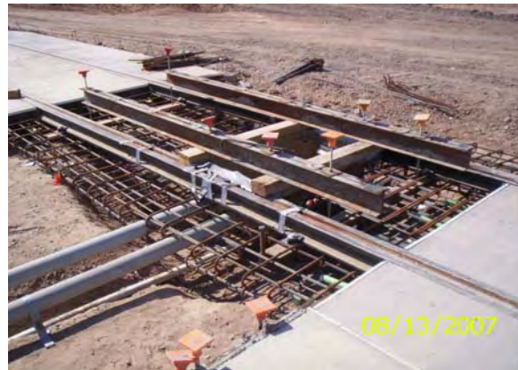
Crews tied rebar around the TPS boxes
