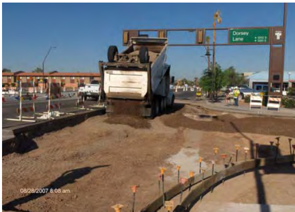
Full Depth Pavement Replacement at Dorsey Road
