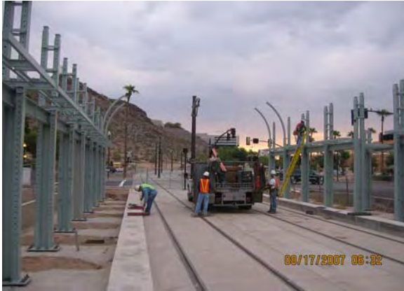
3 rd /Mill Avenue Structural Steel Installation
