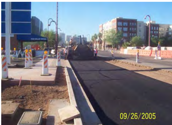
Placing Roadway Paving on Central Avenue
