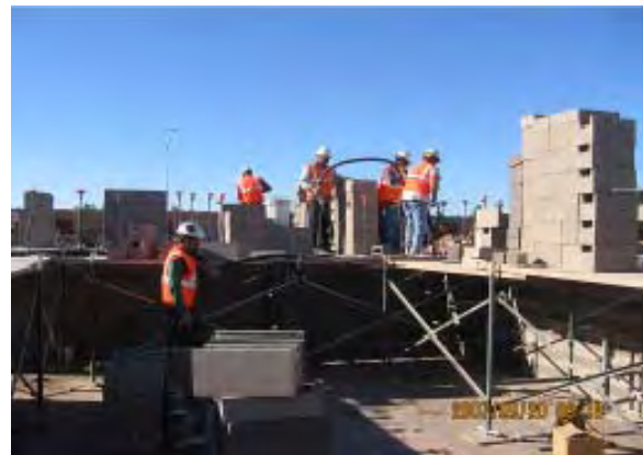
TPSS Number 14: CMU Block Wall Grout Placement
