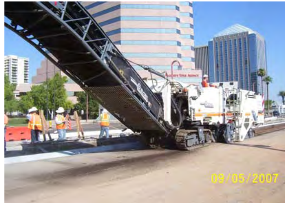
Milling pavement Columbus to Indianola
