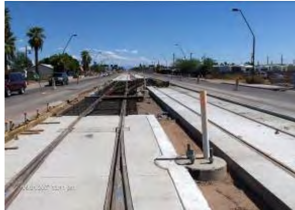
Trackway and Crossover East of River Road, Milestone C
