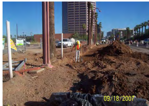
Roadway Widening on Central North of McDowell
