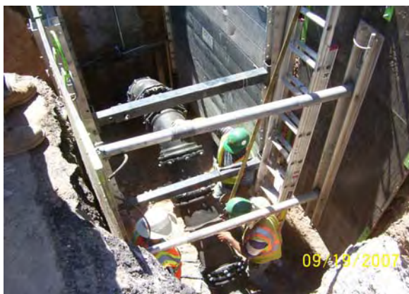
Installing DIP Water line
