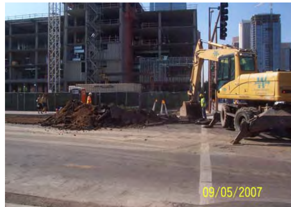
Roadway Pavement Replacement on Fillmore and Central Avenue Intersection
