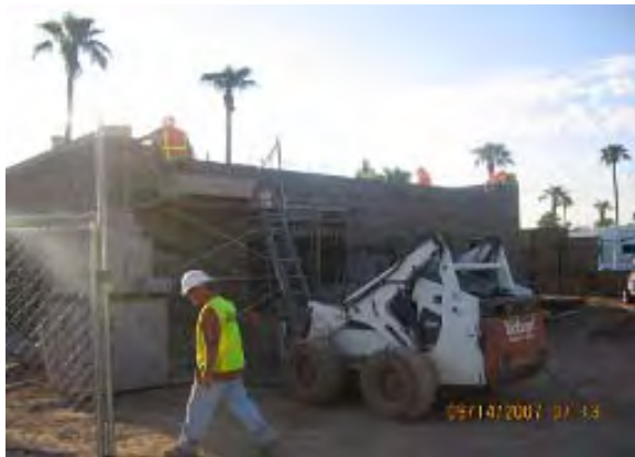
TPSS Number 12: CMU Block Wall Placement
