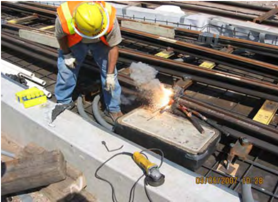
27th Interlocking Cadwelding Power Bonds to Rail
