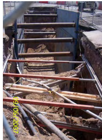
Utilities to work around during the 48" Waterline installation
