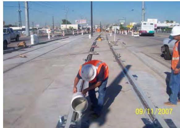
Final Elastomeric Grout Placement at the Washington Street Bridge
