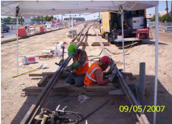
Rail grinding thermite welds
