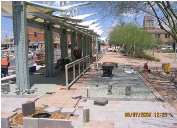
1 st Avenue/Van Buren Paver Installation
