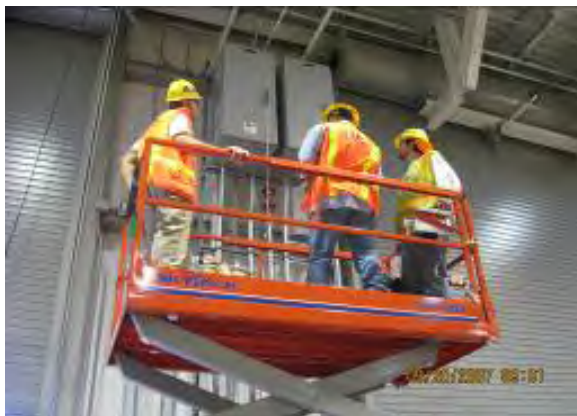
MOE Shop: Installing Permanent DC Disconnect Switches
