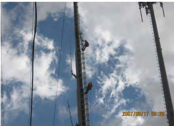
South Mountain Radio Tower Climbing Tower to Install Radio Antennae
