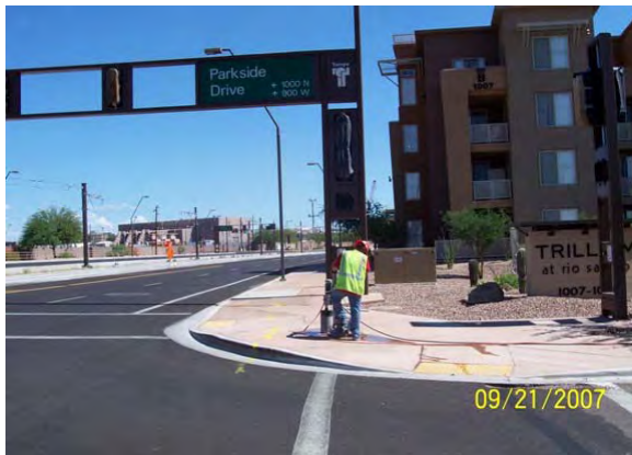
Coring operation for Survey Monument Placement at Parkside COT
