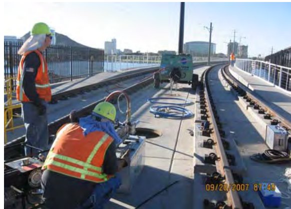
North End TTLB Manhole Blowing Backbone Fiber Cables into Ductbank
