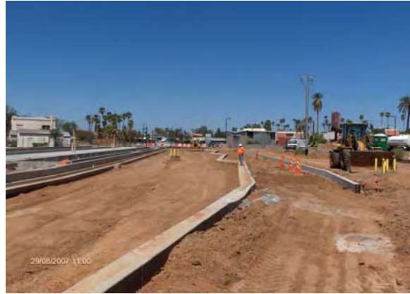
Central/Camelback Transit Center Sitework
