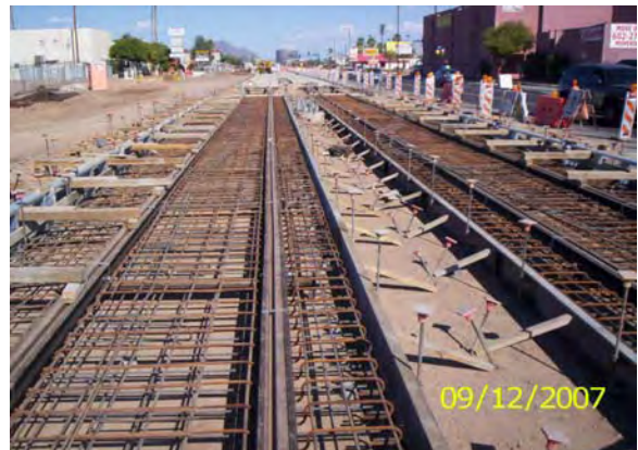
Placing rebar and forms for guideway pour
