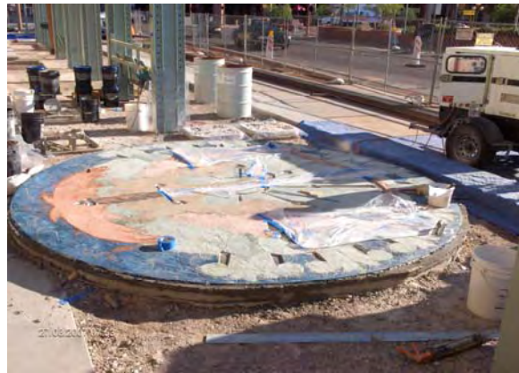
1 st Avenue/Jefferson Station Artwork Installation
