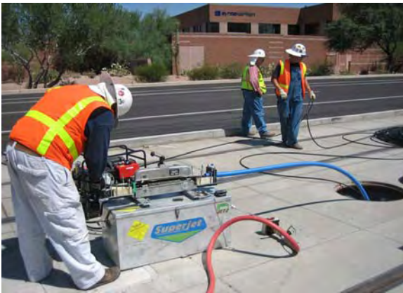
56th/Washington Manhole Blowing Backbone Fiber Cables into Ductbank
