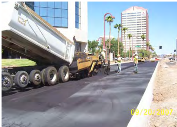
Placing AC Pavement Osborn to Catalina
