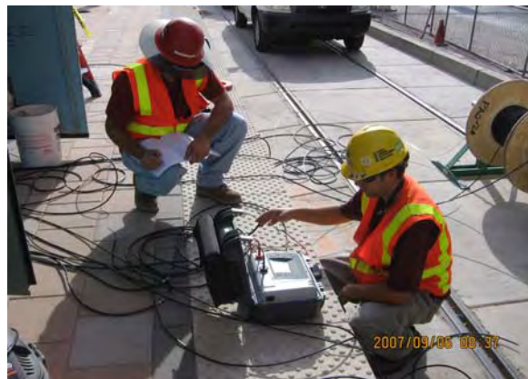
3rd/Washington Station Testing Communication Cables at Stations
