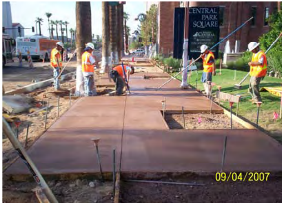
Placing Colored Sidewalk at 2020 Central
