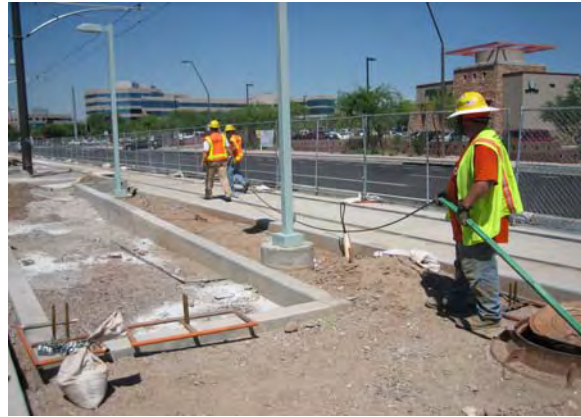
Priest/Washington Station Pulling Fiber Cable at Station Platform
