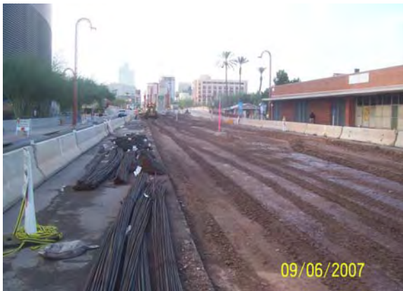
Guideway Subgrade excavation on Central Avenue
