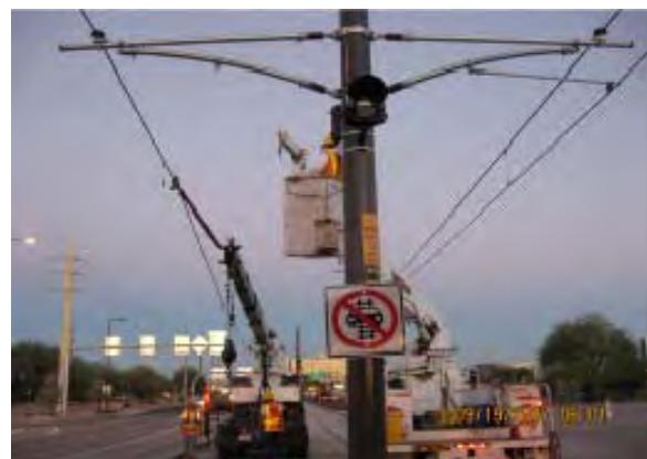
WR 36: Replacement of Messenger Wire
