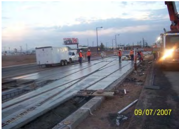
Special Track Work Concrete Placement at 27 th Street
