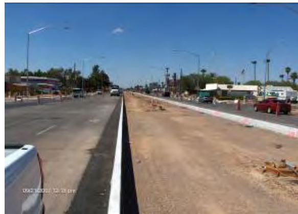
Guideway Work in Mesa, Milestone F
