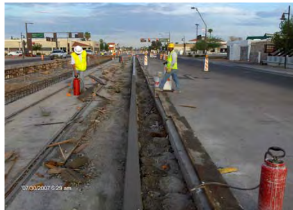
Apache Boulevard at McClintock Station, Milestone B
