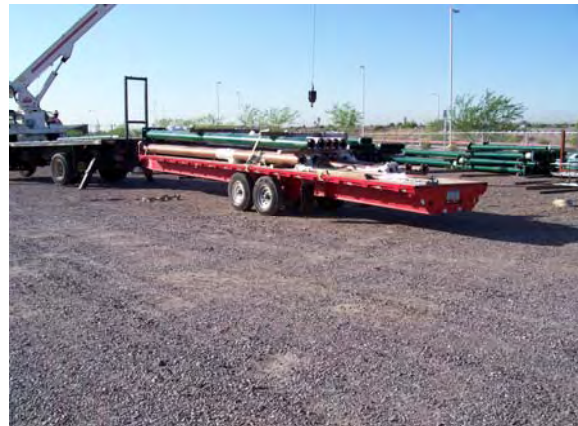
Traffic Signal Poles and Mast Arms being issued to the LS3 Contractor
