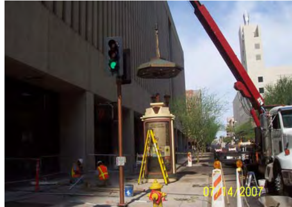
DPP Kiosk installation on 1 st Avenue
