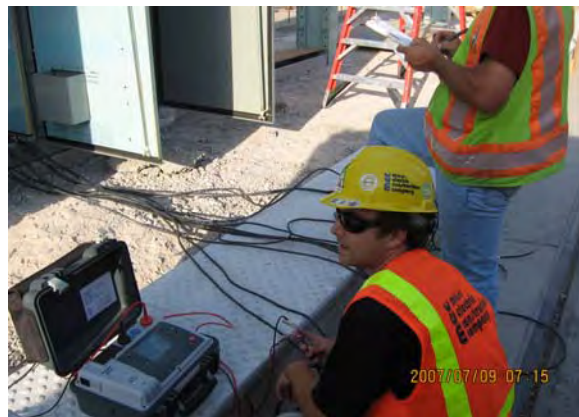
Post-Installation Testing of Communication Cables at 3rd/Jefferson Station
