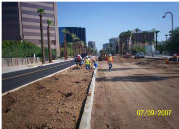
Sub Grade preparation Palm Lane to South end of Project
