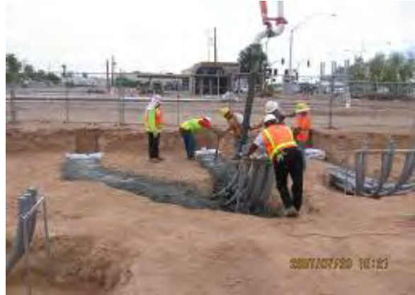
TPSS Number 14 – Concrete Placement for APS Conduits
