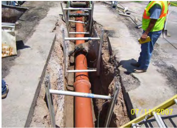
Installing Sanitary Sewer
