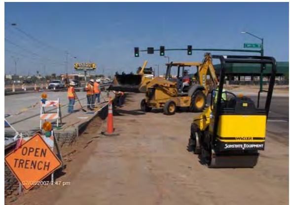
Slot Paving at the 32 nd Street Intersection
