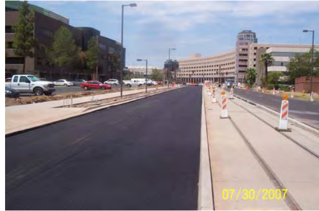
Jefferson frontage road paving
