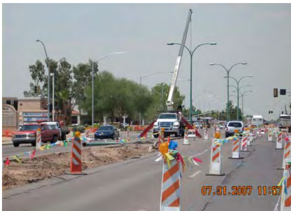
Removing Center Streetlights in Mesa, Milestone E2
