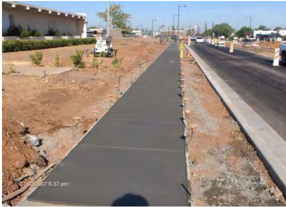
Sidewalk Construction at 26 th Street
