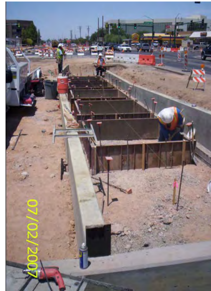
Crews forming the pad foundations for the 19th Ave Station
