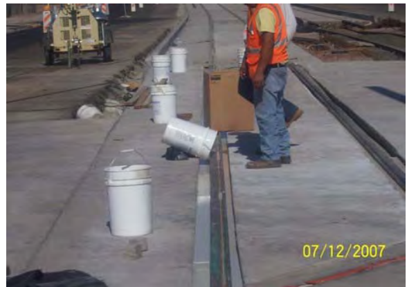
Placing Elastomeric Grout at the Washington Street Bridge
