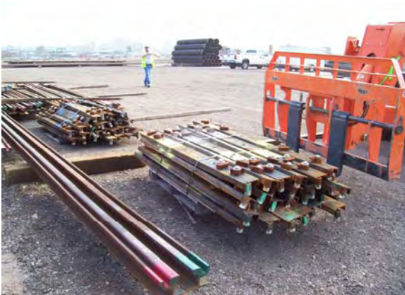
Delivery of two 100-Meter Crossovers to the Contractor's Storage Yard at LS2
