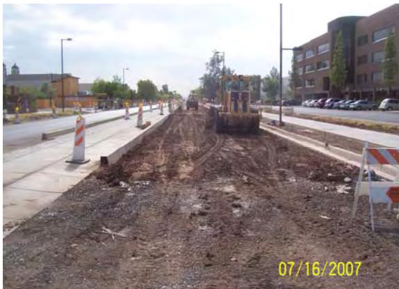
Jefferson frontage road subgrade preparation
