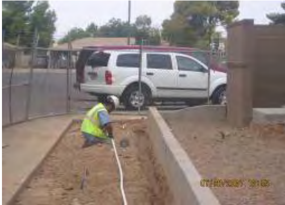
TPSS Number 1 – Installation of Irrigation line
