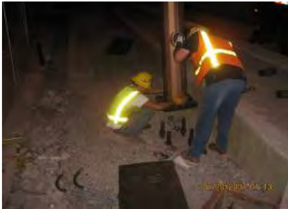
LS3 – OCS Pole Installation
