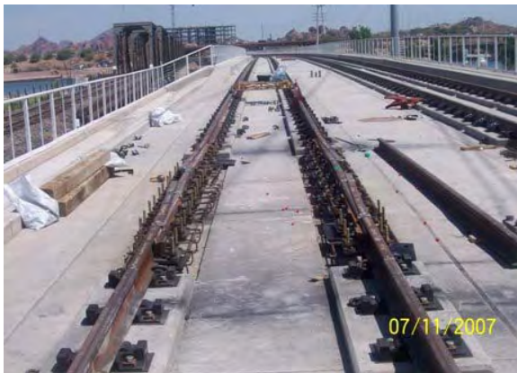
Track Expansion Joint Installation on the Tempe Town Lake Bridge
