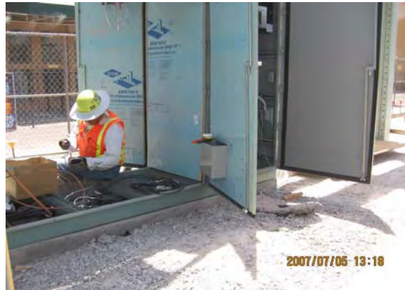
Pulling Communication Cable at Station Communication Cabinets
