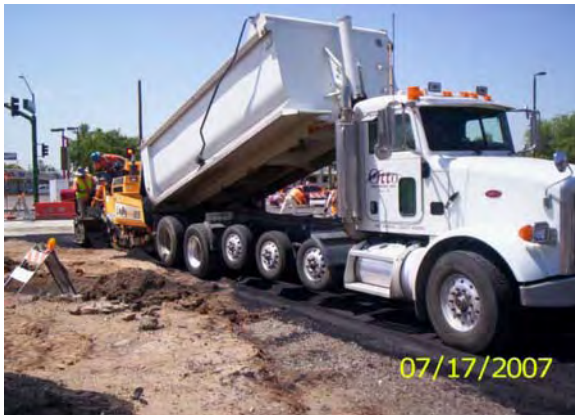
Temporary AC Paving
