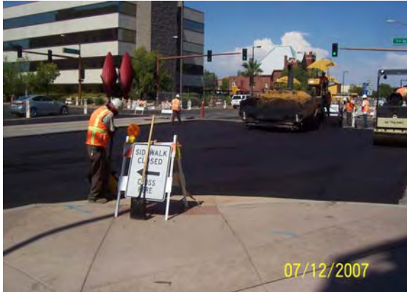
Roadway paving at 7 th /Jefferson
