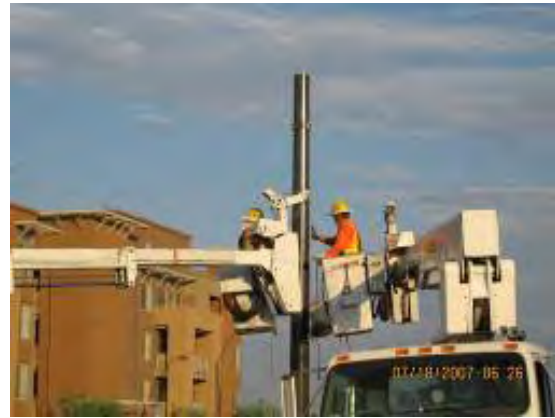
LS4 – OCS Pole Band Installation
