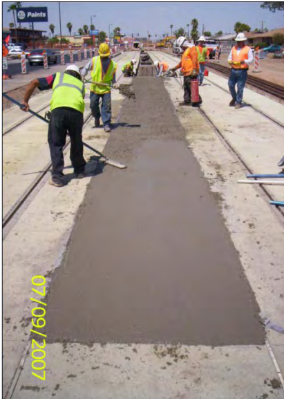
Crews placing concrete for the Guideway Devil Strip
