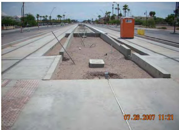
Dorsey Station and Track, Milestone B
