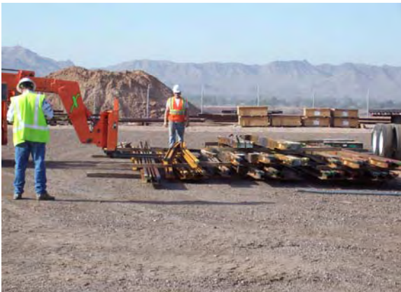
Delivery of two 100-Meter Crossovers to the Contractor's Storage Yard at LS2
