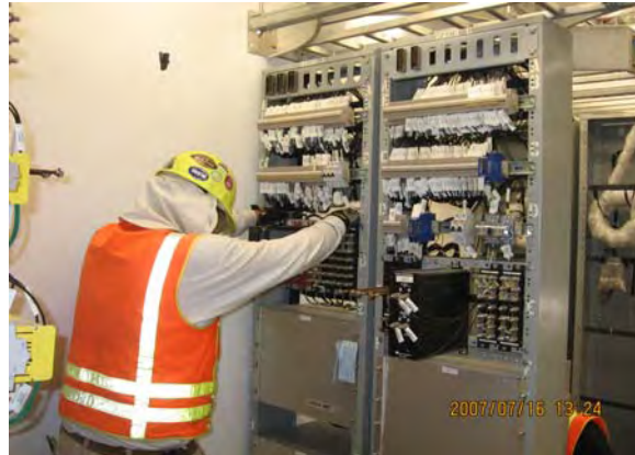
Signal Room Number 2 Installing Signal Rack Equipment
