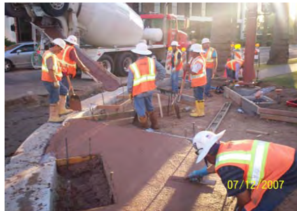
Placement of ADA /Sidewalk ramps
