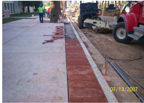
Installing San Stone borders
