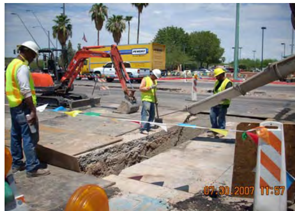
Utility Work in Mesa, Milestone F2
