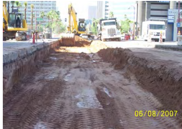
Excavation for Thomas Station
