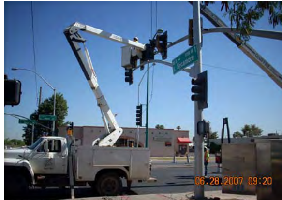
Traffic Signal Work in Mesa, Milestone E2
