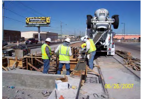
Ramp Construction at the 38 th Street Station
