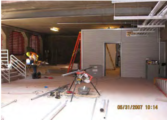
Signal Room Number 2 Completed Exterior Metal Panels
