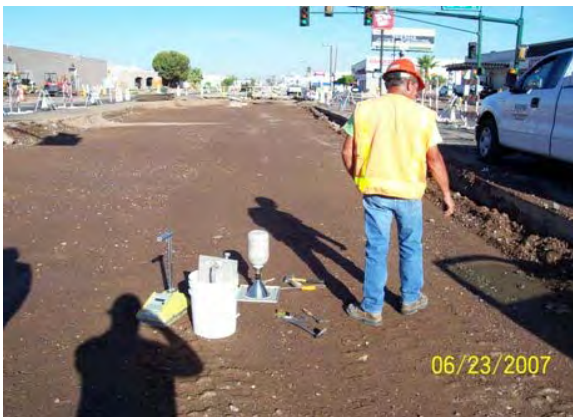
Checking of Sub-Grade Compaction in the Guideway
