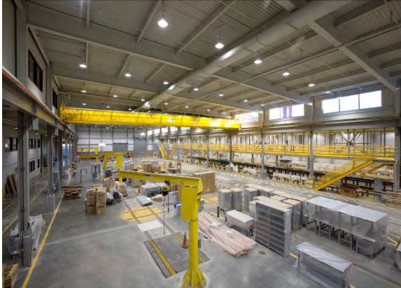
Maintenance of Equipment Building Shop Floor
