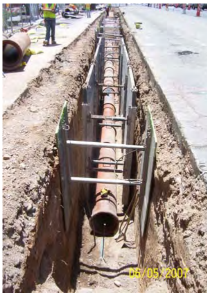
Installation of Sanitary Sewer
