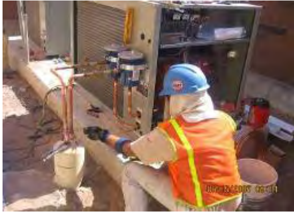
TPSS Number 3 – Installing HVAC Lines to Condenser Unit
