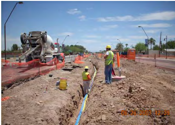
Guideway Ductbank on Apache Boulevard, Milestone C2
