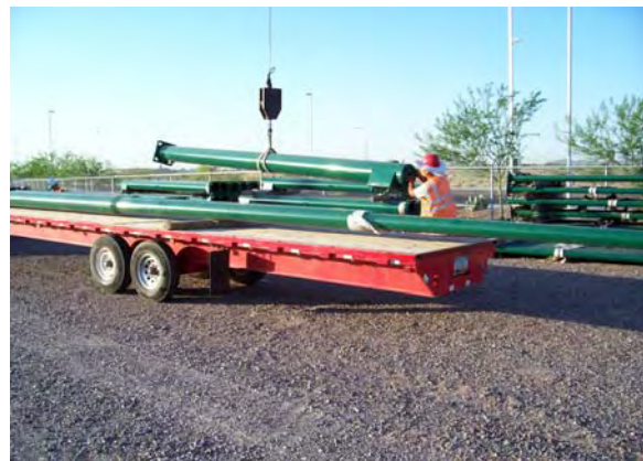
Traffic Signal Poles and Mast Arms being issued to the Line Section 3 Contractor
