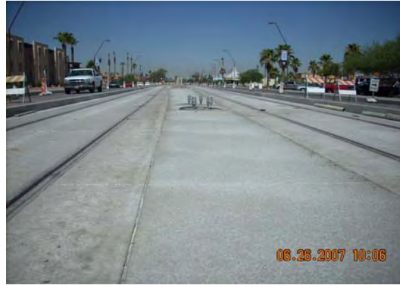
Guideway on Apache Boulevard, Milestone B2
