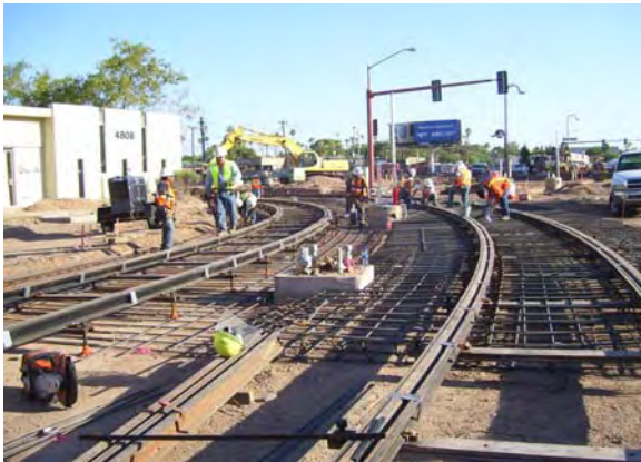
Curve Rail installation at Central crossing
