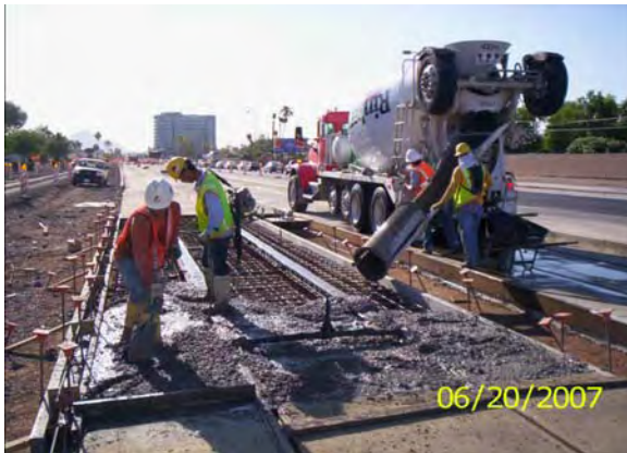
Guideway - RGG crews placing concrete for the Guideway section
