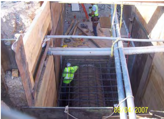
Concrete encasement of 48-inch water line
