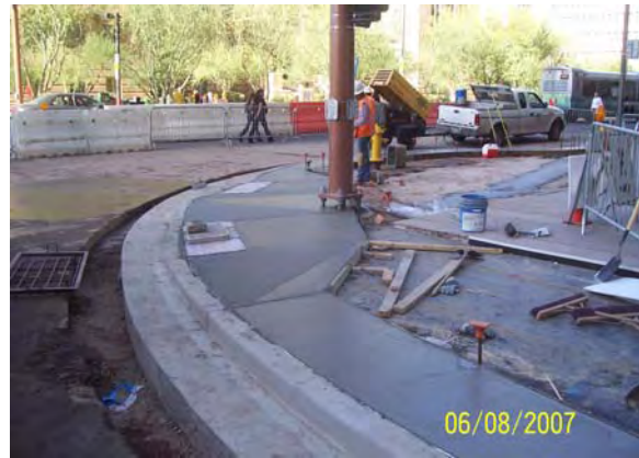
Ramp and sidewalk placement at 1st Avenue/Washington
