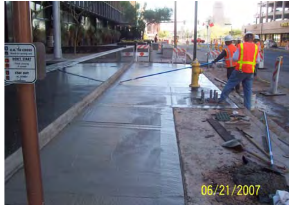
Sidewalk placement on 1st Avenue at Federal Building
