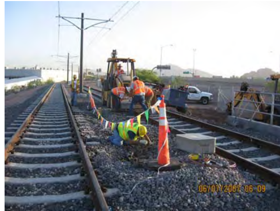
MSF Yard Entrance Ductbank Modifications
