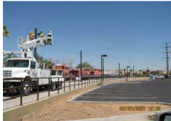
LS5 – Installation of OCS Poles (WR 43 and 44)
