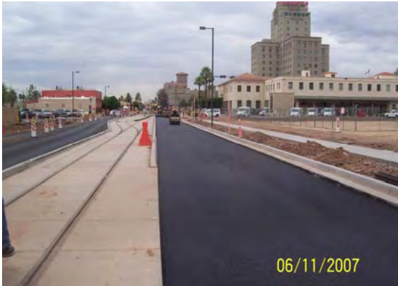
Roadway paving on 1st Avenue
