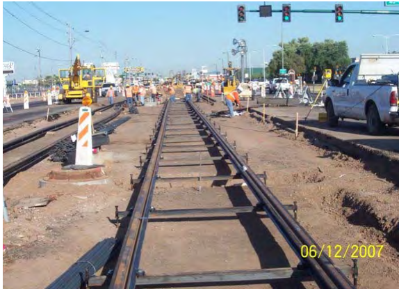
Girder Rail Installation in the Guideway
