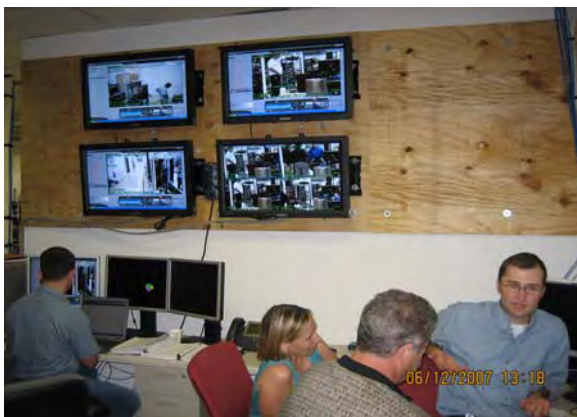
Performing Communications Factory Acceptance Testing of SCADA Hardware
