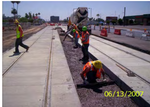
KWC crews placing slurry in the devil Strip
