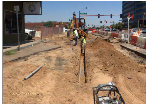
Installation of the 2.5" Conduit For Roadway Lighting
