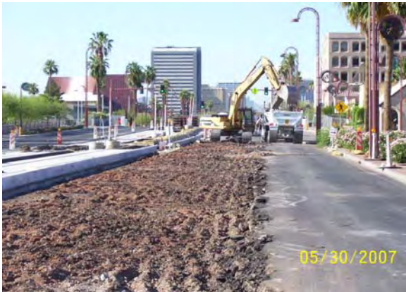
Demolition of Roadway Highland to Cannel Bridge
