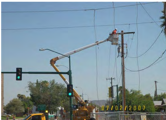
SRP Power removing overhead 12 kV along Camelback Road in LS1
