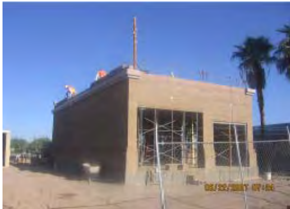
TPSS Number 13 – Final Lift of CMU Walls
