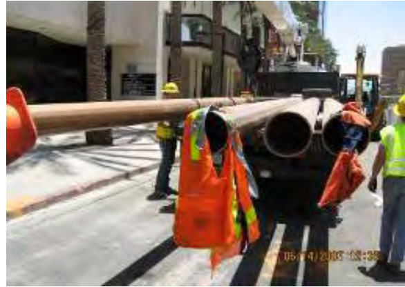
LS3 – Preparing to Install OCS Poles Downtown
