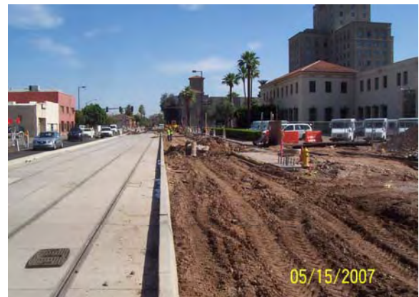
Completed Guideway on 1 st Avenue
