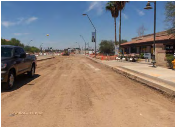
Roadway Work on Apache Boulevard, Milestone D2
