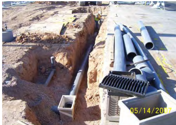
Installation of Track Drainage system
