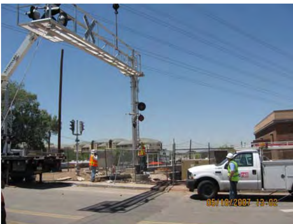
1st/UPRR - Installation of Cantilever
