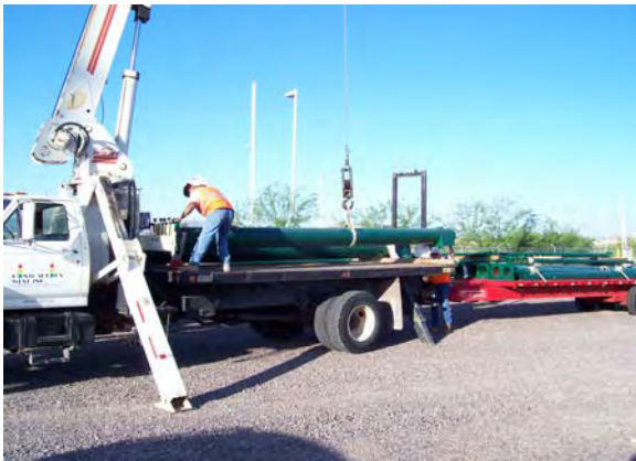
Traffic Signal Poles and Mast Arms being issued to Line Section 3 Contractor
