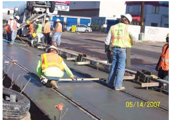
Checking rail alignment during an embedded track concrete placement
