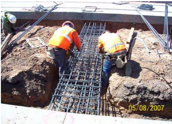
Placing rebar for grade beams at 38 th Street Station
