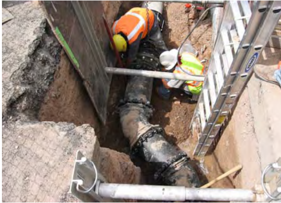
Installing water main north of Virginia
