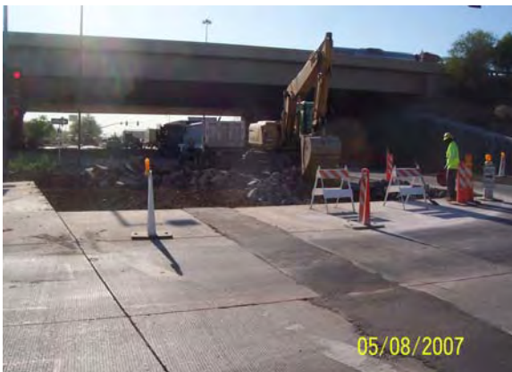
Roadway Paving on 1 st Avenue
