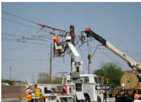
LS4 – Contact Wire Installation (WR 40)
