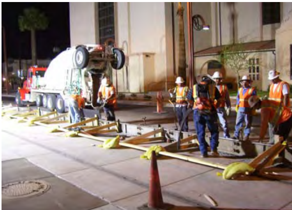
Placing guideway curb North of Highland
