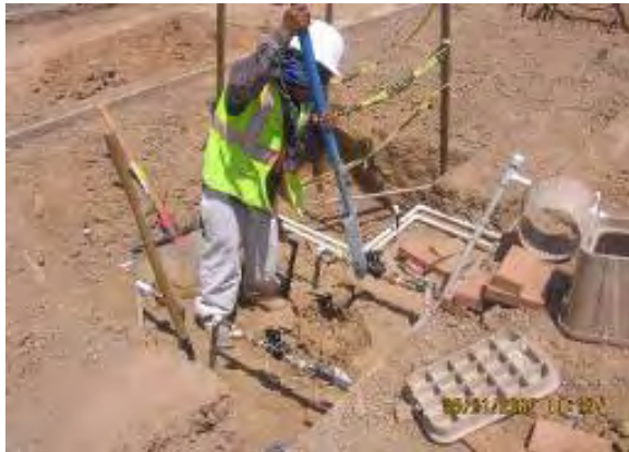
TPSS Number 2 – Installation of Irrigation System
