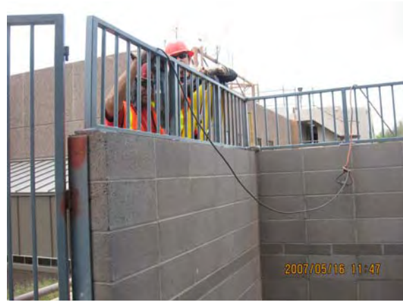
Signal Building Number 6 Installation of Metal Fencing
