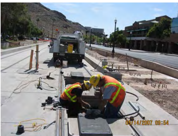
Mill Pocket - Installing Impedance Bonds
