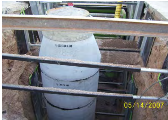
MH Number 14 Off Set Manhole
