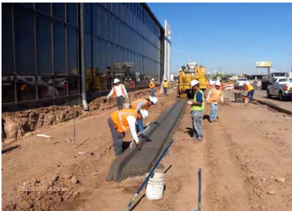
Placing concrete curb/gutter at 28 th Street
