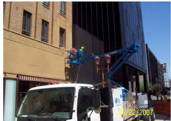
OCS Eyebolt Support Installation at Orpheum Building
