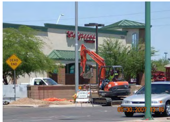
Utility Work in Mesa, Milestone E2
