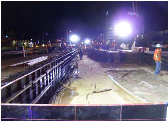
Forming and placing Walls at crossover bathtubs
