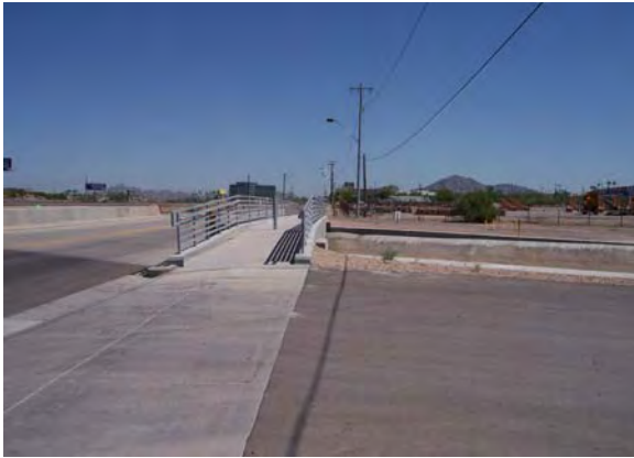
View of the 48 th Street Vehicular and Utility Bridges
