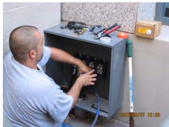
OCC - Terminating Generator Cables
