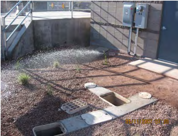
Signal Building Number 4 Completed Irrigation and Landscaping
