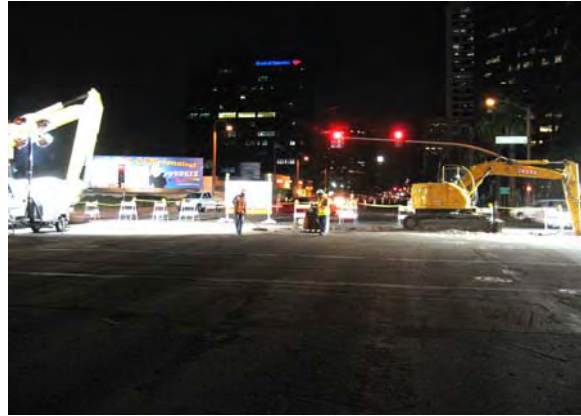
Installing 24" Water main Central/Thomas Intersection Weekend Closure of Central
