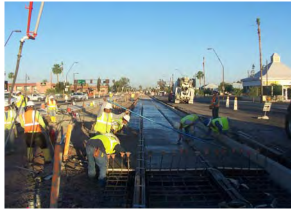
Track Placement at Apache Boulevard, Milestone B2
