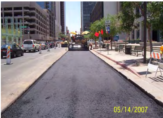
Roadway Paving on 1 st Avenue
