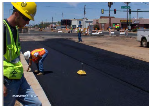
AC Paving - QT check rolling pattern using nuclear gauge
