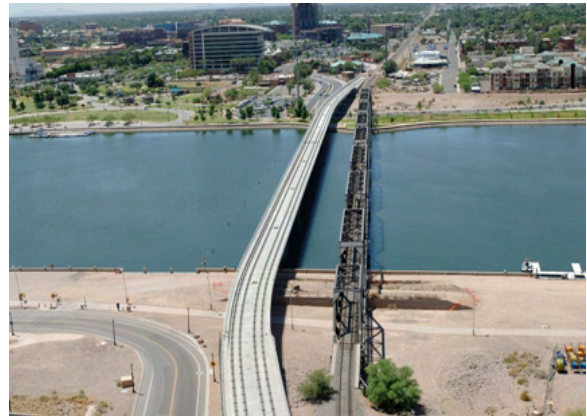
Aerial view of the Tempe Town Lake Bridge with track work complete
