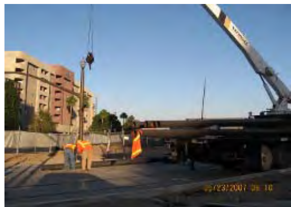
LS5 – Installation of OCS Poles (WR 43 and 44)
