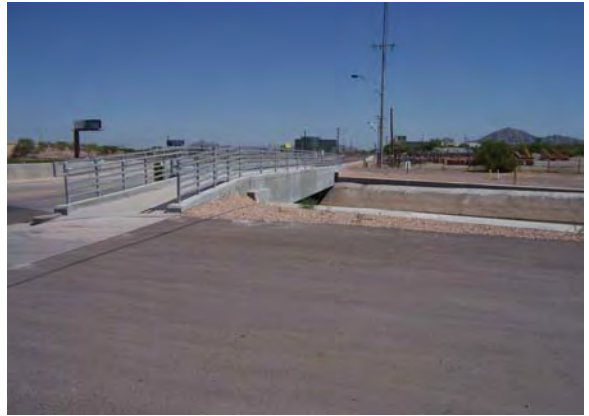
View of the 48 th Street Utility Bridge
