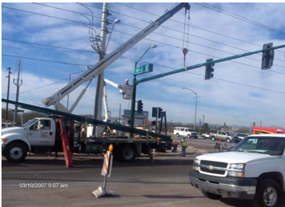
Changing of the signal mast arm at 44 th Street
