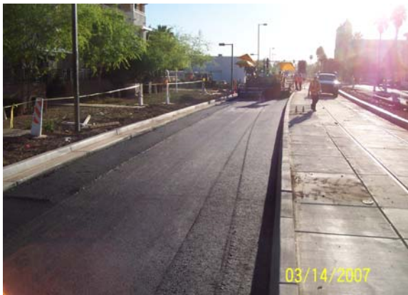
Roadway Paving on Washington
