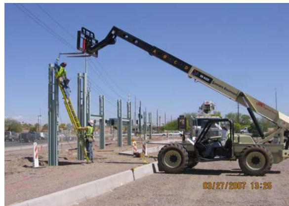
44 th Street and Washington Transit Center Steel
