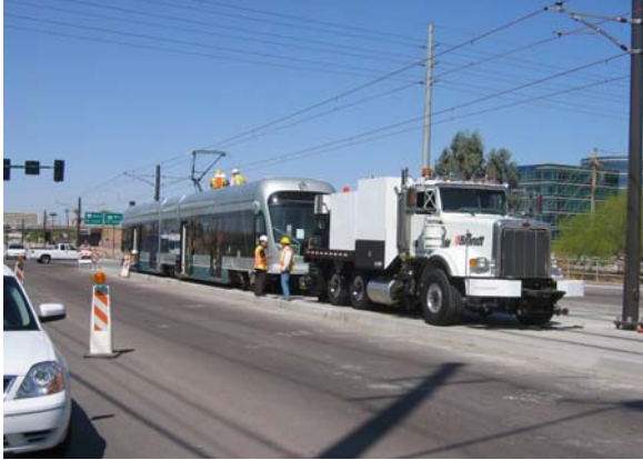
Brandt pulling train on test track during dead wire pull
