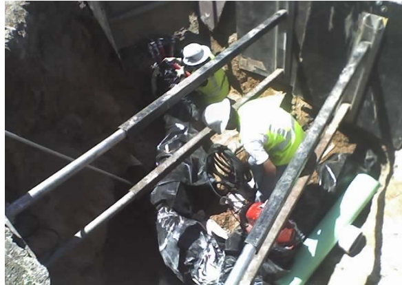
Waterline Work at Main Street and Dobson Road, Milestone E2
