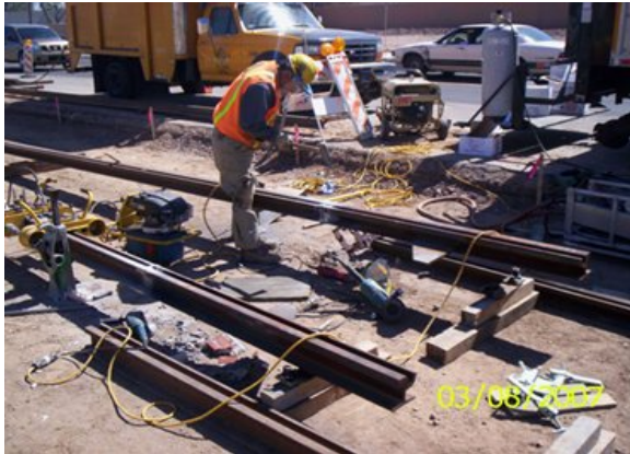
KWC crews performing thermite Welding at R Sta. 1092+02+-, Rt track.
