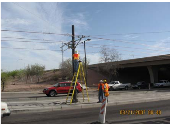
Yard Entrance - Mounting CCTV Camera
