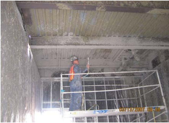
SB No.1 - Applying SFRM
