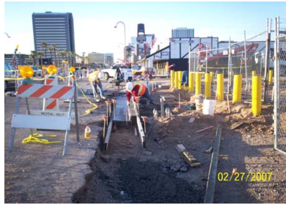
Install Curb and Gutter at Glenrosa
