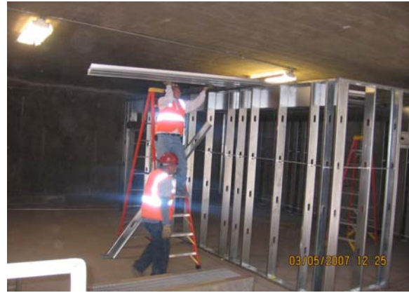
SB No.2 - Installed Interior Roof Decking
