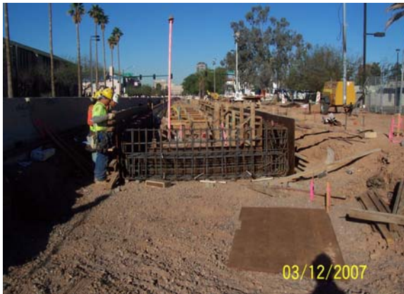
12 th St/Jefferson Station Foundation
