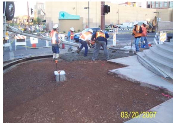
Placing Sidewalk at Jefferson/2 nd Street
