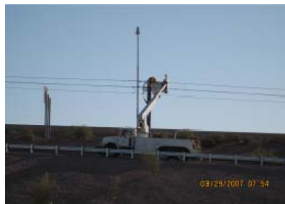
Installation of Lightning Arrestors
