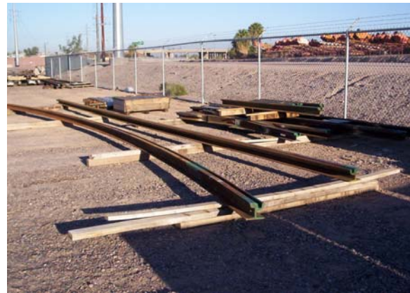
Delivery of 50 meter turnouts (3-12) for Line Section 3.
