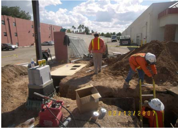
SRP-Power relocation at the Fry's property along Camelback Road in LS1
