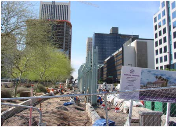
Steel Installation at 1 st Avenue and Van Buren Station
