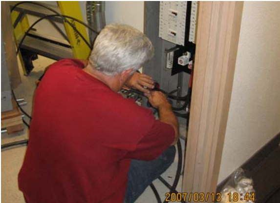
OCC - Performing Electrical Connections
