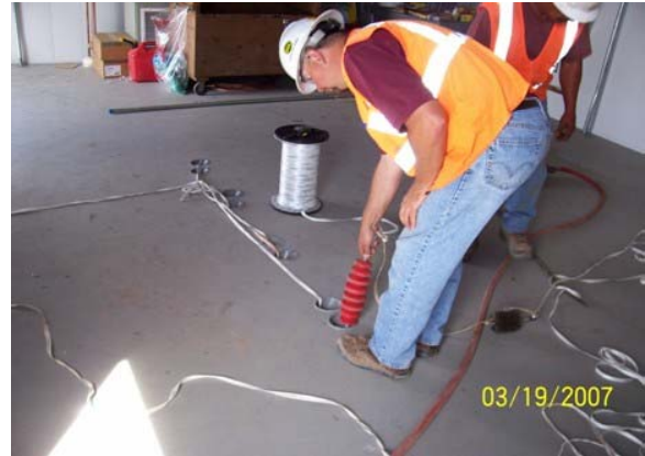
Mandrel of conduits at TPSS No.8
