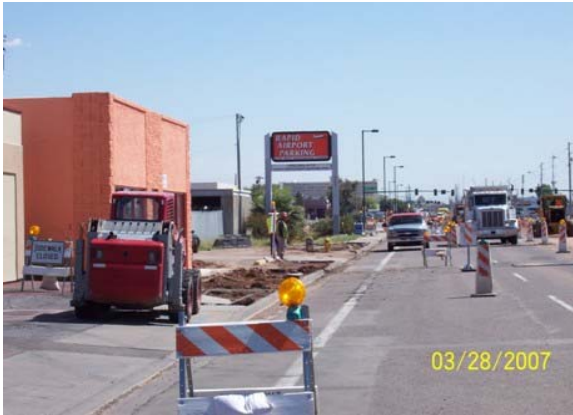
Curb/gutter and sidewalk demolition west of 36 th Street
