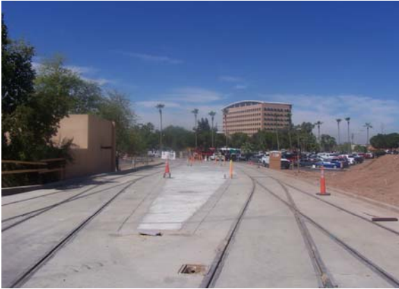
Switch Area at Pocket Track, Milestone A2
