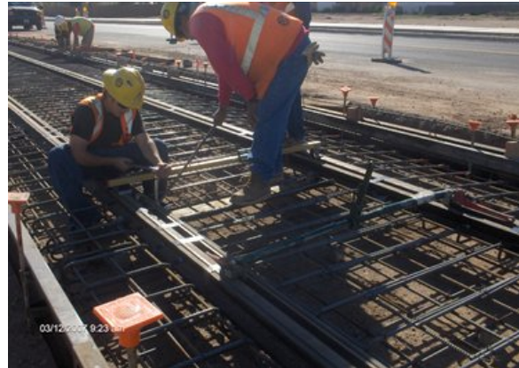
KWC crew making final adjustments to track gauge, RT track 1096+20 to 1094+20.
