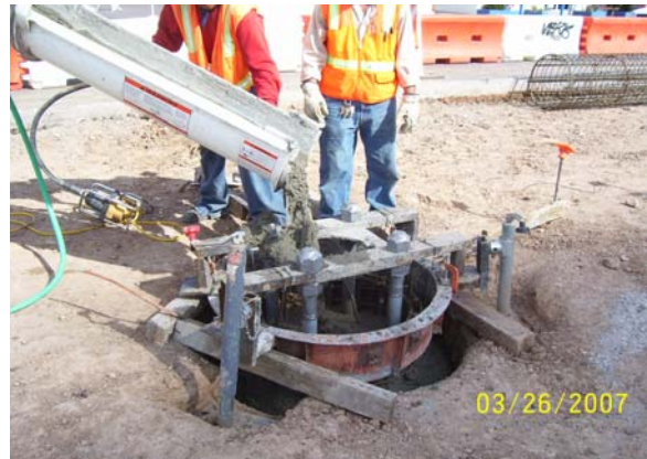
Placing OCS Foundations
