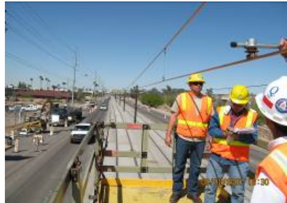
Test Track OCS Inspection
