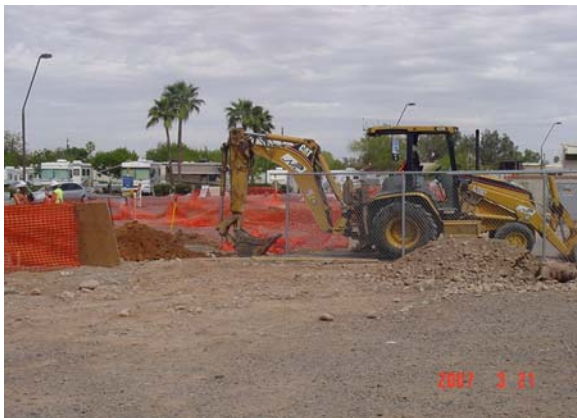
SWG relocation at McClintock and Apache Boulevard in LS5
