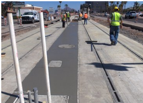
RGG placed concrete for the devil strip 1098+97 to 1101+00.
