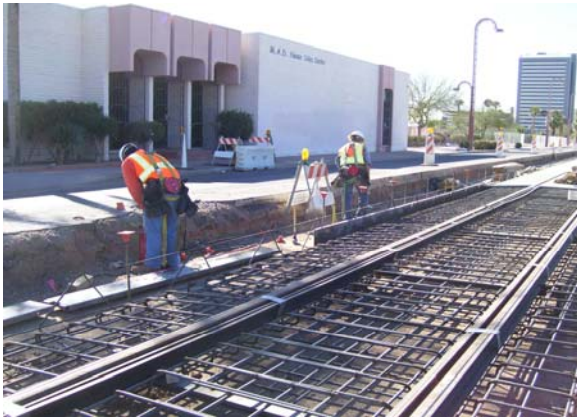
Installing Guideway reinforcing south of Campbell Station
