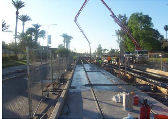
Track Placement at Terrace Road, Milestone B2
