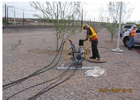
OMC Yard - Installation of Fiber Cable
