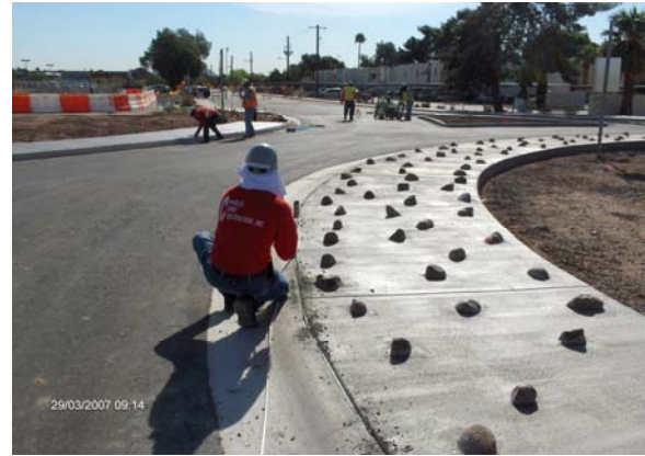
Road construction at 19 th and Montebello Transit Center
