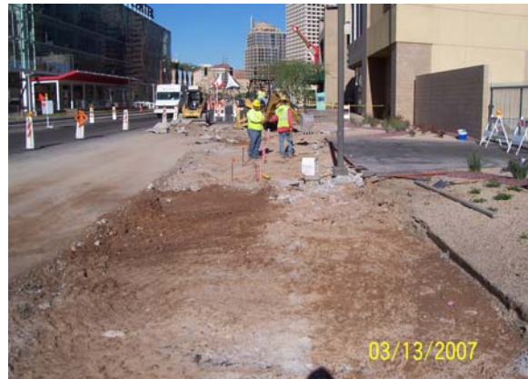
Sidewalk and Driveway Installation on Jefferson
