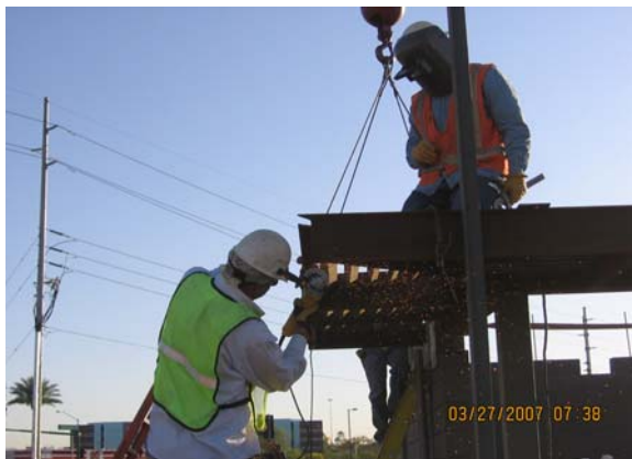
OPF 3 Steel Canopy Installation
