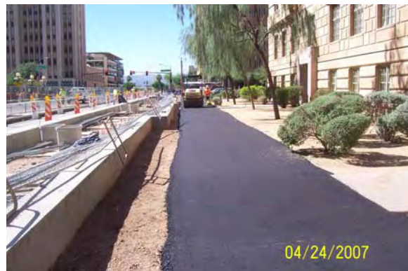
Temporary sidewalk at 1 st Ave and Jefferson Station (County Courthouse)
