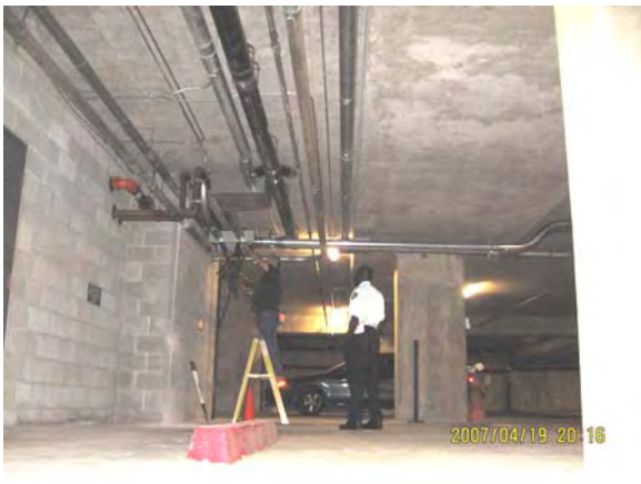
OCC Garage - Pulling Electrical Cables
