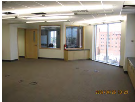
OCC - Operations Room Nearly Complete
