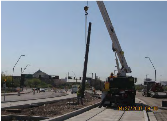
LS4 OCS Pole Installation (WR 39 and 40)
