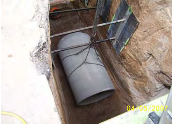
Installing storm drain off set Manhole north of Thomas
