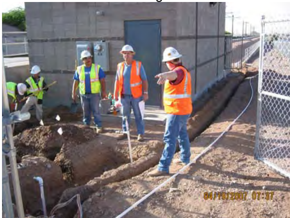
SB number 4 - Installation of Irrigation System
