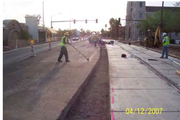
Guideway on Washington
