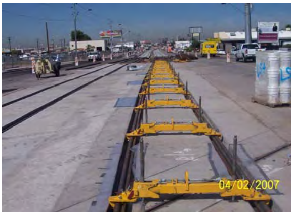
Elastomeric grout placement on the Washington Street Bridge
