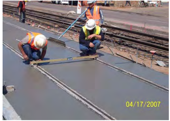
Checking rail gauge alignment for embedded track
