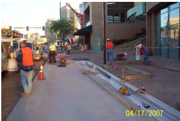
Sidewalk restoration on Collier Center
