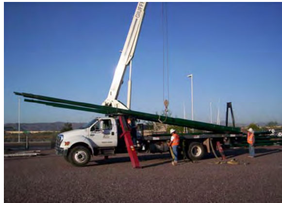
Contractor returning four Mast Arms to Metro Storage Yard for LS4.
