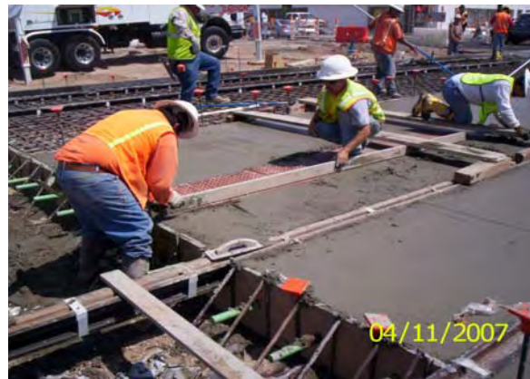
Concrete guideway placement between 17 th and 19 th Avenues
