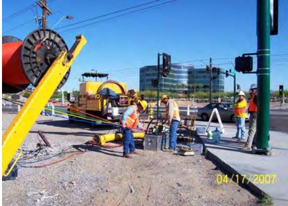
Micro-duct installation at 48 th Street
