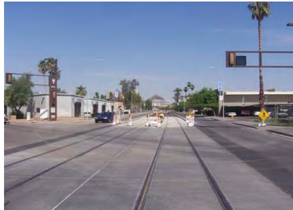
Track Placement at Terrace Road, Milestone B2
