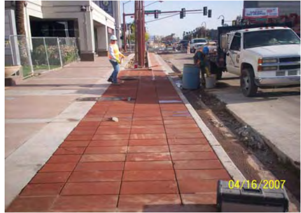
Installing hardscape sandstone pavers at 3800 Central
