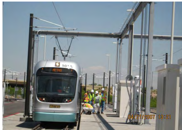
South Yard West Approach Live Wire Test Run
