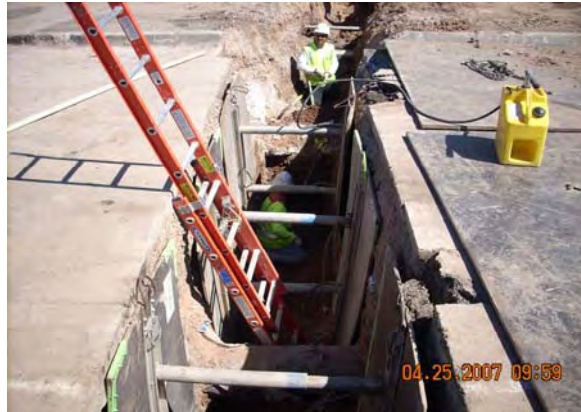
Utility Work in Mesa, Milestone E2
