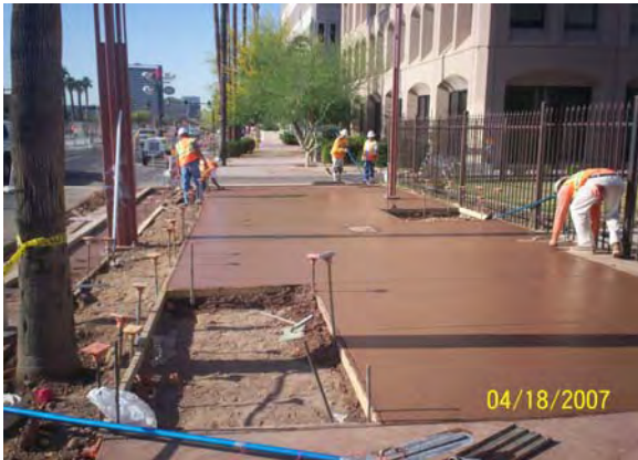
Placing sidewalk North of Campbell
