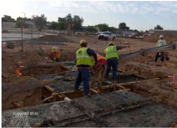
19 th Avenue/Montebello Transit Center Bus Shelter Footing Placement.
