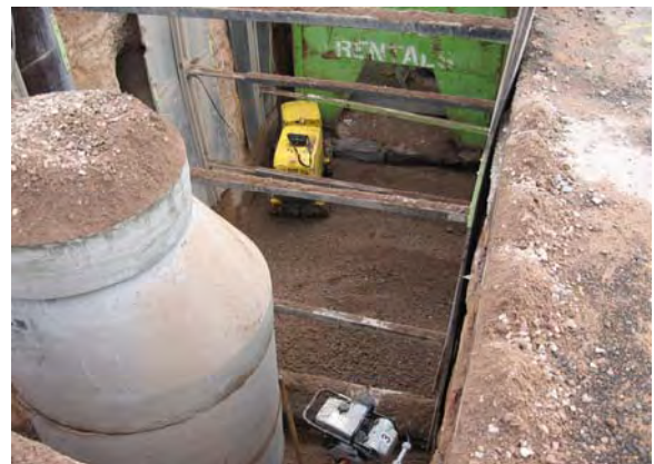
Backfill around off-set manhole NW corner of Thomas
