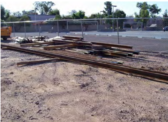
100 Meter Crossover delivered to Contractor's Yard at Line Section 1
