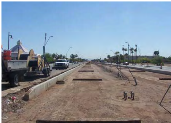
Guideway Work on Apache Boulevard, Milestone B2
