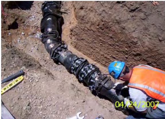
PandCS performing cathodic protection on 8" waterline
