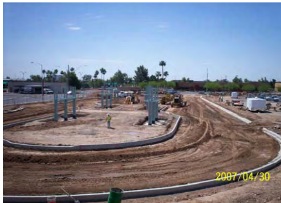
Sycamore / Main Street Transit Center
