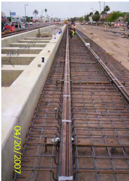
Contractor performing rebar tying on Camelback
