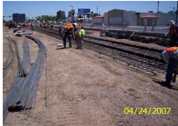
Great Western performing Rebar work on Camelback and 7th Avenue
