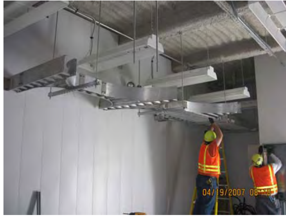
SB number 6 - Installation of Overhead Cable Trays
