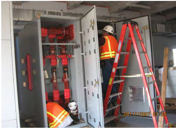
TPSS Equipment Installation TPSS Number 10
