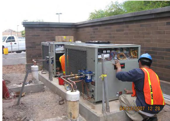
HVAC Installation TPSS Number 11
