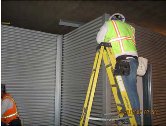
SB number 2 - Installation of Exterior Metal Siding
