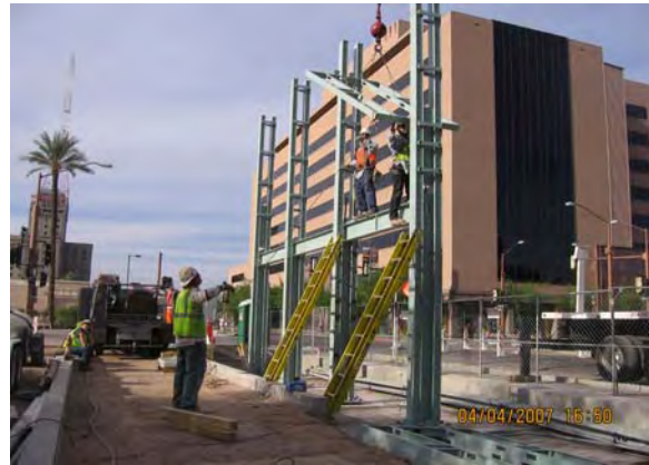
Light Fixture Frame Installation at Central Avenue / Van Buren
