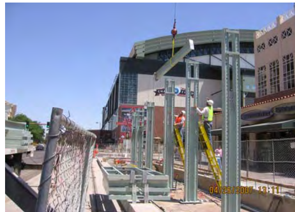
3 rd Street / Jefferson Steel Installation
