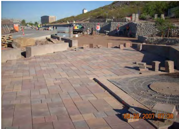
West End of ASU Promenade, Milestone G
