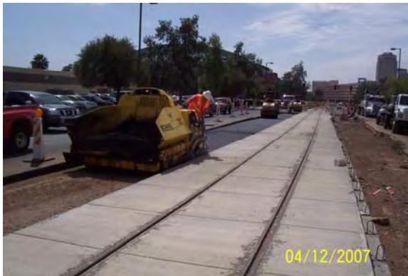
Roadway Paving on Jefferson
