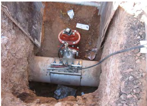
Installing Tapping sleeve onto existing water main
