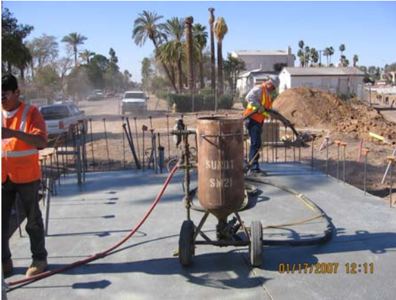
SB No.1 - Sandblasting Slab Concrete Cure
