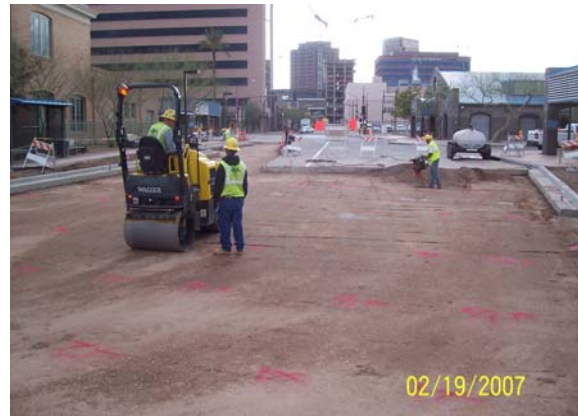
Paving Preparation for Central Station
