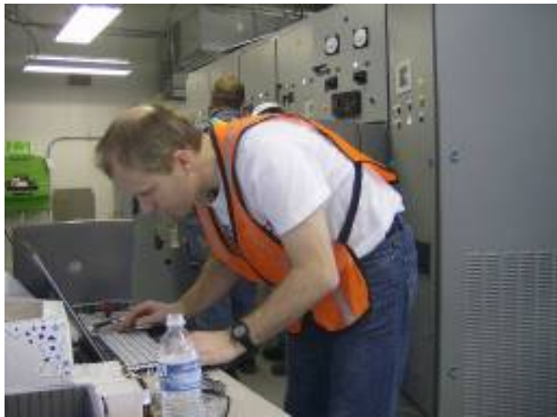
TPSS No. 15 – Testing and Commissioning
