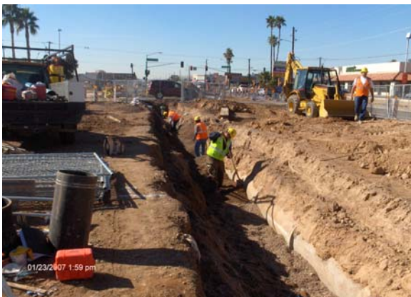
KWC placing the top lift of bedding over the new 12 inch DIP water line between 415+50 and 416+50
