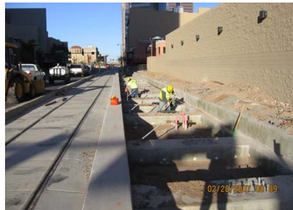
3 rd and Washington Station Underground utility conduit installation
