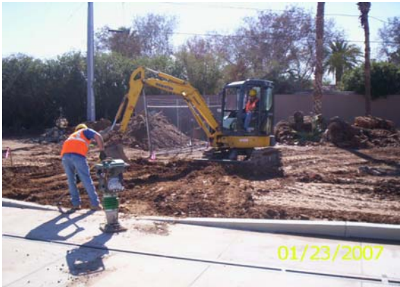
Sidewalk - KWC crews excavating for the Sidewalk at Sta. 471+60+-, Rt. 1087+50+-
