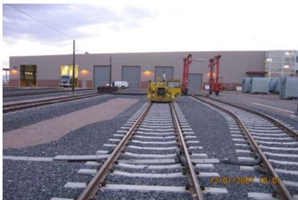
MOE building from the east side
