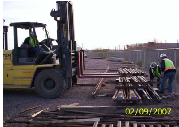
Delivery of two 50 meter turnouts for LS3
