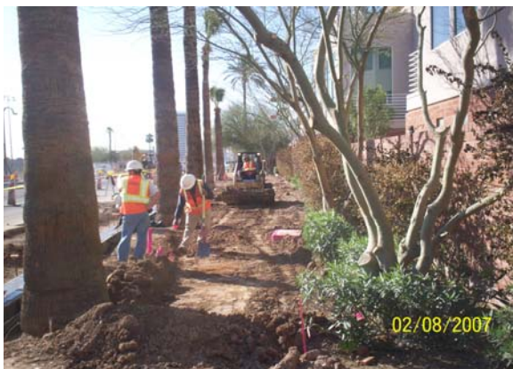
Grading for sidewalk South of Campbell West side of Central
