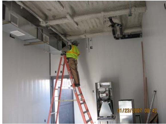
SB No.6 - Installing Mechanical Ductwork
