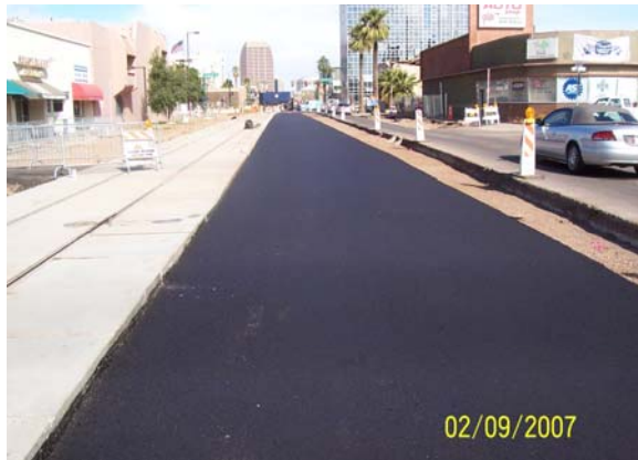
Roadway Paving on Central Avenue
