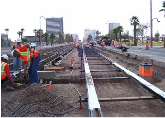
Installing Guideway reinforcing south of Campbell Station
