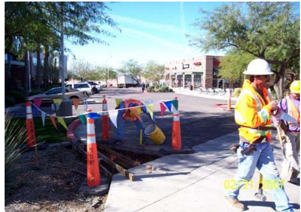
Punchlist work near 48 th Street
