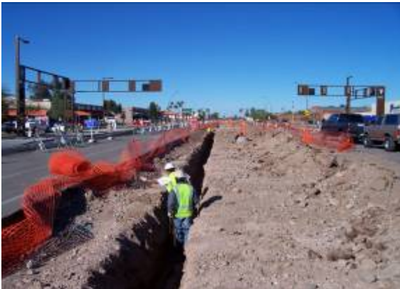
Guideway Ductbank Placement Apache Boulevard
