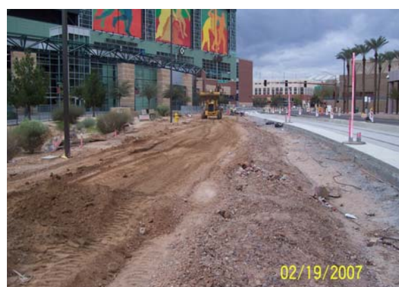
Excavating for Frontage Road on Jefferson at Chase Ball Park
