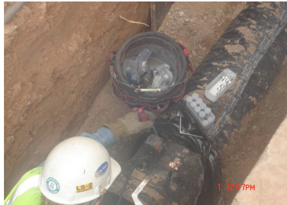
Installing Cathodic Protection jumpers on Water Main
