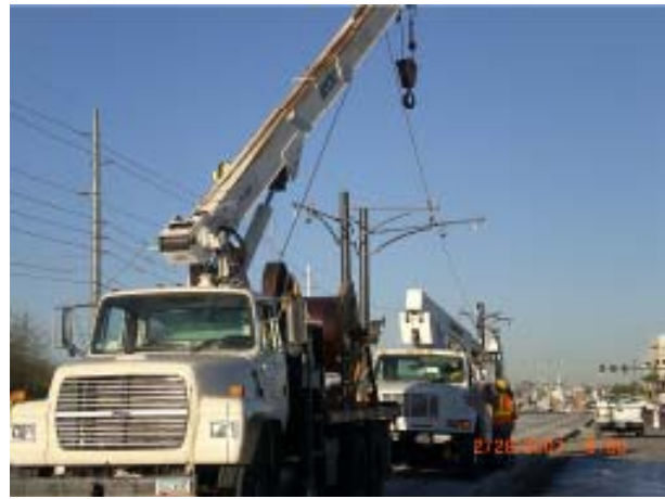
Test Track – Messenger Wire Stringing
