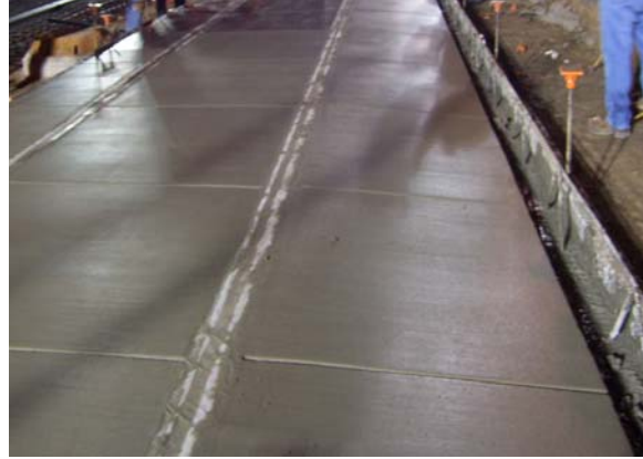
Guideway Placement south of Campbell Station
