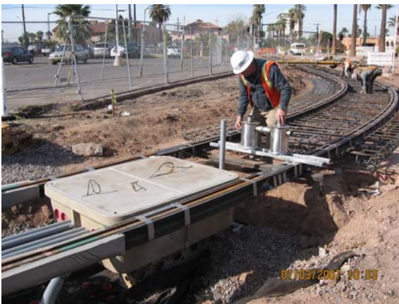
McKinley Loop - Installing Signal Cans
