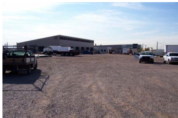
MOW building and the MOW storage yard
