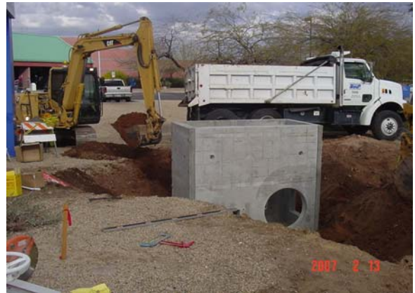
SRP-Irrigation relocation at River and Apache Boulevard. in Line Section 5
