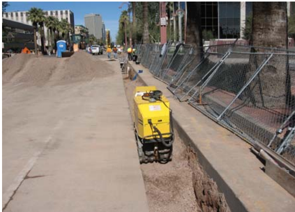
Compacting Water Main Trench south of Palm Lane
