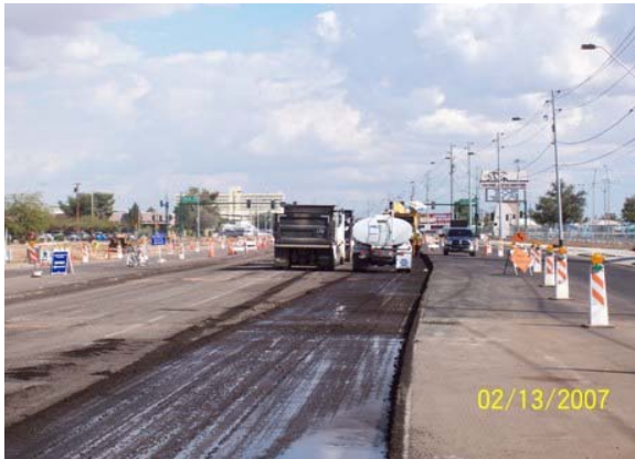
Roadway demolition in preparation for guide-way construction
