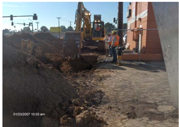
Contractor West trenching for joint trench
