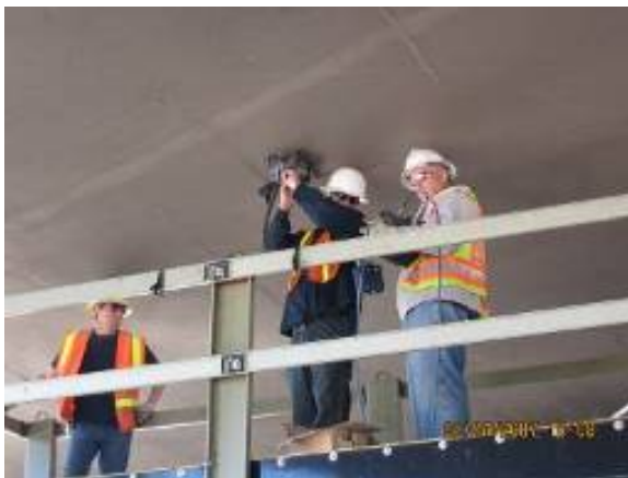
Loop 202 Underbridge Support Installation
