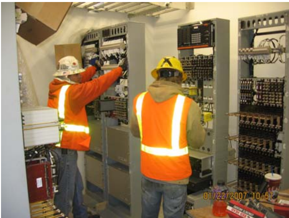
TPSS No.1 - Installing Signal Racks
