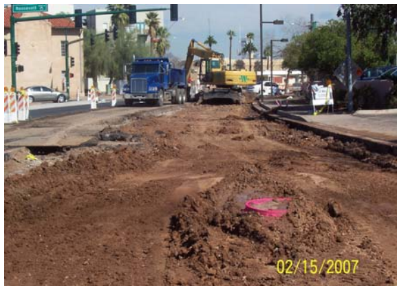
Excavation for Guide Way on 1st Ave
