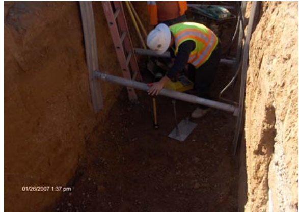
Density Test- ATL performing nuclear density test on SRP Bedding 418+30
