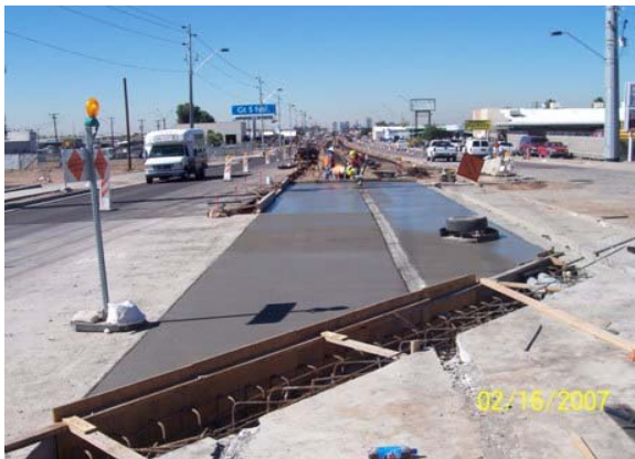
Guide-way placement at the Washington Street Bridge
