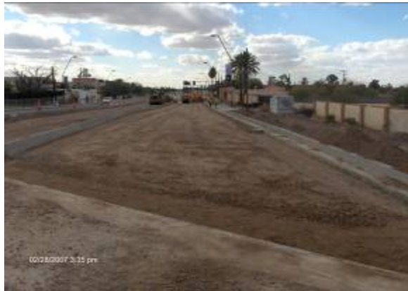
Roadwork at Tempe Canal Bridge
