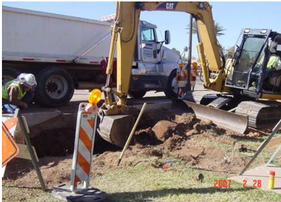
SRP-Irrigation relocation at Smith and Apache Boulevard in Line Section 5
