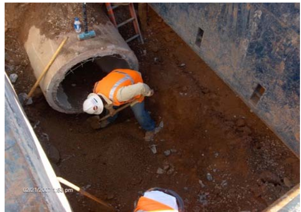
Offset manhole installation
