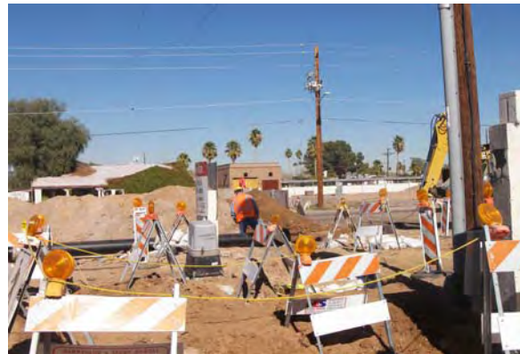
SRP-Power relocation on 16 th Avenue and Camelback Road in Line Section 1
