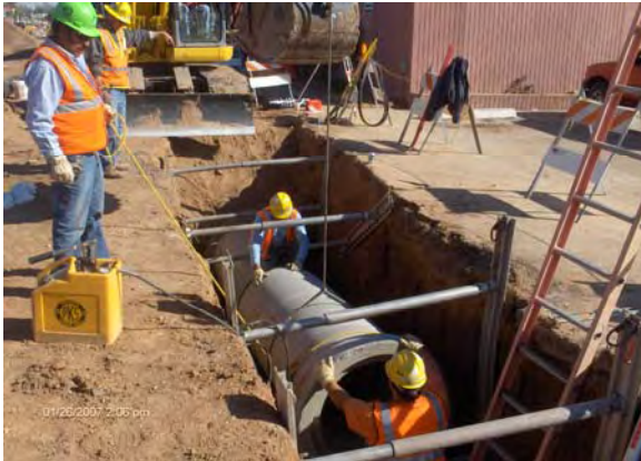
SRP 30 Inch Irrigation- KWC installing new SRP 30 Inch at 418+30
