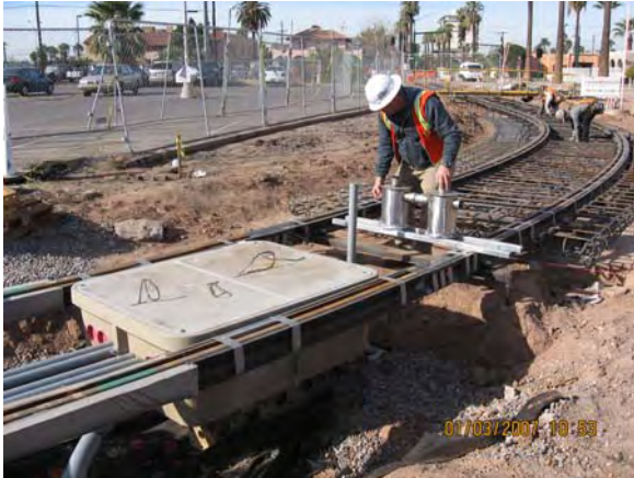
McKinley Loop - Installing Signal Cans
