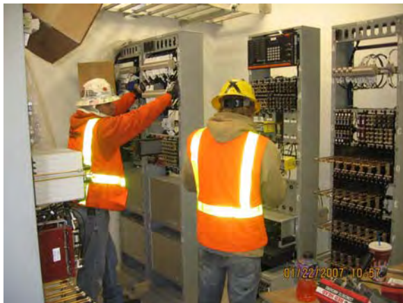
TPSS #1 - Installing Signal Racks
