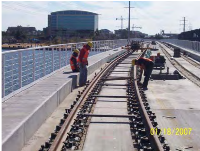
Direct fixation plinth construction on the Town Lake Bridge
