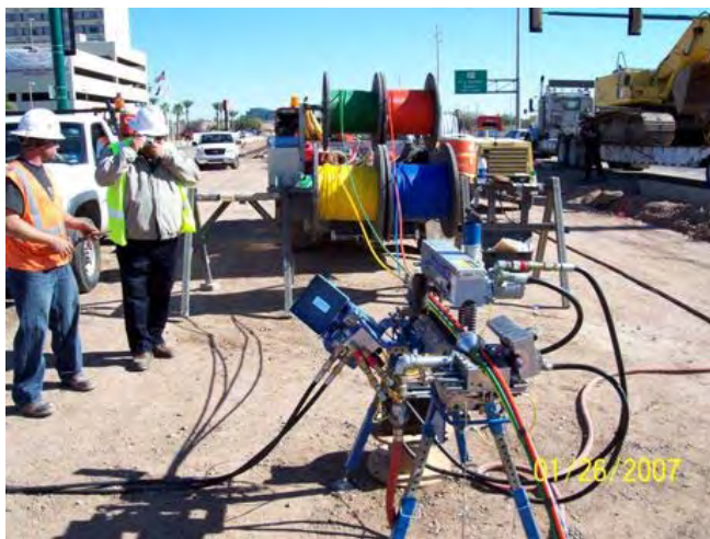
Micro-duct installation across the Washington Street Bridge at the Grand Canal
