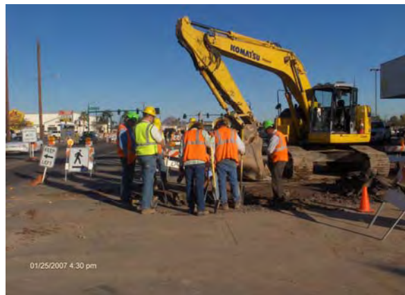
KWC Staff Working on locating water 2 inch water service corp stop to shut water off for the service that was hit by KWC removal crew at 396+80 Camelback
