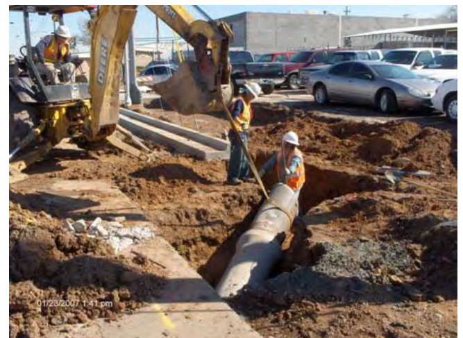
Storm drain catch basin installation at 34 th Street
