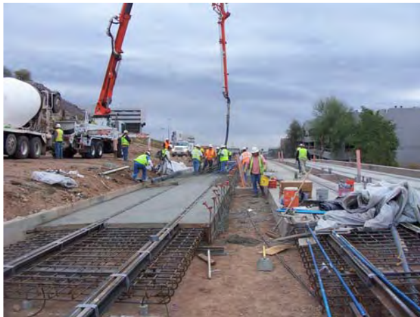
Track Placement, Pocket Track
