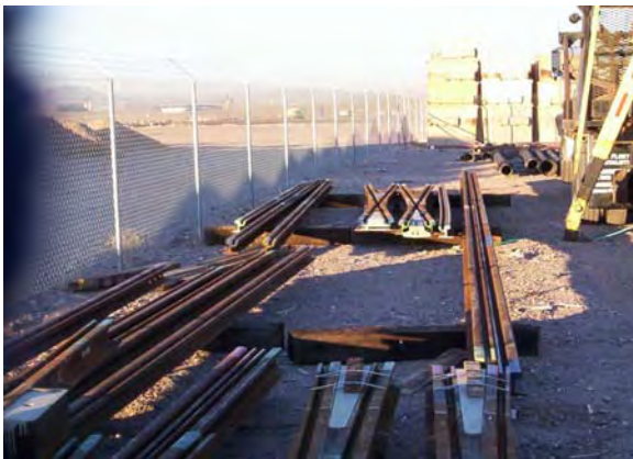
Delivery of a Left Hand Single Crossover 2-3 & 2-4 for Line Section 2
