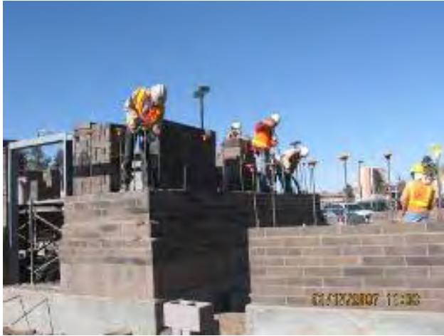
TPSS No. 11 – 3 rd Lift of CMU
