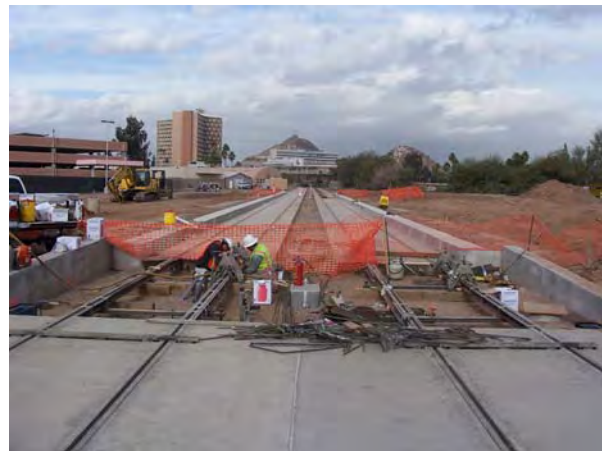
Trackway and Station Foundation—Rural Road
