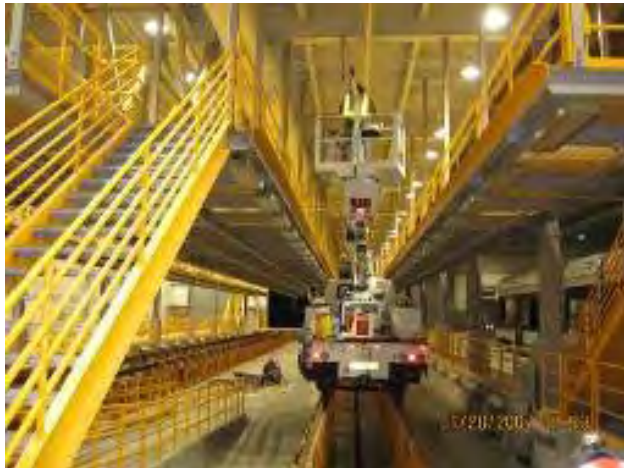
MOE Shop Tracks – OCS Installation
