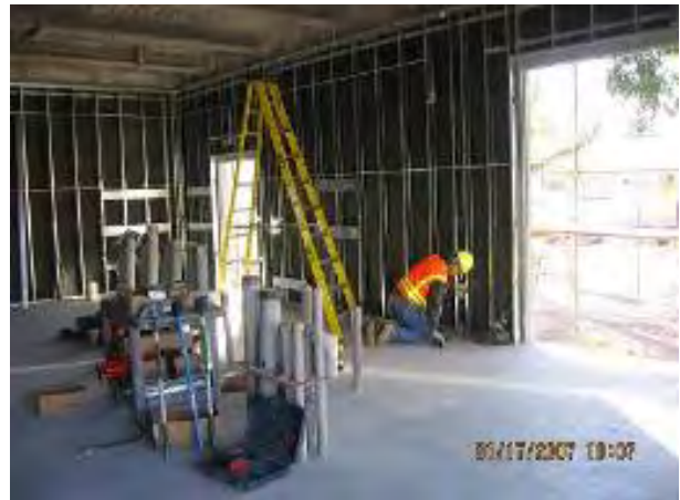
TPSS No. 5 – Metal Stud Framing Installation
