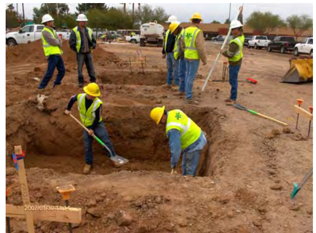
Excavation for bus shelters at Sycamore / Main Street Transit Center
