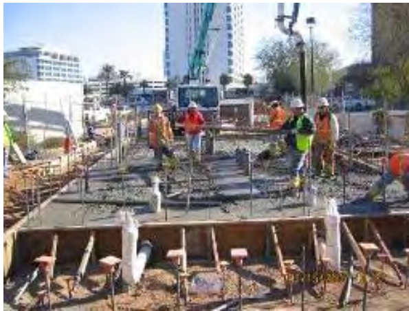
TPSS No. 4 – Slab Concrete Placement
