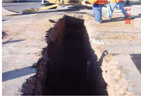
SRP relocating underground 12 kV on Apache Blvd. in Line Section 5
