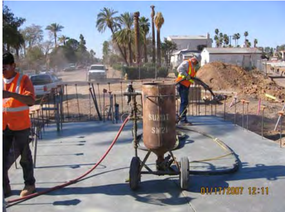
SB #1 - Sandblasting Slab Concrete Cure
