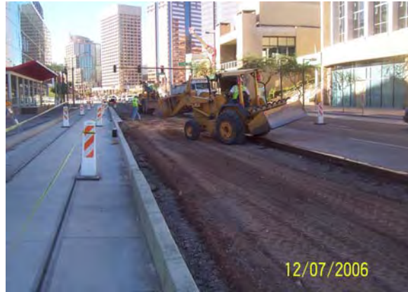
Pavement Sub Grade Preparation on Jefferson
