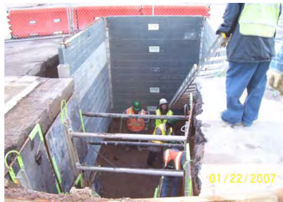
Excavation for 24" water main at Osborn
