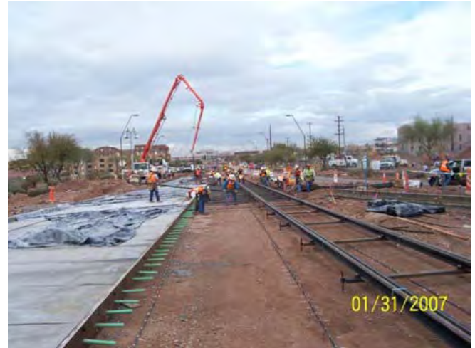
Guide-way construction across Washington Street near Lake View Drive
