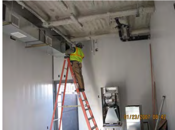
SB #6 - Installing Mechanical Ductwork
