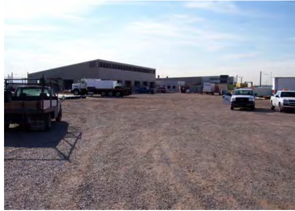
MOW building and the MOW storage yard
