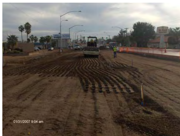
Roadwork at Tempe Canal Bridge
