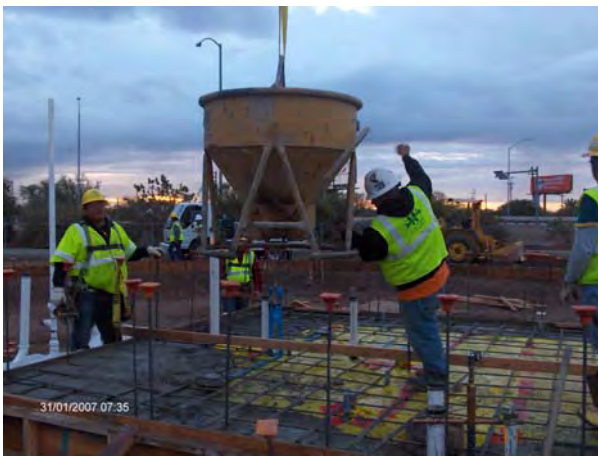
OPF-3 Foundation Slab Placement at 44 th Street / Washington Transit Center
