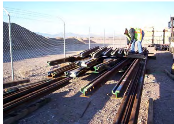
Delivery of a Left Hand Single Crossover 2-3 & 2-4 for Line Section 2
