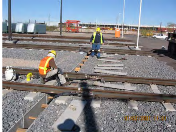
OMC Yard - Installing Crossbonds
