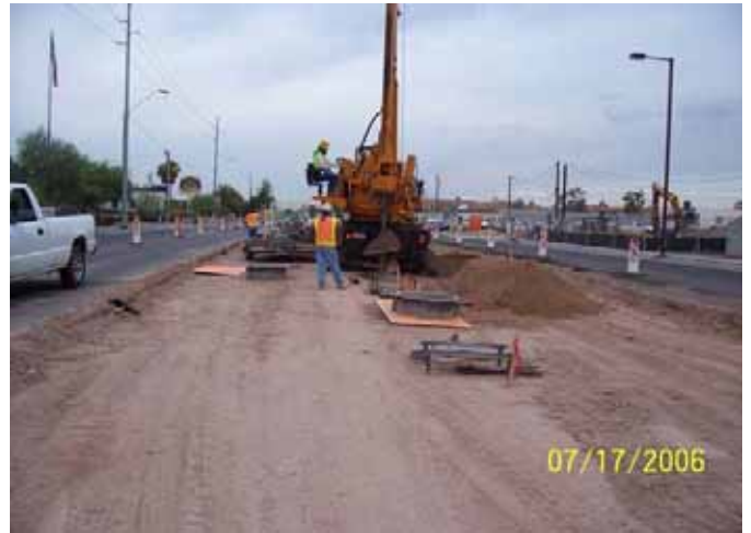
OCS foundation excavation
