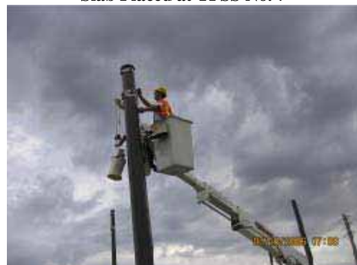
Installation of Pole Bands - North MSF Yard
