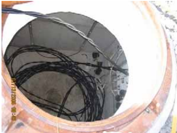
MSF Yard - Pulling Signal Cable
