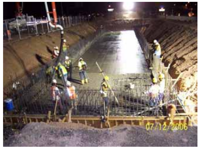
Placement of the APM foundation west of 44 th Street
