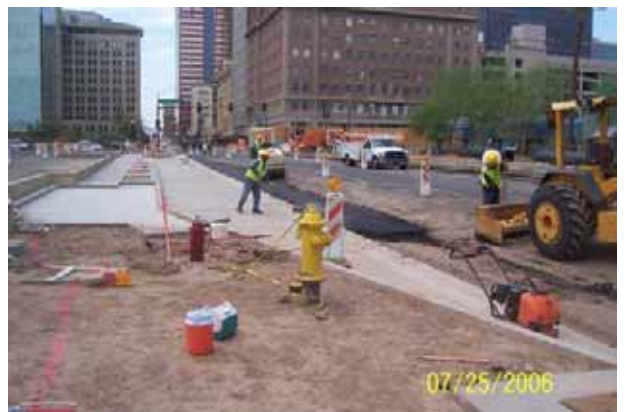
Central Bus Way pavement between Van Buren and Polk
