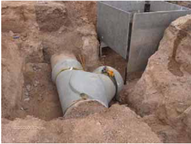
Offset storm drain manhole construction
