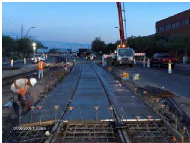
Guideway placement east of 56 th Street
