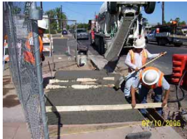
Sidewalk Pour near Central High School.
