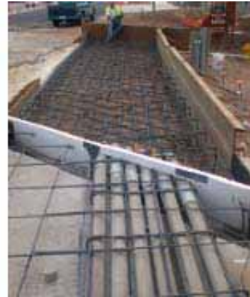
Roadway Work at Tempe Canal Bridge
