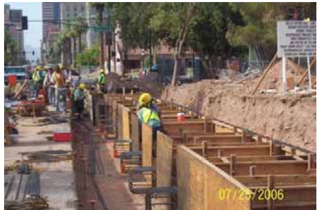
Roosevelt/Central Station Foundation Formwork
