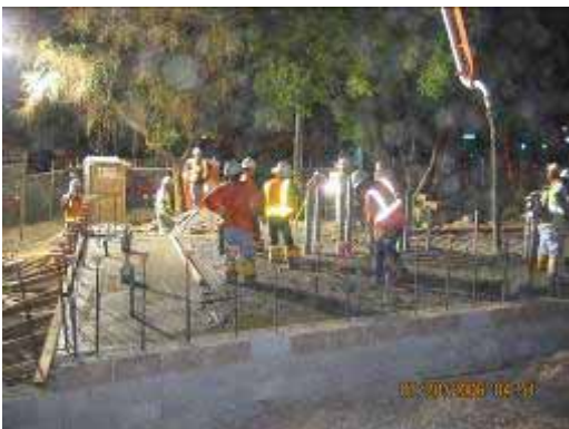
Placement of Slab at TPSS No. 5
