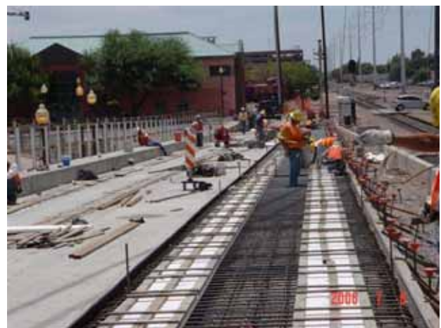
Right Track Slab at South Approach
