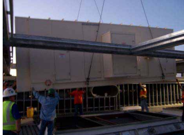
Setting HVAC equipment on MOE lower roof
