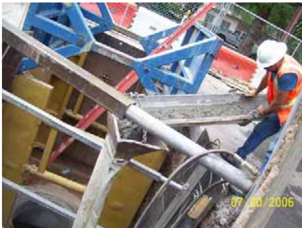
Concrete being placed around collar at Manhole 21.
