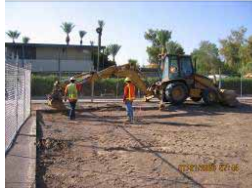
Initial Clearing and Grubbing at TPSS No. 11
