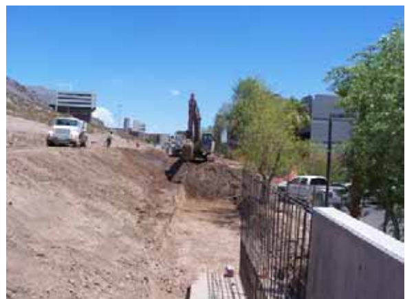
Continuation of Work at Retaining Wall 1
