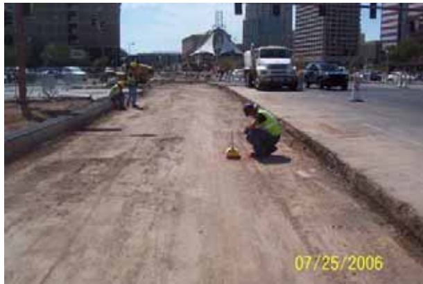
Guideway Subgrade Preparation
