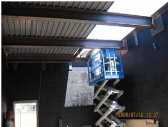
SB No. 3 - Installation of Roof Decking
