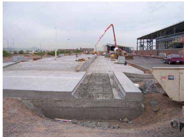
Service and cleaning platform looking west
