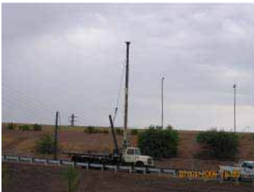
Installation of OCS Poles – North MSF Yard
