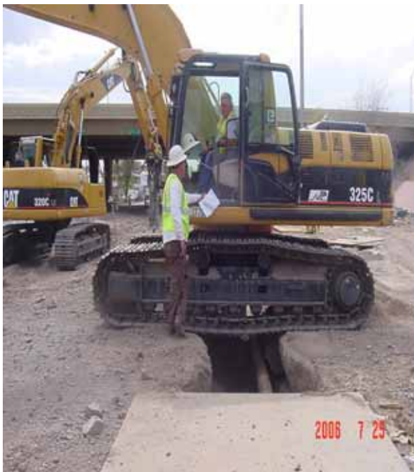
SWG relocation 8-inch High Pressure Gas main at Washington Street and SR 202 in Line Section 4
