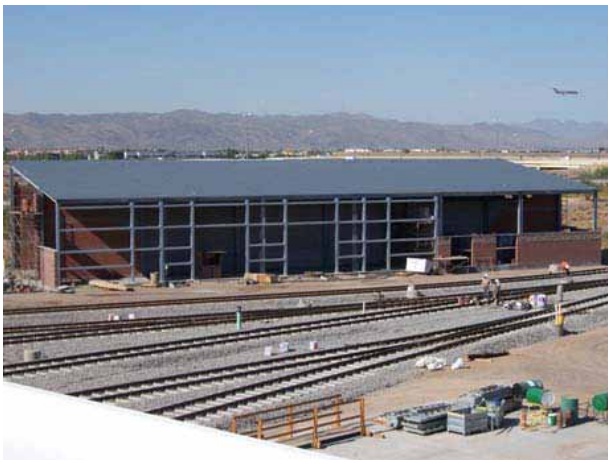
View of the LRV building from northeast
