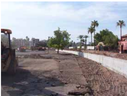
Retaining Wall 5, Ash to First Street
