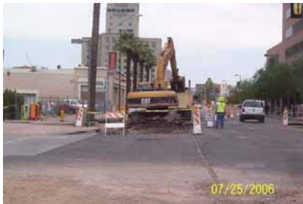
Demolition of Central pavement between Polk and Fillmore
