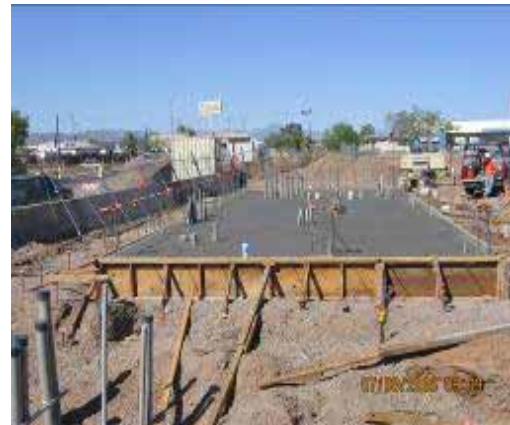
Slab Placed at TPSS No. 7
