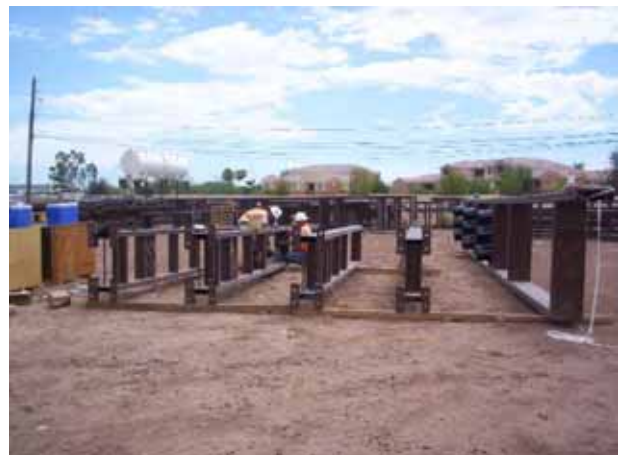
Traffic Signal Poles being assembled at the LS5 Apache Blvd Storage Yard
