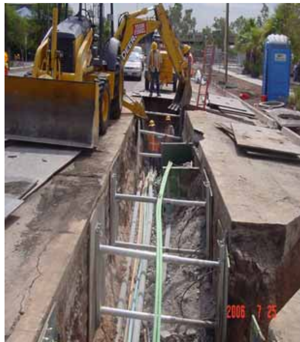
Level 3 relocating on Washington Street in Line Section 3
