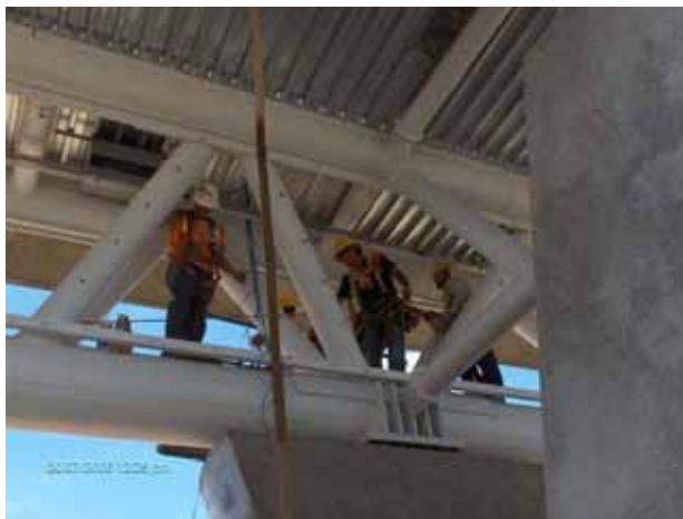
Electricians Installing Luminaires
