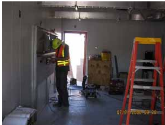
SB No. 5 - Installation of Signal Equipment
