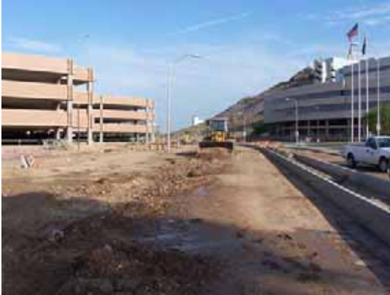
Roadway Work at Veterans' Way
