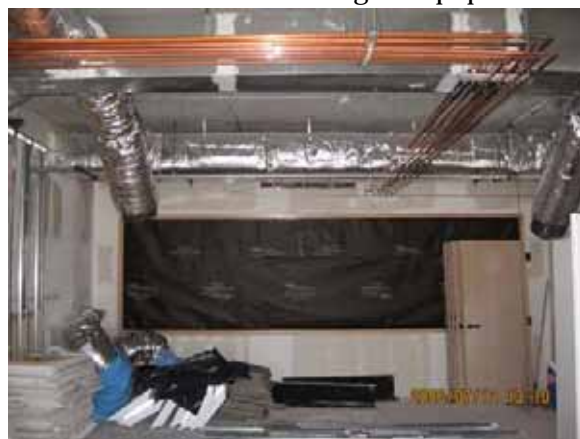
OCC - Continuing Mechanical Installation
