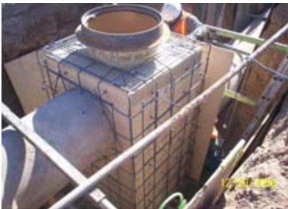
Forming SRP Manhole
