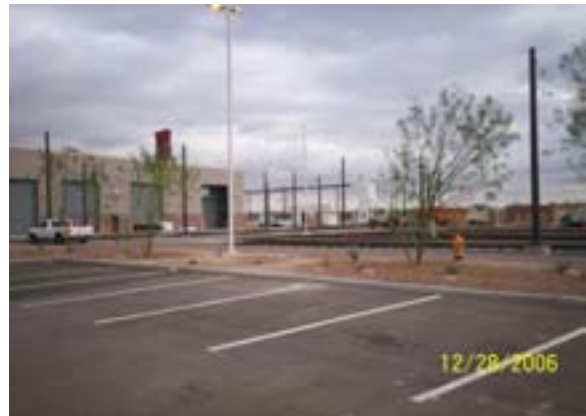
SW MOE and Inspection Platform
