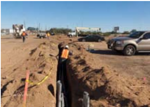
Electrical conduit installation at 44 th Street and Washington Transit Center
