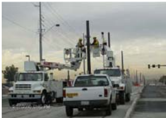
Installation of Cantilever Arms for Test Track
