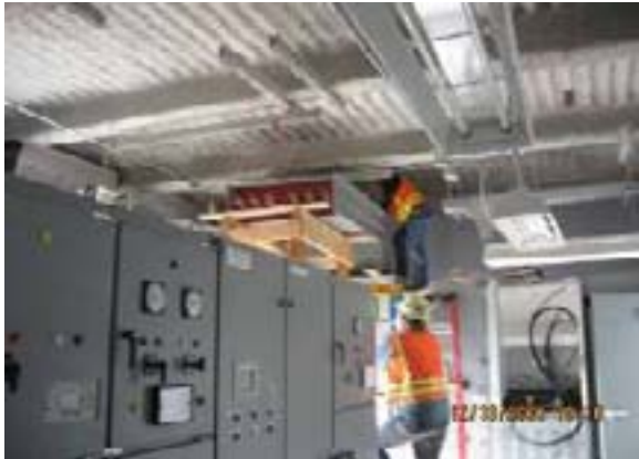
Bus Duct Installation at TPSS No. 15
