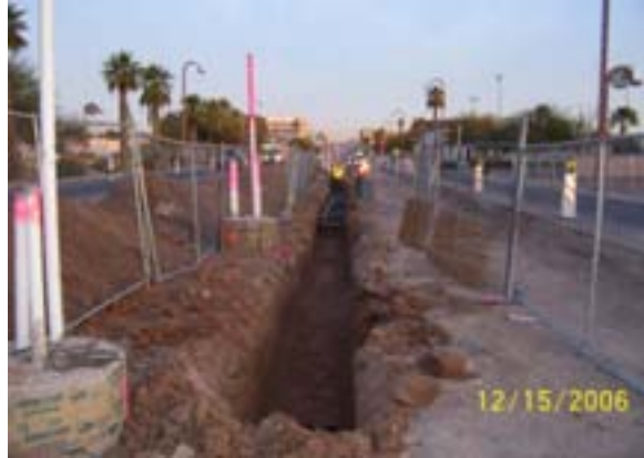
Installing Backbone Ductbank
