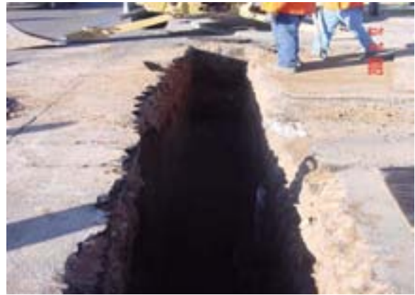
SRP relocating underground 12 kV on Apache Blvd. in Line Section 5
