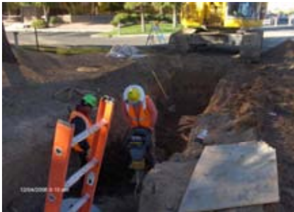
KWC compacting bedding for 24" water line south of Camelback.
