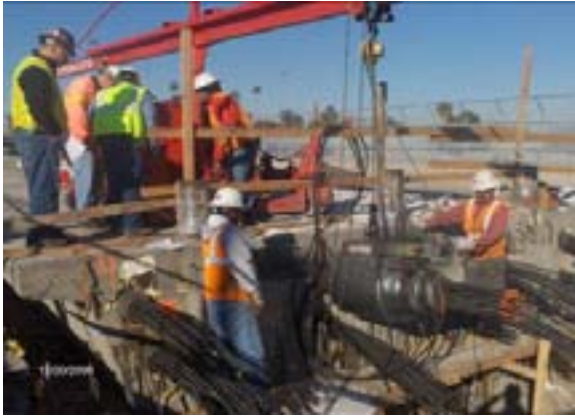
101 Freeway Bridge, Post-Tensioning New Center Girder
