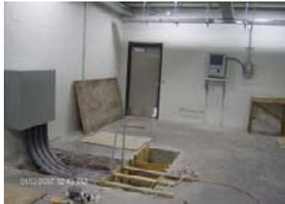
TPSS No. 16 (Shop TPSS)
