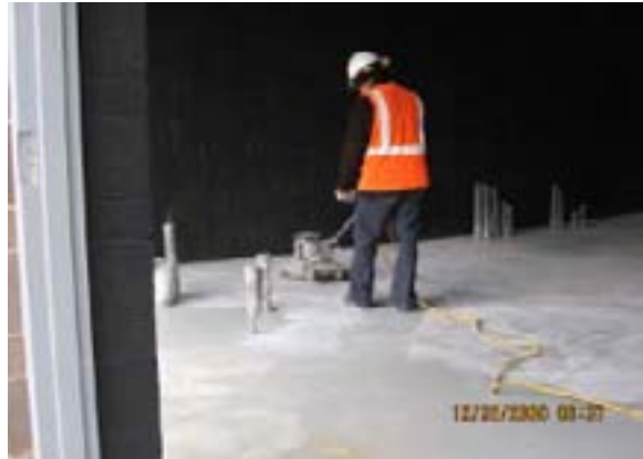
Dielectric Floor Application at TPSS No. 5
