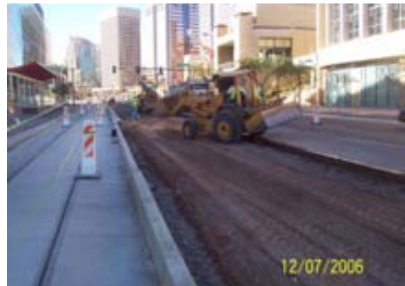
Pavement Sub Grade Preparation on Jefferson
