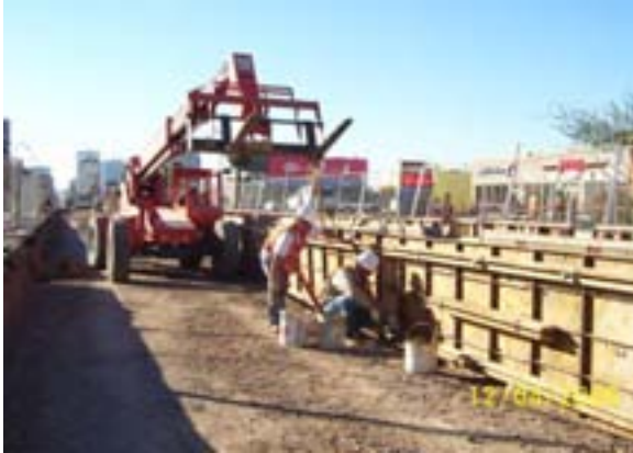
Forming Campbell Station
