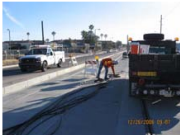
Yard Entrance - Pulling Signal Cable
