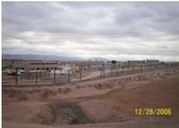
Site Overview from Yard Lead
