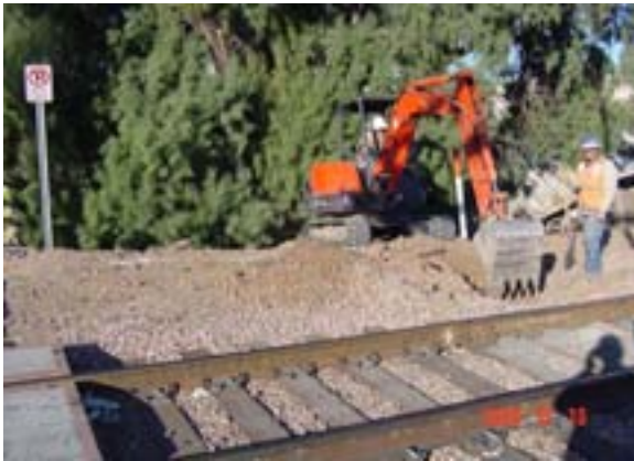
UPRR relocation at 1 st Street and Ash Line Section 5
