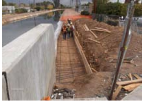
Placing Gravity Wall at Tempe Canal Bridge
