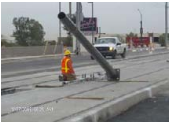
Pole Installation for the Test Track
