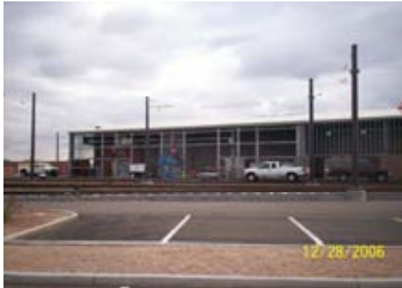
LRV Wash Facility
