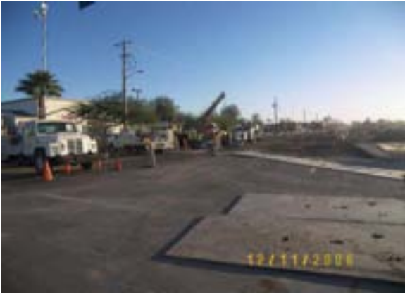
SRP-Power relocation on Camelback Road in Line Section 1
