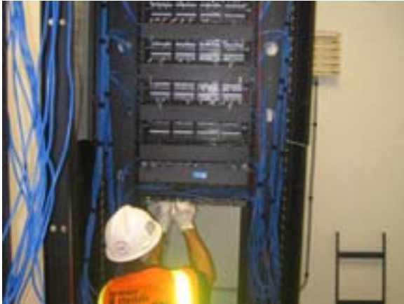
MSF MOE - Installing Telephone System
