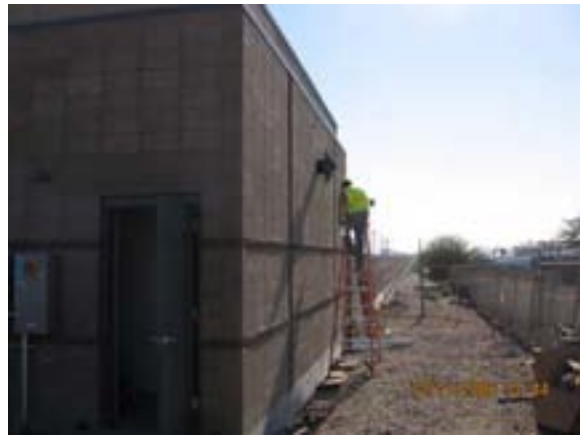
SB No. 4 - Installing Exhaust Ventilation
