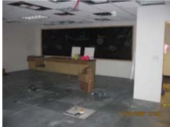
OCC - Completing Flooring and Ceiling
