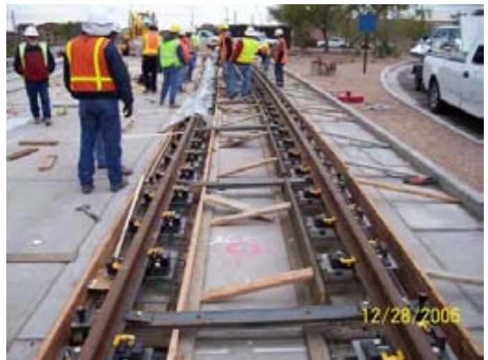
DF fastener/plinth installation at Tempe Town Lake Bridge
