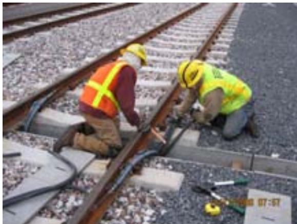
MSF Yard - Installing Crossbond Cables
