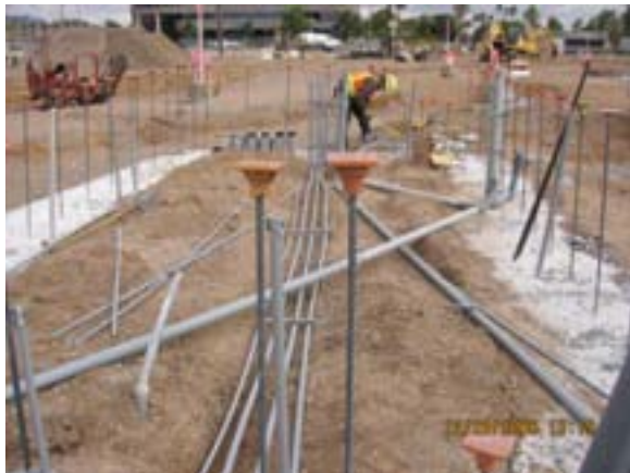
SB No. 1 - Installation of Underslab Conduits
