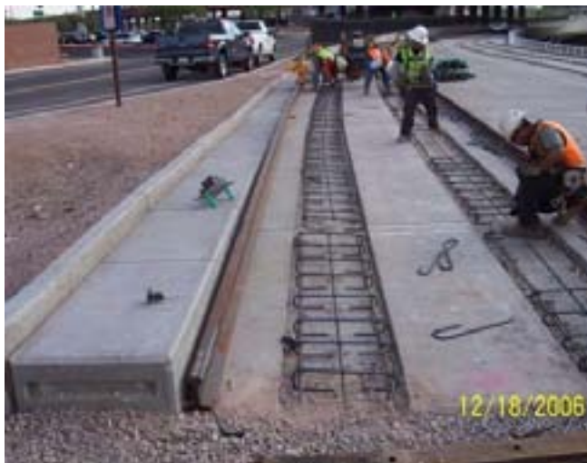
Installing plinth reinforcement at the Tempe Town Lake Bridge
