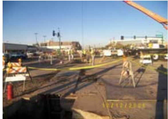
SWG relocation on 19 th Avenue and Camelback Road in Line Section 1
