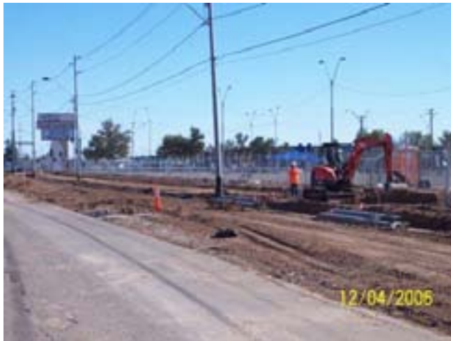
Grading sub-grade prior to sidewalk installation
