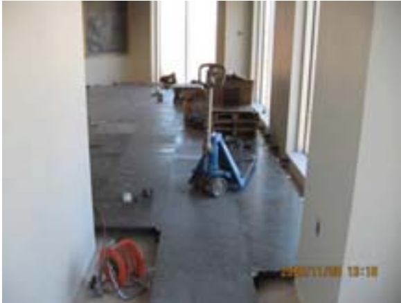
OCC - Installed Access Flooring System
