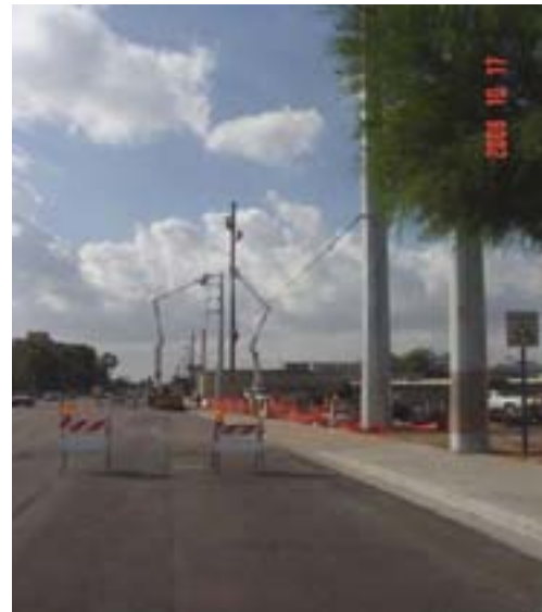
SRP relocating 69 kV at Rural and Tyler in Line Section 5
