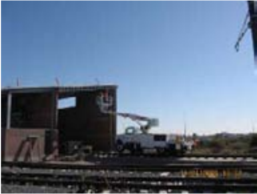
Cantilever Installations in the South Yard
