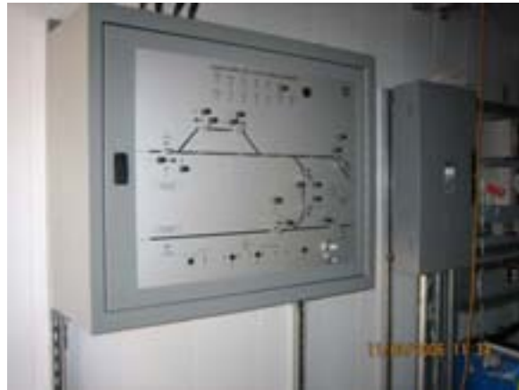
SB No. 3 - Installed McKinley LCP
