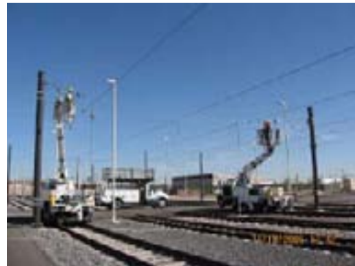
Re-Adjustment of Headspans in the North Yard
