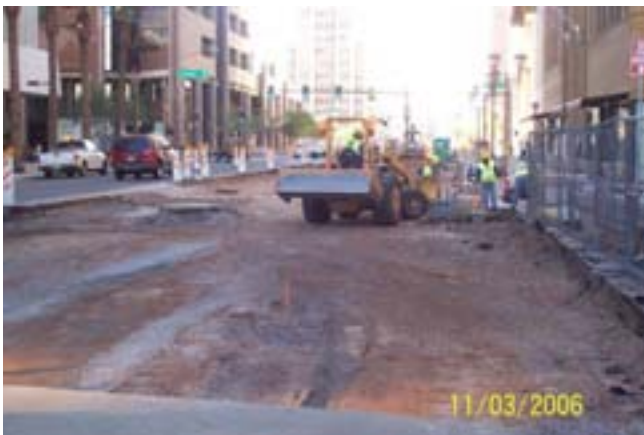
Guideway Excavation at 1 st Ave and Adams
