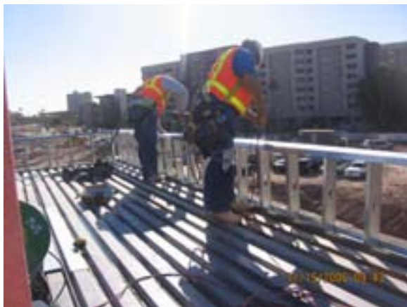
SB No. 6 - Installing Parapet Roof Frame
