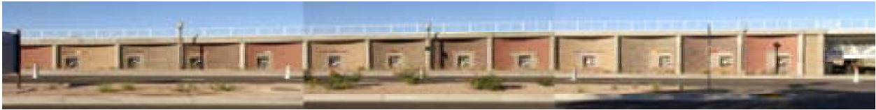
Southeast Retaining Wall with Artist’s Plaques
