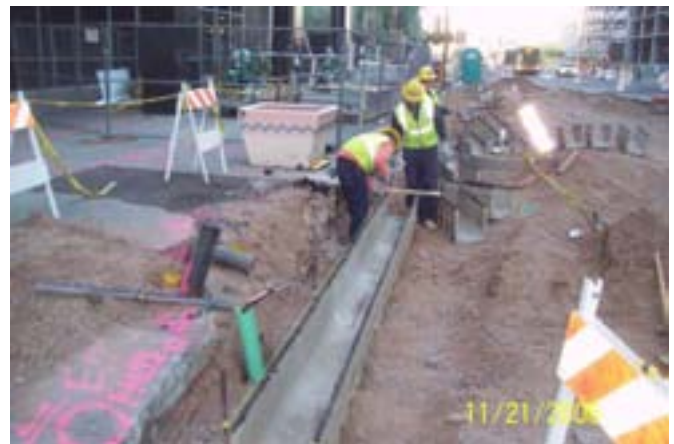
Trench Drain Installation at 1 st Ave
