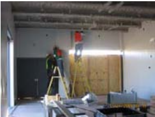
Metal Panel Installation at TPSS No. 1
