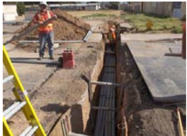
11-14-06 SRPP Joint Trench-Contractors West Installing Conduits In The Lateral Trench At 346+18
