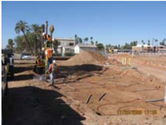
SB No. 1 - Installation of Ground Grid System
