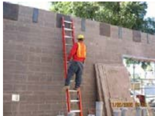
CMU Installation at TPSS No. 5
