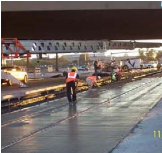
Guide-way Slab Placement under SR143
