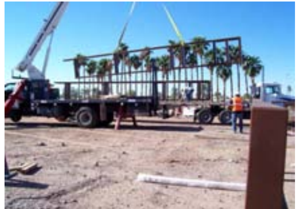
Delivery of the Mast Arms Structures for the LS 4 and LS 5.
