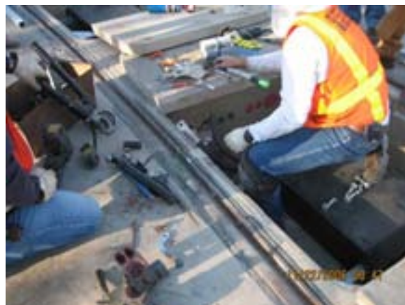
Yard Entrance - Installing Impedance Bond and Connections
