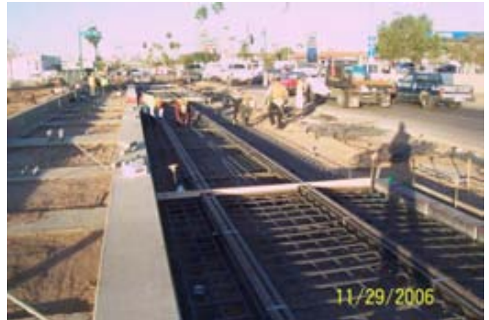
Track Installation at Washington/24 th Street Station
