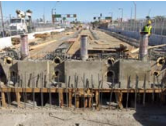
101 Freeway Bridge, Forming for New Center Girder
