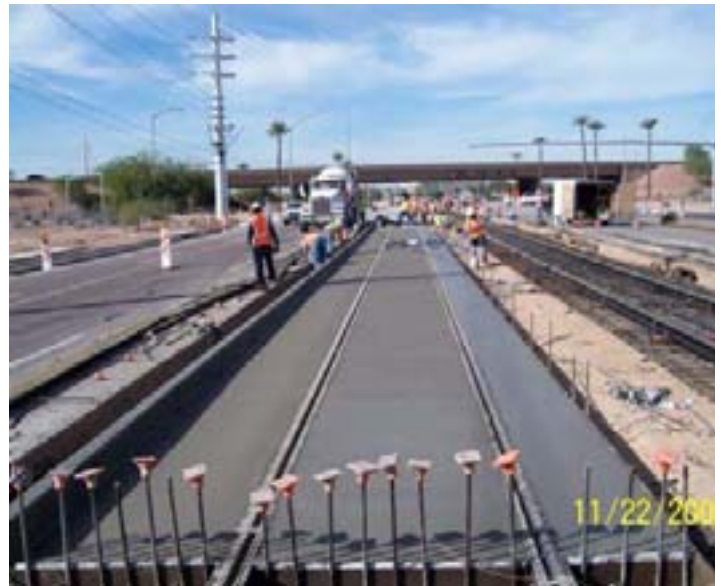
Guide-way Slab Placement 44 th Street to SR143
