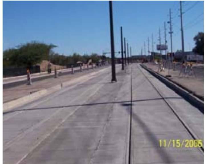
Substantial Completion of the first phase of the Test Track
