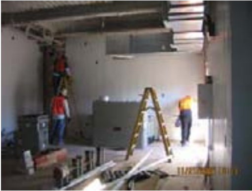
Interior Rough-In at TPSS No. 6
