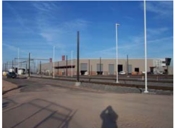
View of the MOE building from the Southeast
