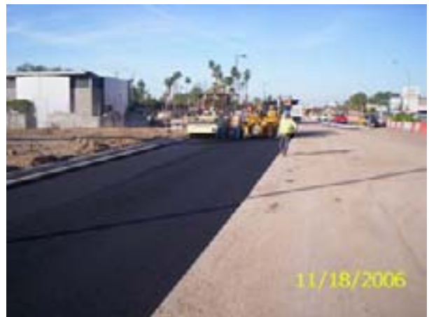
11-18-06 Roadway - Combs Crews Compacting Ac At Sta. 476+00
