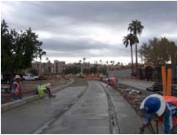
Track Placement, Ash to 1 st St
