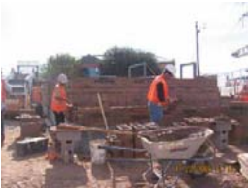
Installation of CMU Walls at TPSS No. 10
