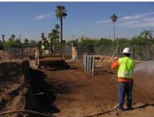
Ductbank Installation at TPSS No. 3
