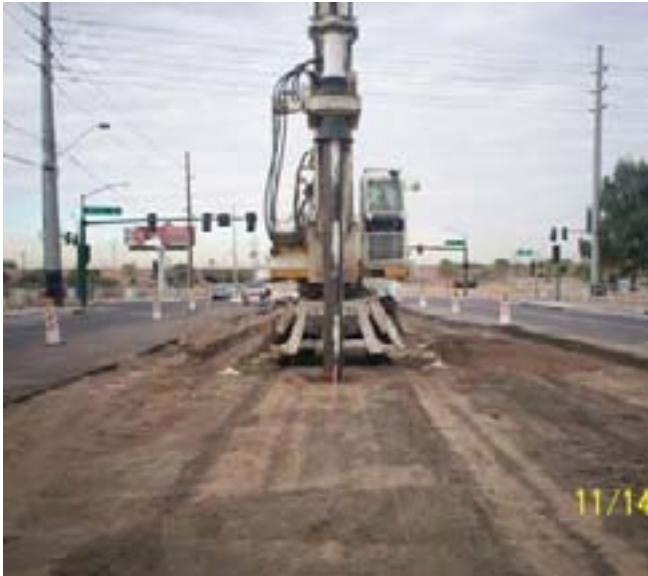
Drilling OCS foundations west of 44 th Street
