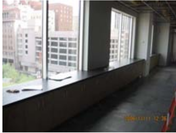
OCC - Completed Cabinetry and Millwork
