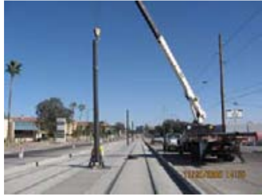
Setting OCS Poles in the Test Track
