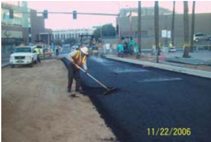
Asphalt Pavement at Jefferson 5th to 7 th Streets
