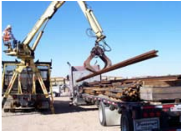
Delivery of the 100m Right Hand Single Crossover for LS2
