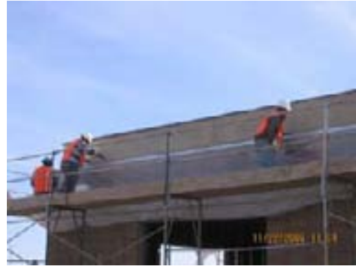
Stucco Application at TPSS No. 7
