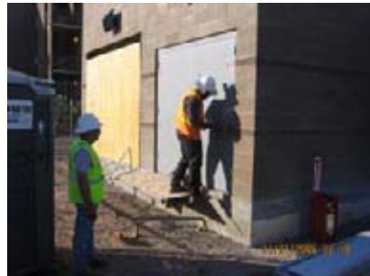
Door Adjustments at TPSS No. 2
