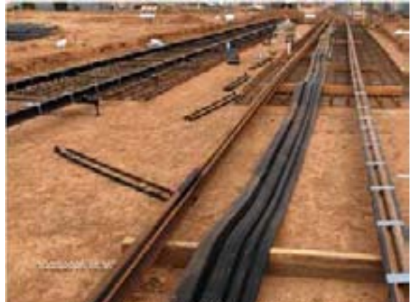
KWC placed rubber rail boot on RH rail of RT-Track 002
