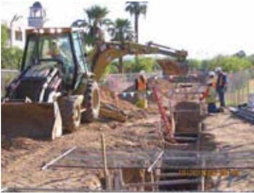
Ductbank Installation at TPSS No. 3
