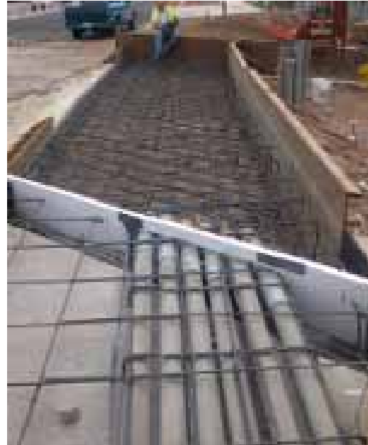
Roadway Work at Tempe Canal Bridge
