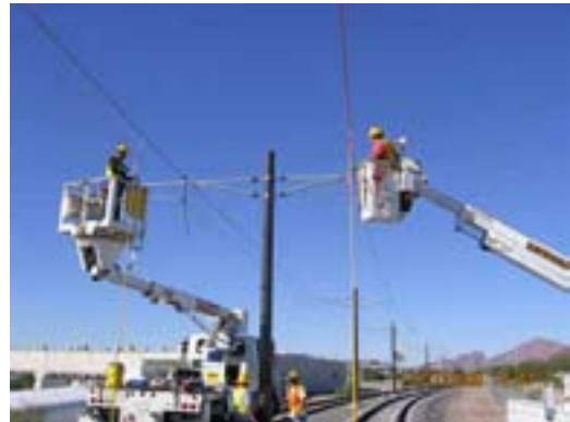
OCS Installations in the MSF Yard
