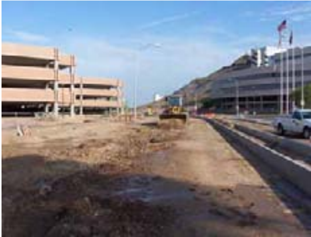
Roadway Work at Veterans' Way
