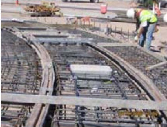
Yard Entrance - Installed TWC Loops
