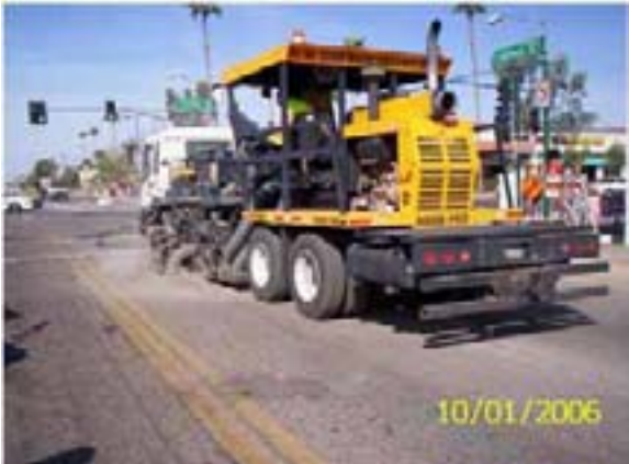
PMU striping obliteration truck east of 7th Avenue and Camelback Road
