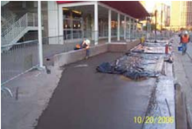
Sidewalk Pavement at USAC
