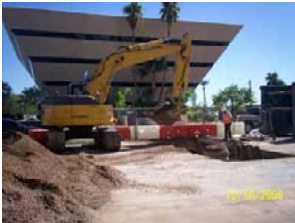
BRB backfilling Manhole 11 Excavation in front of Pyramid Building.
