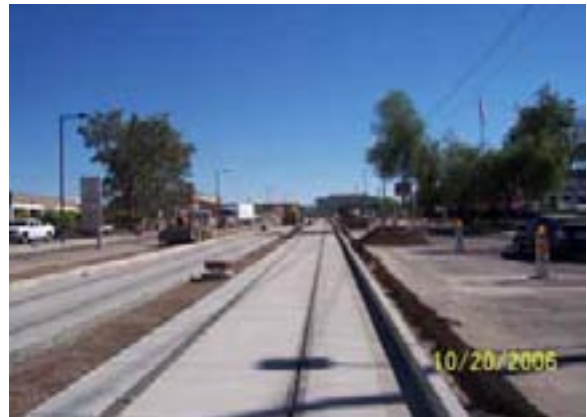
Guide-way between 54 th to 56 th Streets ready for devil strip slabs
