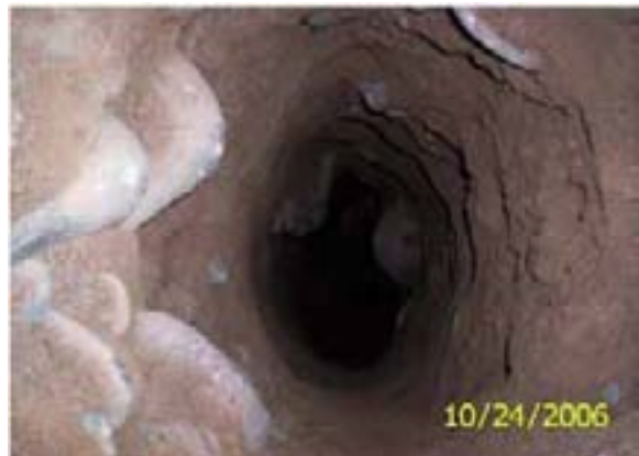
HMS crews pothole at the OCS foundations
