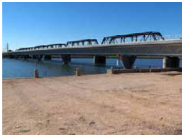
North Bank Restored
