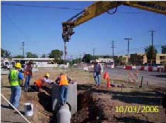
KWC crews installing a precast irrigation structure at STA. 335+68, 54' RT.
