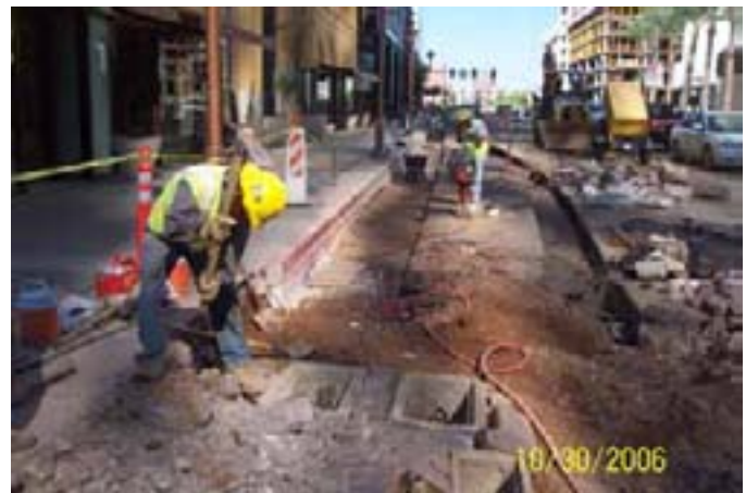
Trench Drain Installation at 1 st Ave/Adams to Monroe
