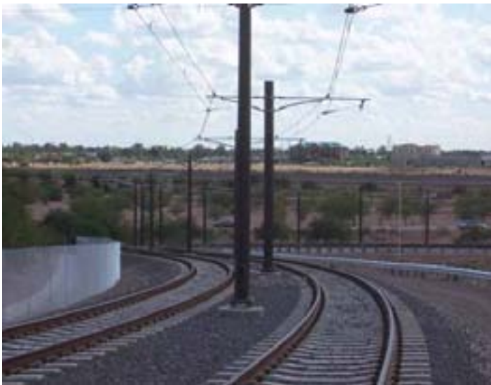
View of the Yard Lead Track and OCS
