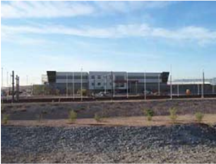
North Elevation of MOE building
