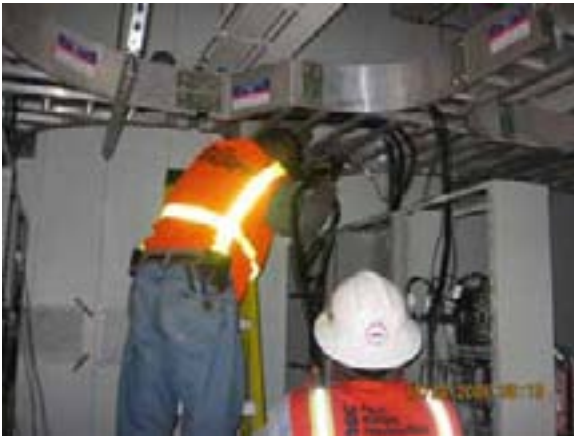
SB No. 3 - Pulling Cable to Signal Racks
