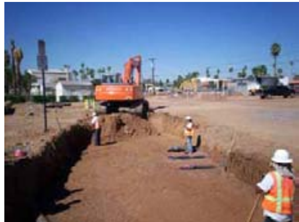
1114+00 platform sub-grade preparation at Camelback Station Site.
