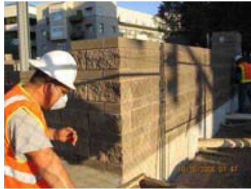
CMU Installation at TPSS No. 5
