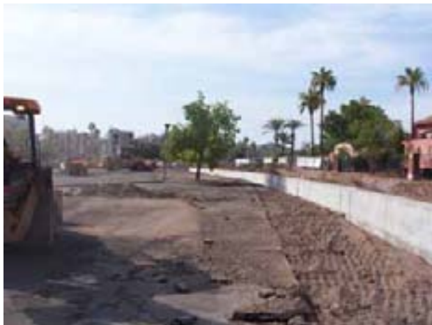
Retaining Wall 5, Ash to First Street
