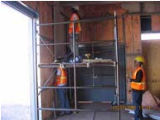
Metal Panel Installation at TPSS No. 1
