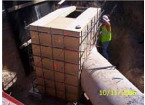
Olsen crews forming SRP Manhole No. 9 at STA. 18+96, LT
