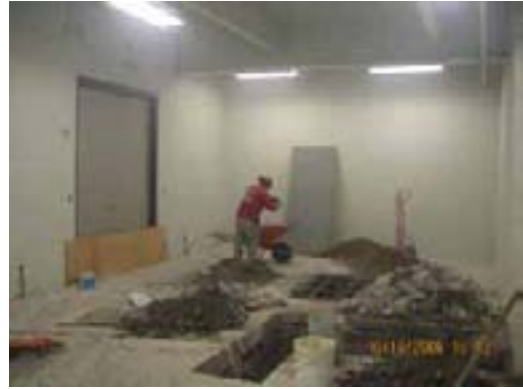
Floor Slab Preparation at TPSS No. 16
