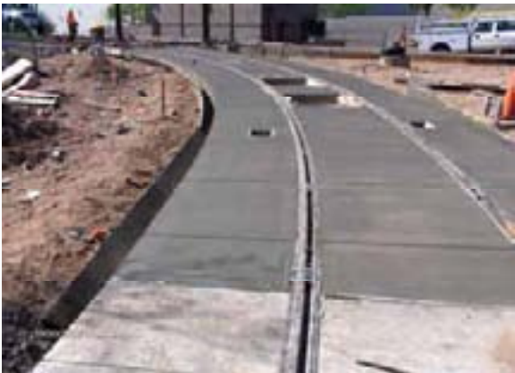
East curve track leading to MSF yard lead track
