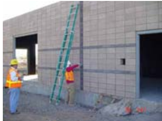
Caulking at TPSS No. 7
