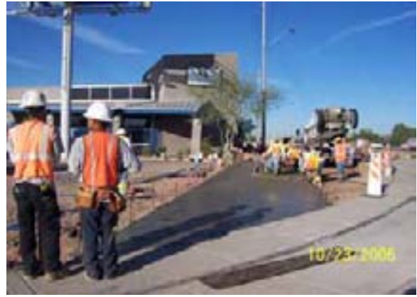
Placing the business access driveway at MSF Yard Lead
