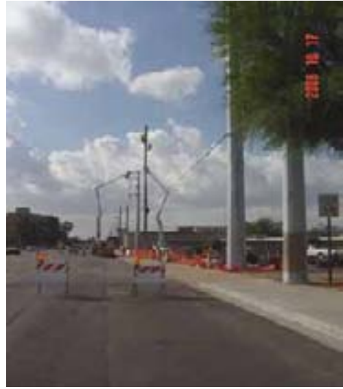
SRP relocating 69 kV at Rural and Tyler in Line Section 5
