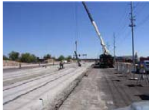
Setting OCS Poles in the Test Track
