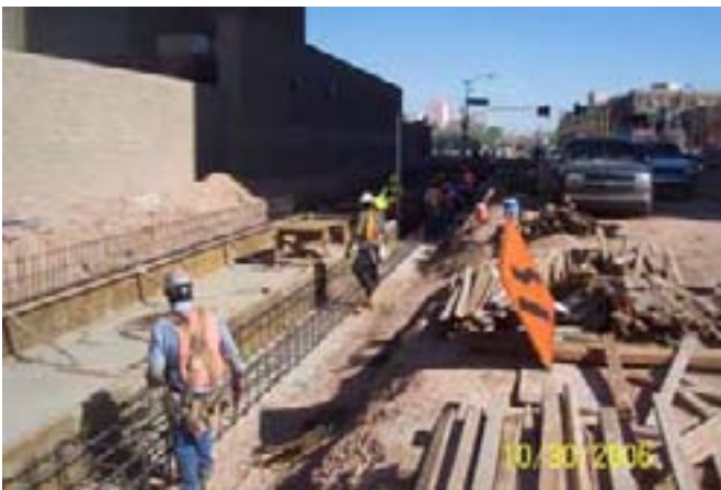
3 rd ST/Washington Station Foundation
