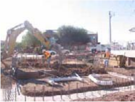
Slab Preparation at TPSS No. 10
