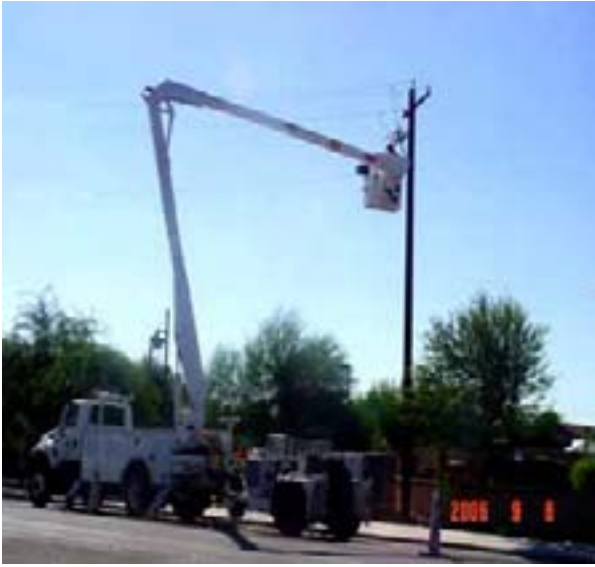
SRP – Temporary Shoo-Fly on Apache Boulevard in Line Section 5
