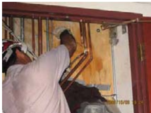
OCC - Installation of Condensate Drain Lines
