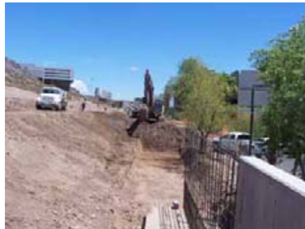
Continuation of Work at Retaining Wall 1
