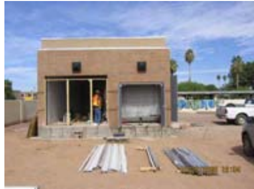
Metal Panel Installation at TPSS No. 2
