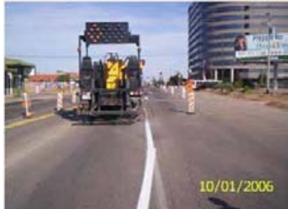
PMU striping truck west of Central Avenue and Camelback Road
