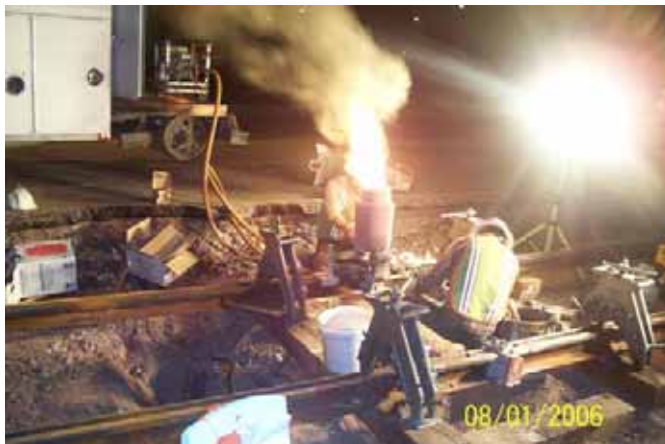
Thermite welding track east of Priest Drive
