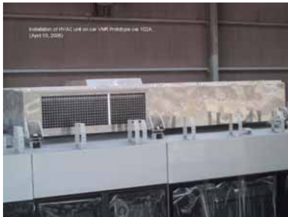
Installation of HVAC unit on roof of METRO prototype car 102A on April 10.
