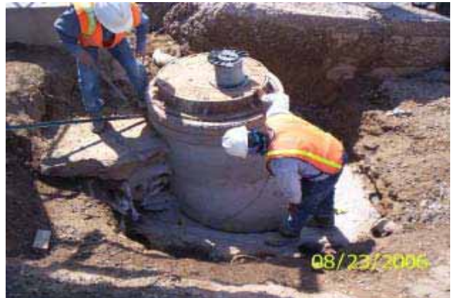
Olsen crews installing turnbuckles on the pressure manhole on Camelback Road
