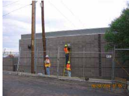
Installation of Exterior Lights at TPSS No. 9
