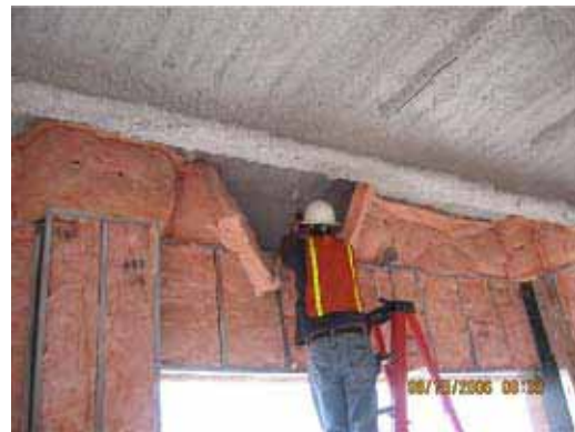
Fireproofing Material Tests at TPSS No. 1
