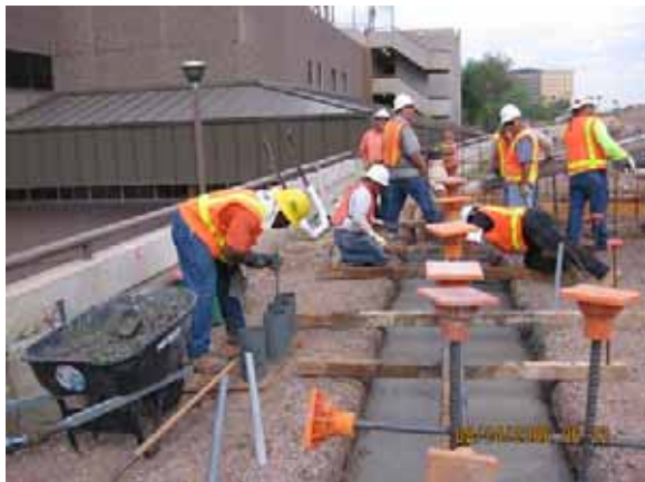
SB No. 6 - Preparing Site for Ground Grid
