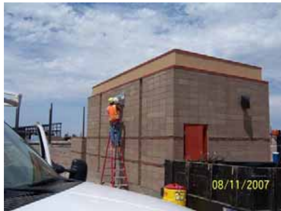
SB No. 5 - Installation of Exterior Components
