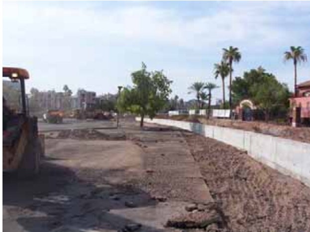
Retaining Wall 5, Ash to First Street
