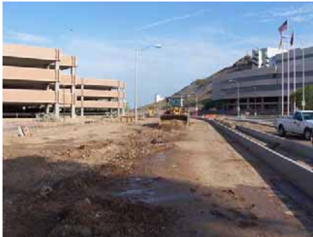
Roadway Work at Veterans' Way
