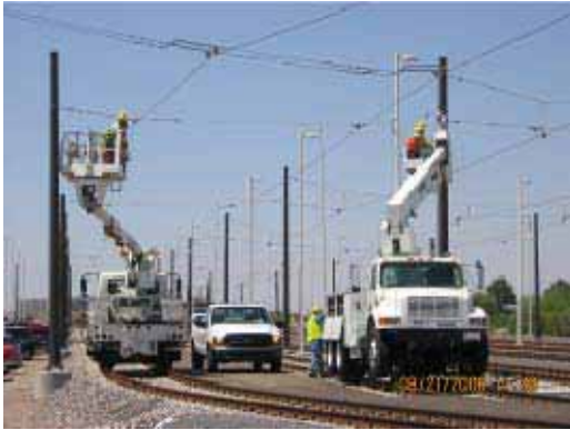
Adjustment of Headspan in the North Yard
