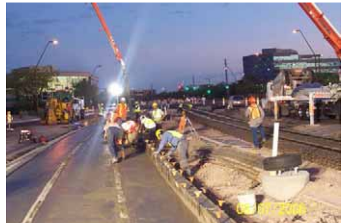
Placement of the right guide-way slab
