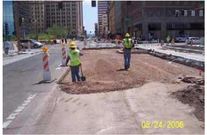
Pavement Preparation Central/Van Buren
