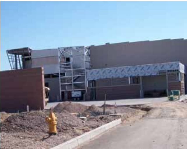
View of the MOE building from the west
