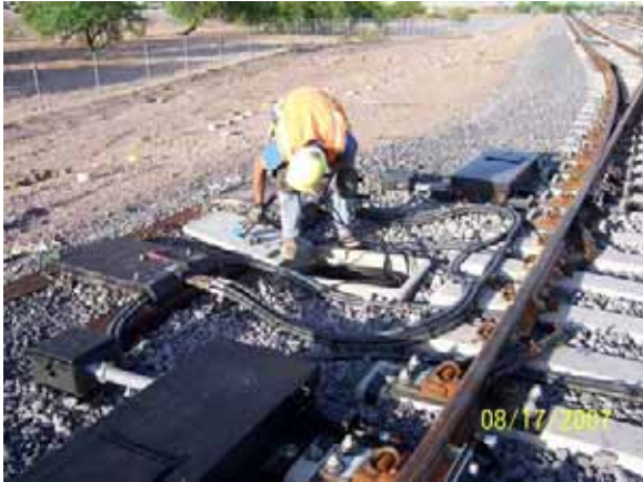
MSF Yard - Terminating Cable for Switch Machines
