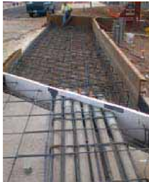
Roadway Work at Tempe Canal Bridge
