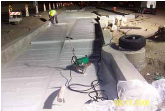
Installation of isolation membrane in special track bathtub
