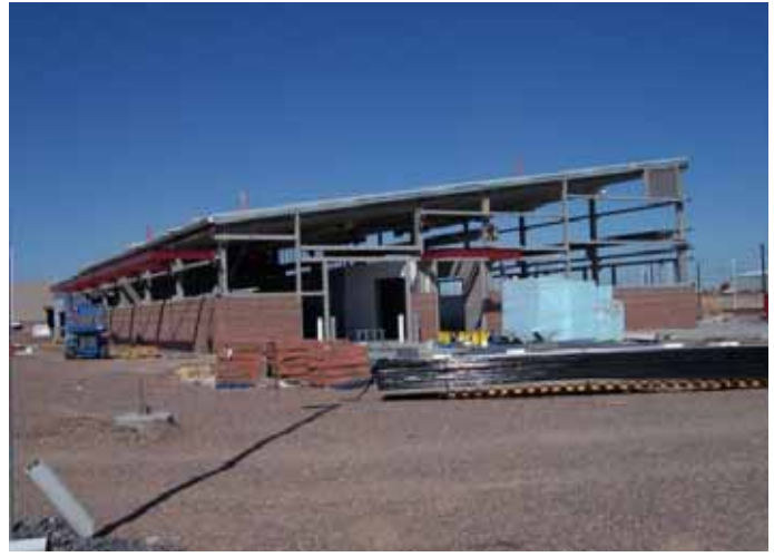
View of the MOW building from the southeast
