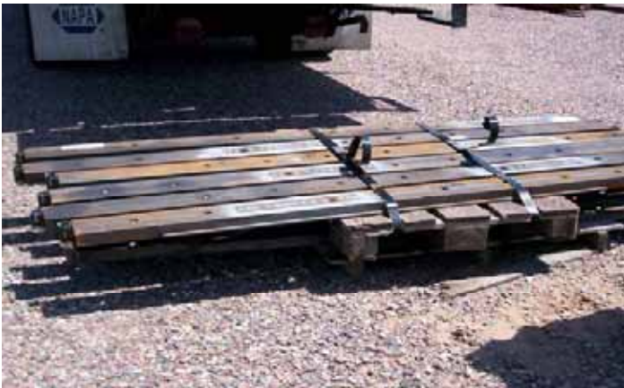
Crossties for Turnout 4-5 and 4-6 that is to be installed on Line Section 4.
