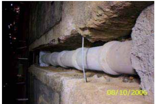
KWC crews installed the 30-inch SRP irrigation line at STA. 453+40
