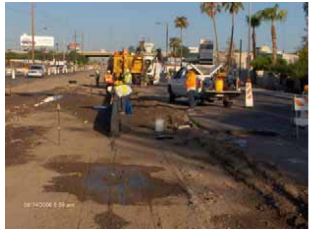
Placement of extruded guide-way curb west of 54 th Street
