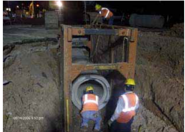
KWC crews installed the 30-inch SRP irrigation line at STA. 453+40
