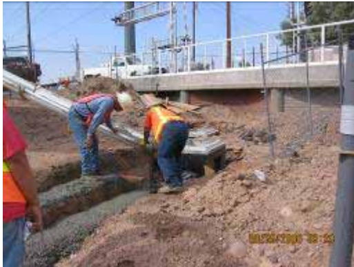
Ductbank Installation at TPSS No. 10
