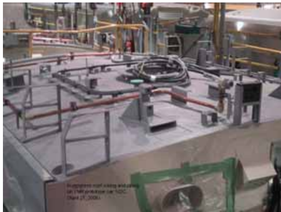
In-progress roof wiring and piping on METRO prototype car.
