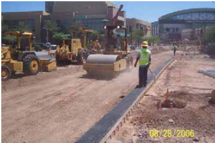
Guideway Preparation Jefferson/2 nd Street
