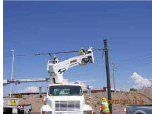
Installation of Deadend in the North Yard
