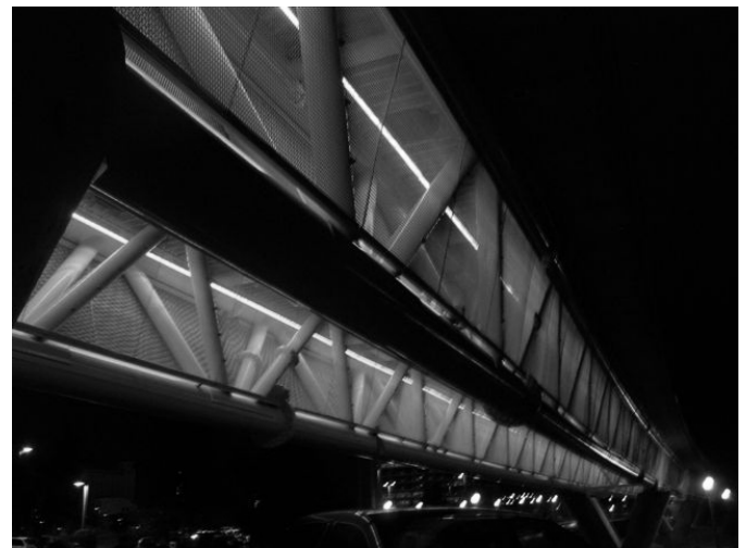
LED Lights in Trusses
