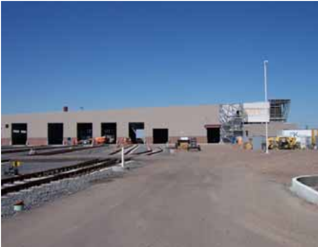
View of the MOE building from the east
