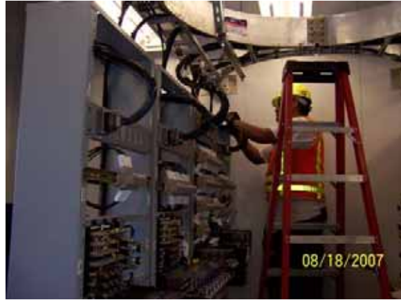
MSF Yard - Wiring Signal System Equipment
