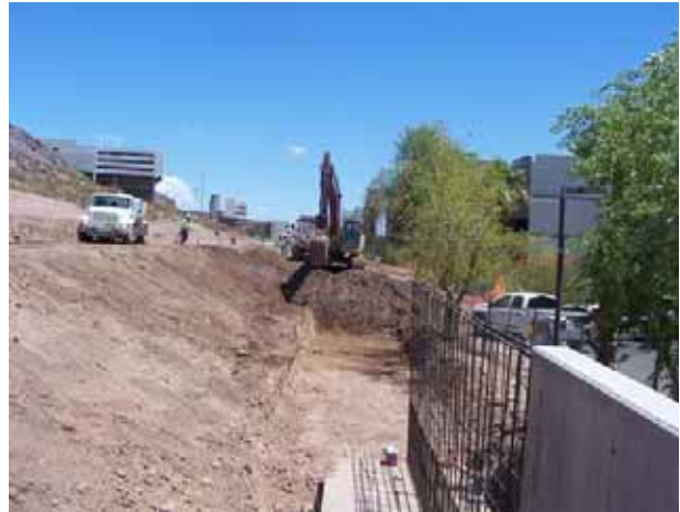
Continuation of Work at Retaining Wall 1
