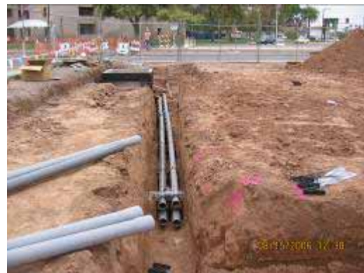
Ductbank Installation at TPSS No. 11
