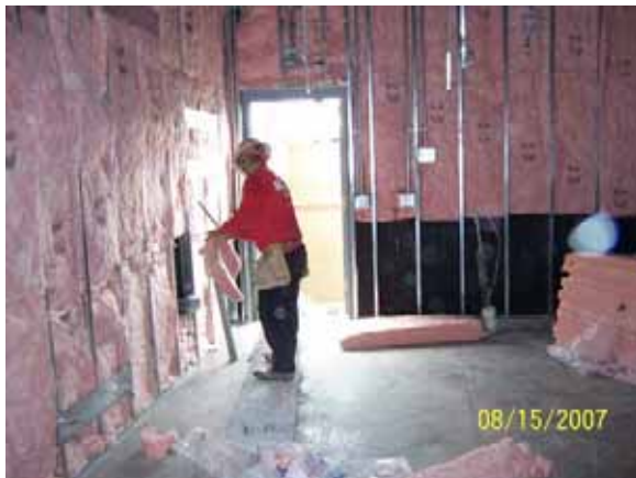
SB No. 3 - Installation of Insulation Material
