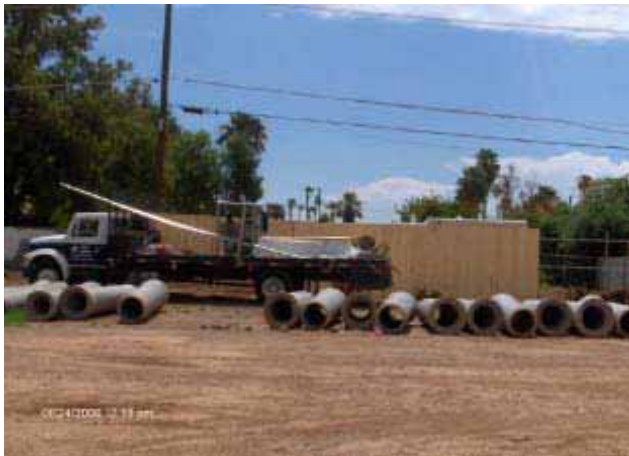
Installing private fence between 7 th and 3 rd Avenue
