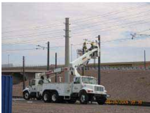
Installation of Cantilever Arm in the MSF Yard
