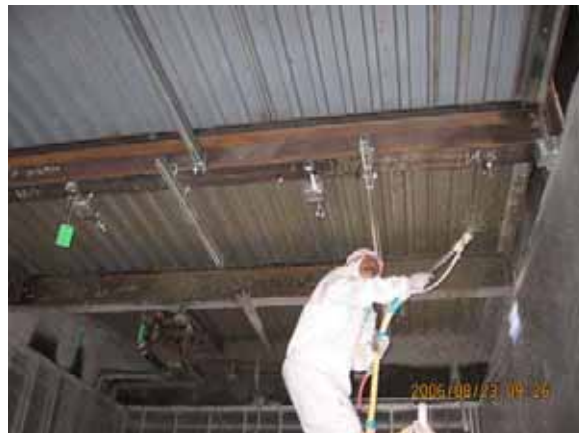
SB No. 4 - Applying SRFM
