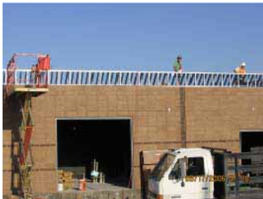
Parapet Framing Installation at TPSS No. 2
