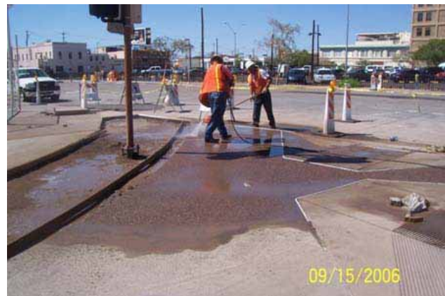
Exposed Aggregate at the US Airway Center Plaza
