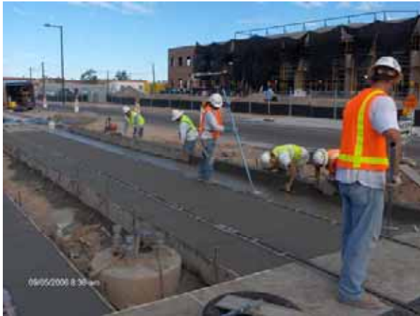
Guideway placement west of 56 th Street
