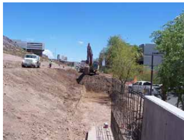
Continuation of Work at Retaining Wall 1
