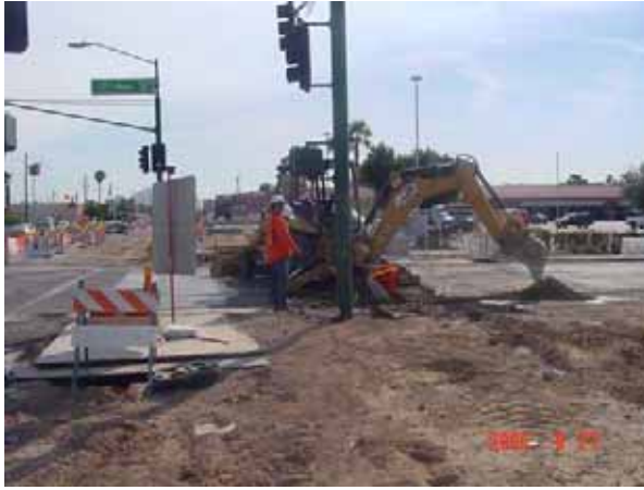
SRP-Power under grounding 12 kV on Camelback Road in Line Section 1
