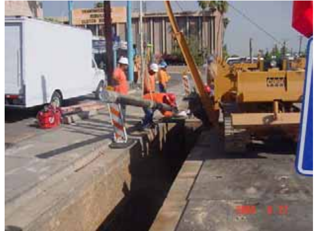
SWG relocation 8-inch High Pressure Gas Main on 19 th Avenue in Line Section 1
