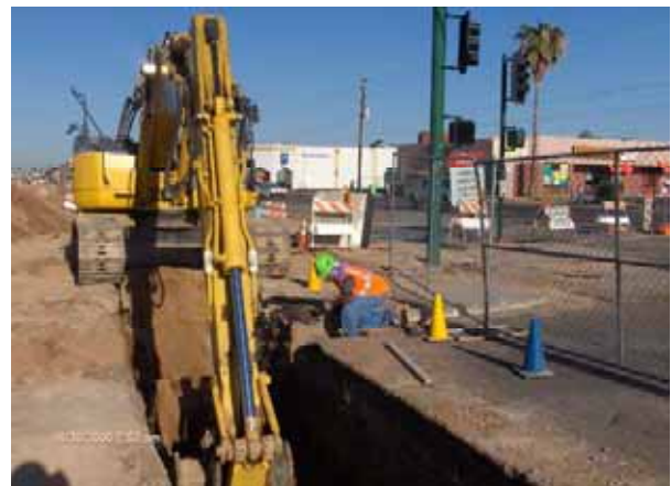
KWC Excavating for the New SRP 30-inch RGRCP Across 17 th Avenue
