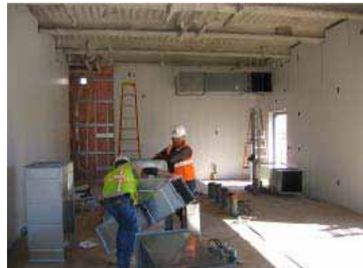
Ductwork Installation at TPSS No. 6
