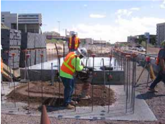
SB No. 6 - Compacting for AC Pad
