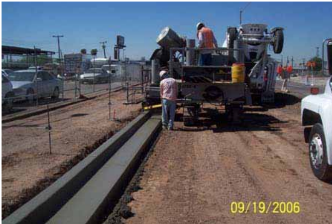
Curb and Gutter at Jefferson Between 24th and 25th Street
