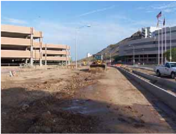
Roadway Work at Veterans' Way
