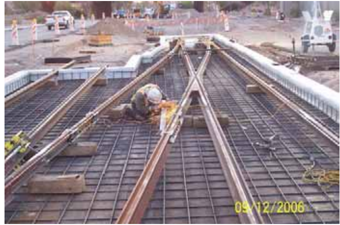
4-5/4-6 Single Crossover Construction
