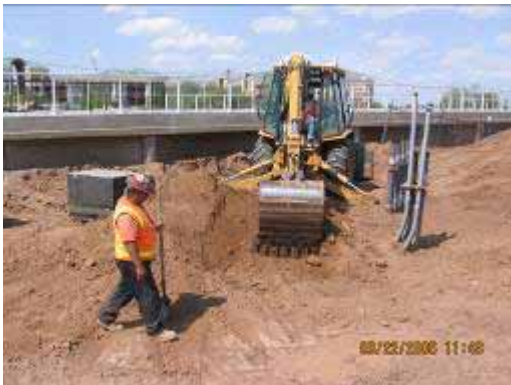
Grading work at TPSS No. 10
