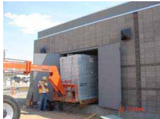
Installation of Rectifier into TPSS No. 9
