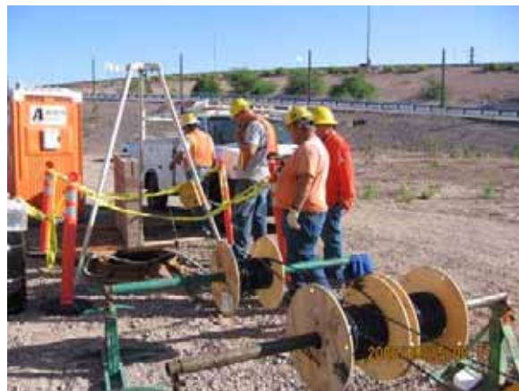
SB No. 5 – Installation of 480V Power Cable
