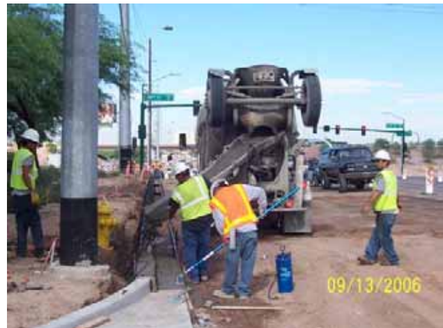
Placement of curb/gutter east of 48 th Street
