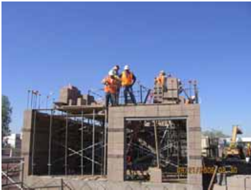
2 nd Lift of CMU Walls at TPSS No. 7
