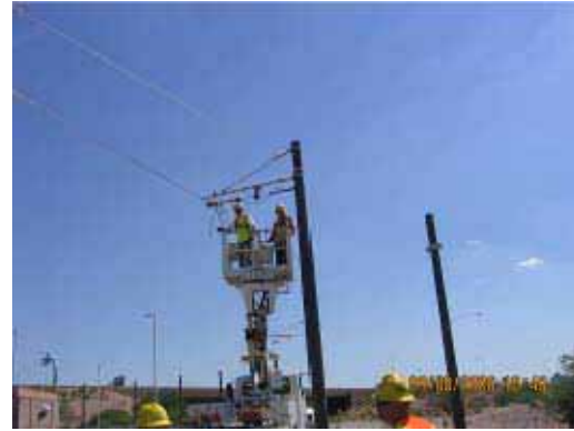
Cantilever Arm Installation at MSF Yard
