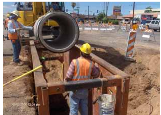
KWC Installing the New 30-inch SRP at 415+50
