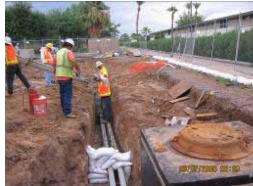
Concrete Encasement of Negative Ductbank at TPSS No. 11
