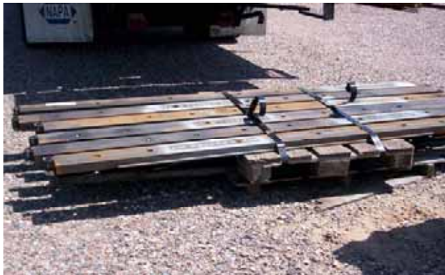
Crosssties for Turnout 4-5 and 4-6 that are to be installed on Line Section 4
