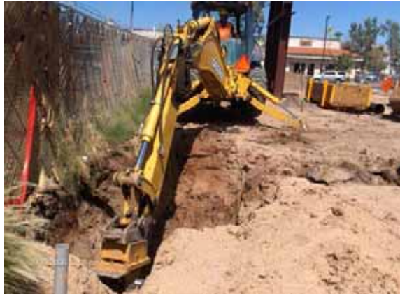
KWC Backfilling the Open Excavation Material Removed at 450+75 RT
