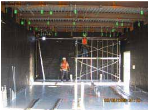
Metal Stud Framing at TPSS No. 2
