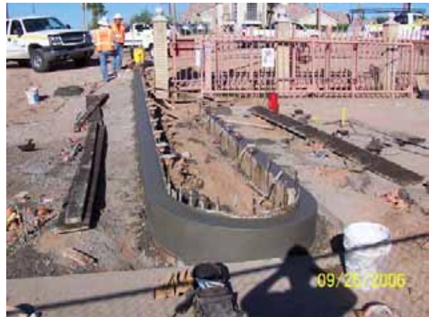
Newly poured curb return at Minnezona.
