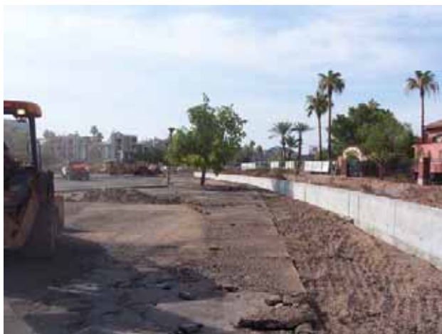
Retaining Wall 5, Ash to First Street
