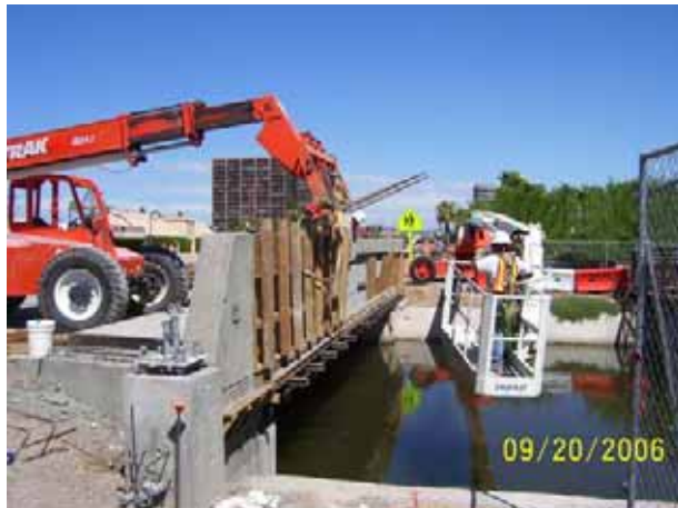
Stripping forms of the bridge barrier wall at GCB
