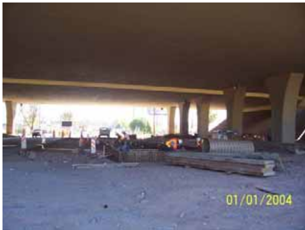
Forming 4-8 Turnout Bath Tub to MSF Yard Lead Track
