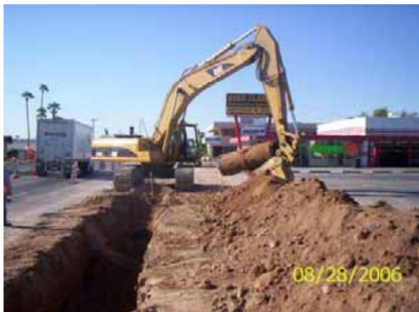
KWC Crews Removing SRP Irrigation Line on 19 th Avenue
