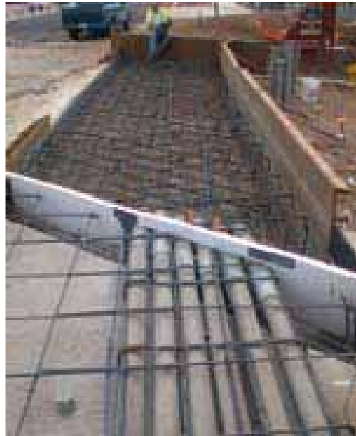
Roadway Work at Tempe Canal Bridge
