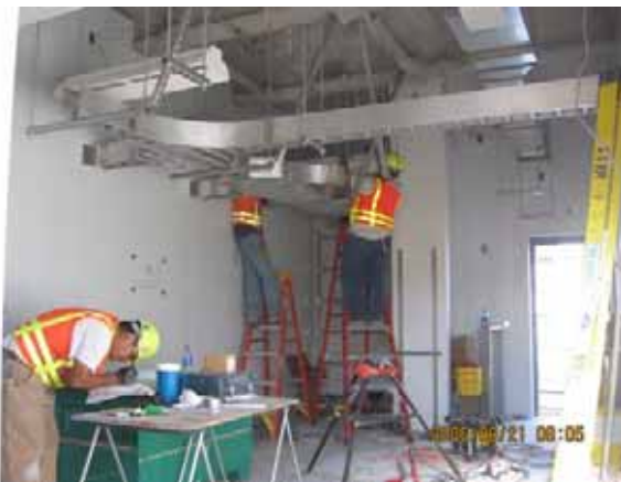
SB No. 3 - Installation of Overhead Cable Trays
