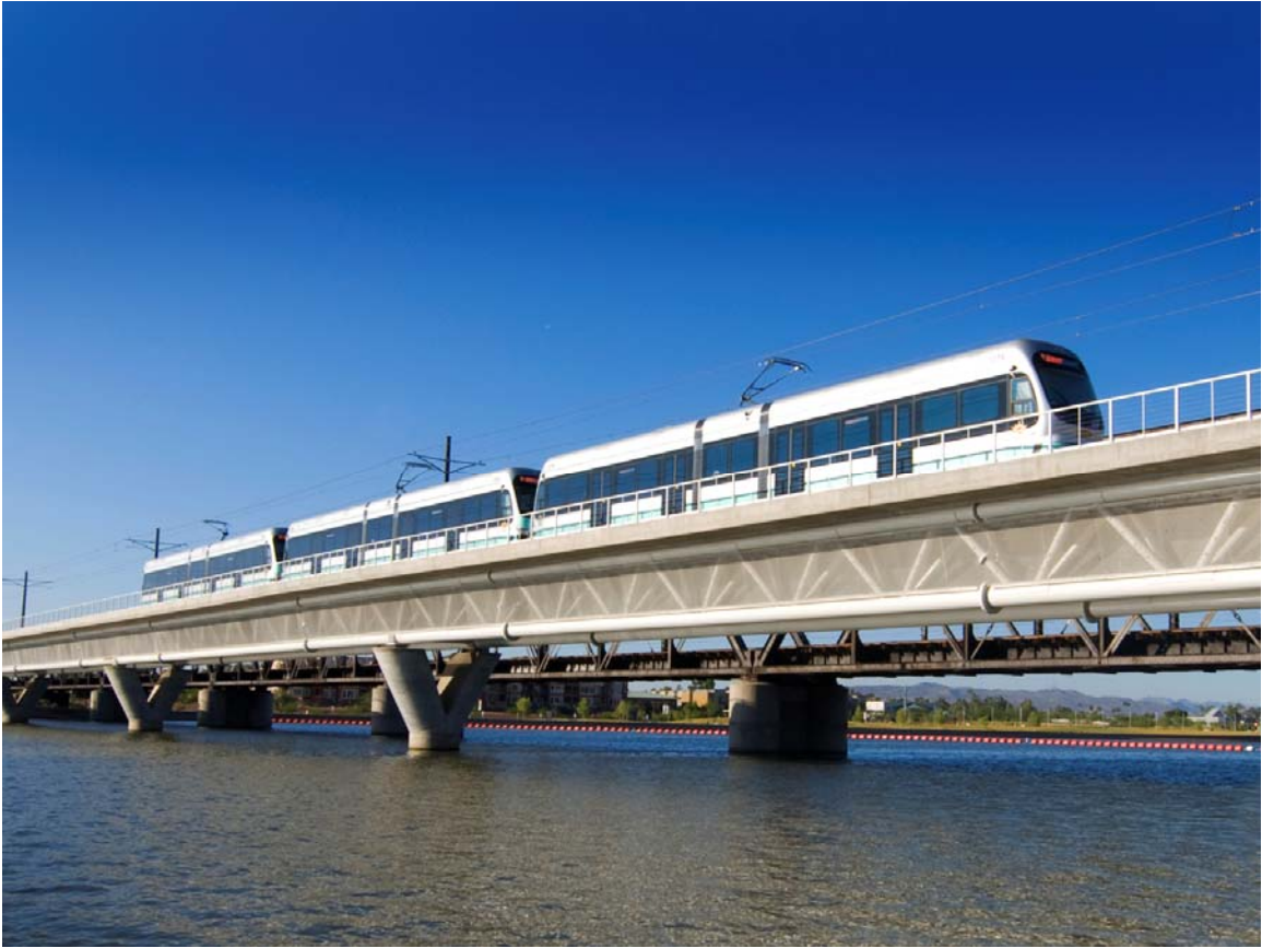
A METRO three-car train on the Tempe Town Lake Bridge
