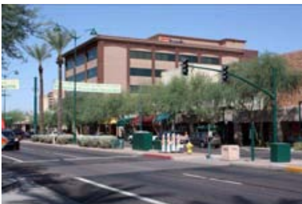
PHOTO 21: Mid-block crossing at One MacDonald Center looking northwest
