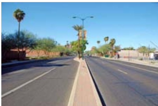
PHOTO 39: Mesa Drive looking east
