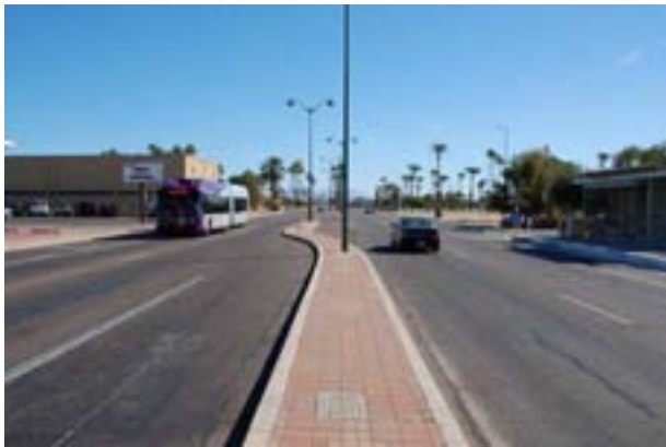
PHOTO 40: Mesa Drive looking east
