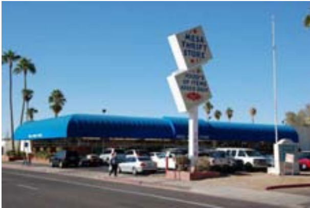
PHOTO 12: Mesa Thrift Store, looking northwest
