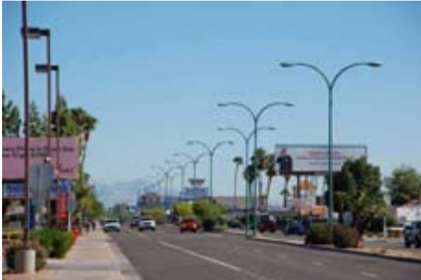
PHOTO 6: Main Street at Alma School looking east
