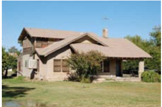
PHOTO 13: Standage House looking north
