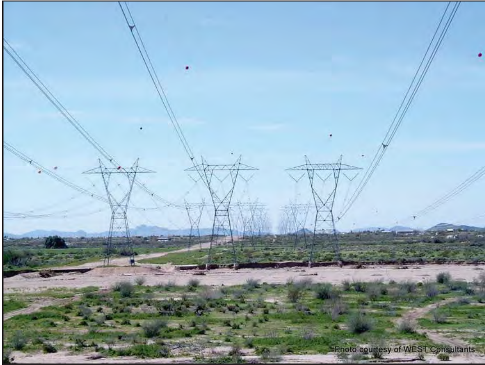
Overview of channel at SRP poles
