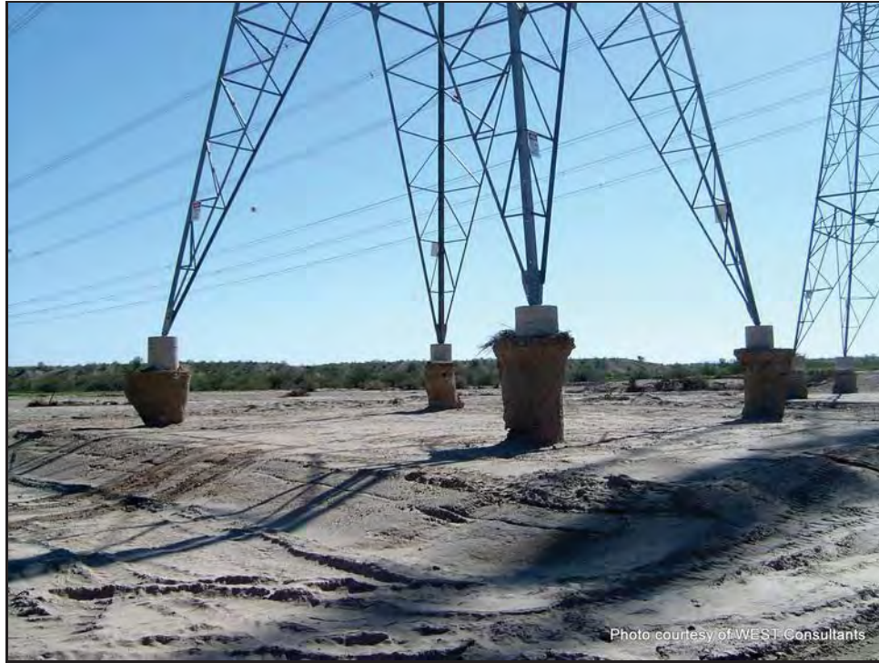
Channel erosion at SRP poles
