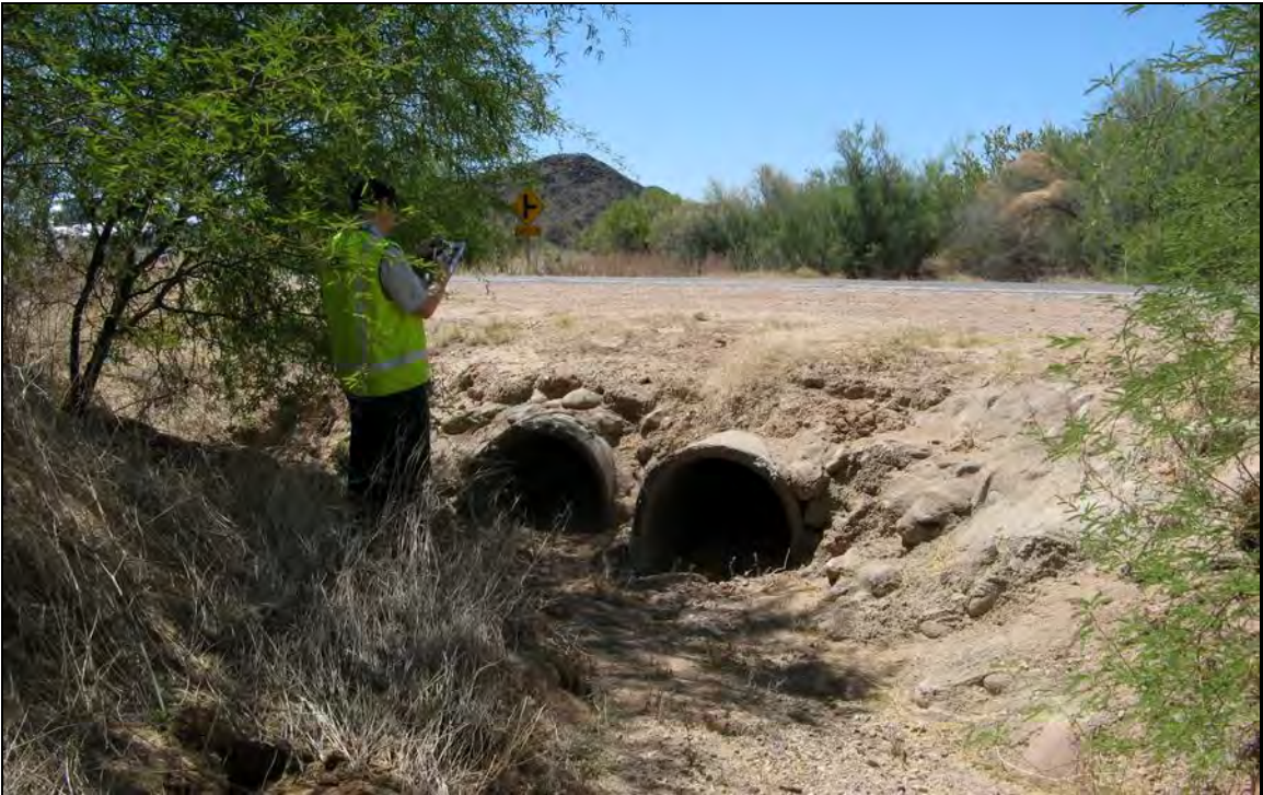
722: D/S at Fourmile Wash culverts
