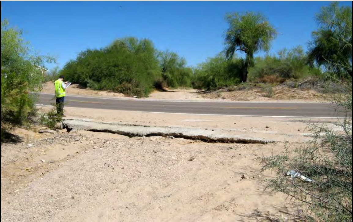
690: U/S at Dickey Wash crossing
