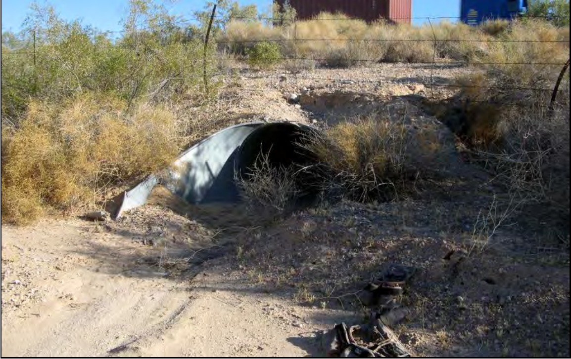
638: U/S at I-10 Culvert
