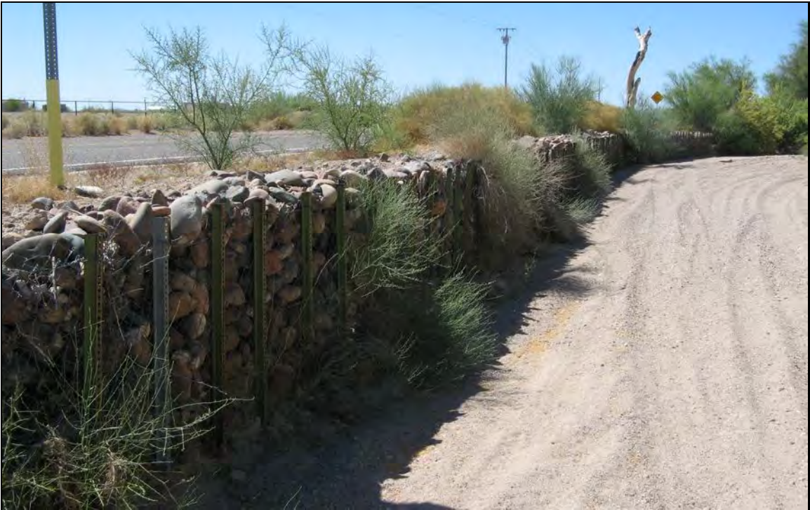
700: D/S at gabion lining along L Bank of Phillips Wash
