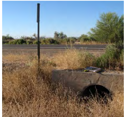
Culvert near Palo Verde Road
