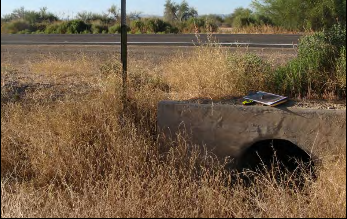
624: Culvert near Palo Verde Rd
