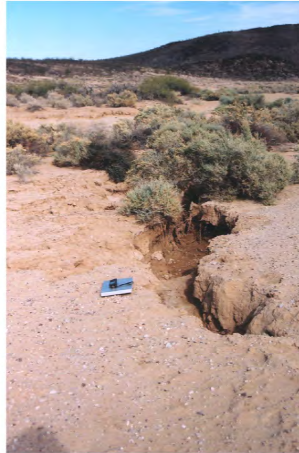
Figure 10. Typical crack, near north end of main cluster.
