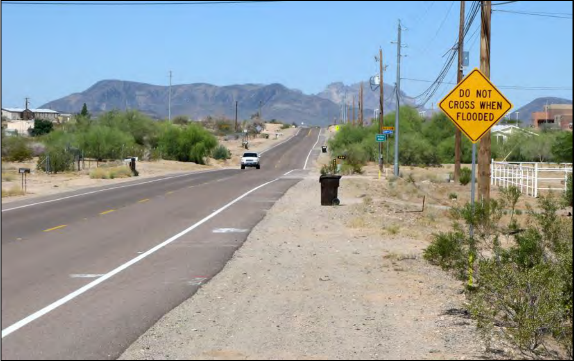
687: W towards Dickey Wash crossing
