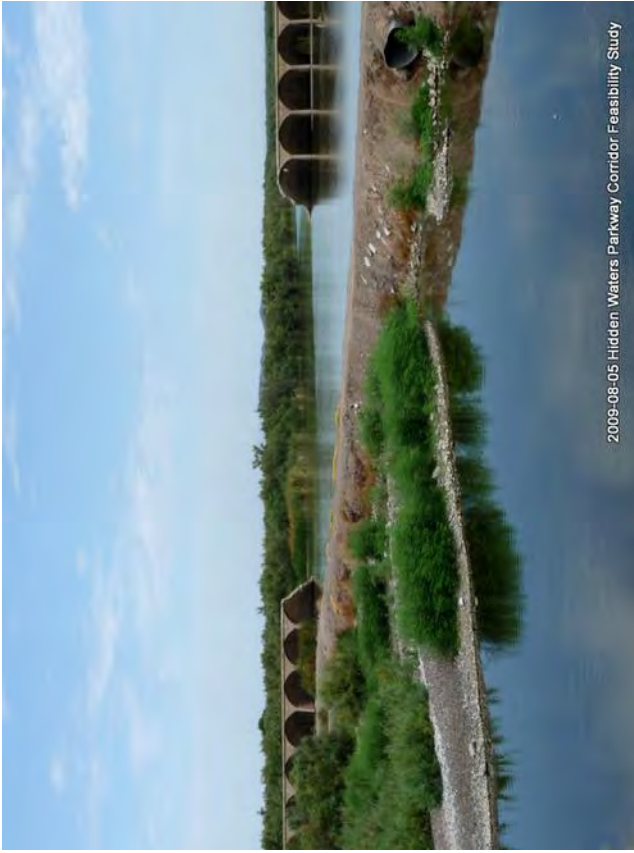
Photo 0333: Looking upstream at Gillespie Dam breach
