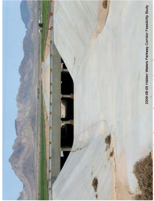
Photo 0314: New Box Culverts Crossing of Old US 80 at Layton Wash
