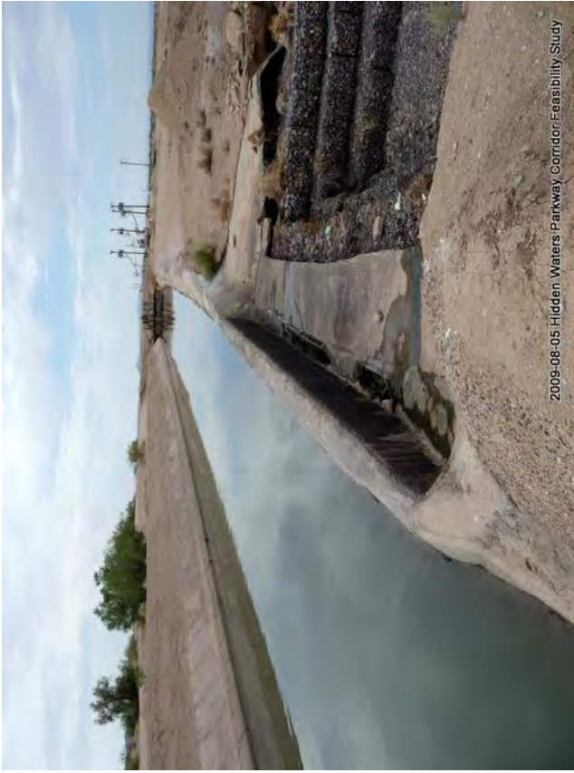
Photo 0302: Overflow overshoot of Gila Bend Canal
