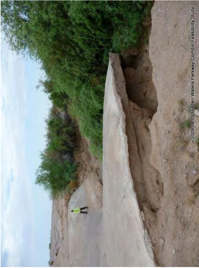
Photo 0288: Downstream section and erosion at Gila Bend Canal...
