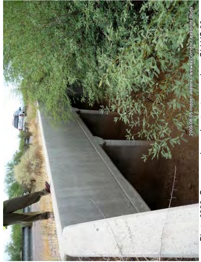
Photo 0338: Overgrown box culvert entrance along Old US 80
