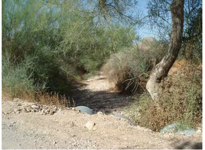
304: Culverts at 387th Ave
