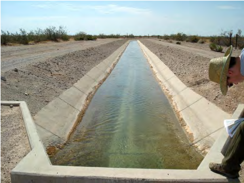
310: Tonopah Irrigation District Canal
