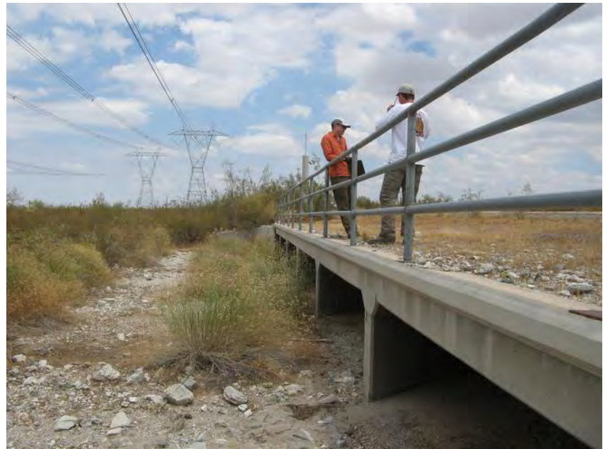
609: White Tank Wash box culverts at Sun Valley Parkway
