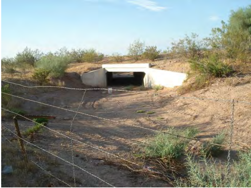
256: I-10 entrance ramp box culvert (near 411th Ave)
