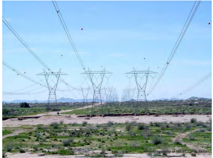
Overview of channel at SRP poles
