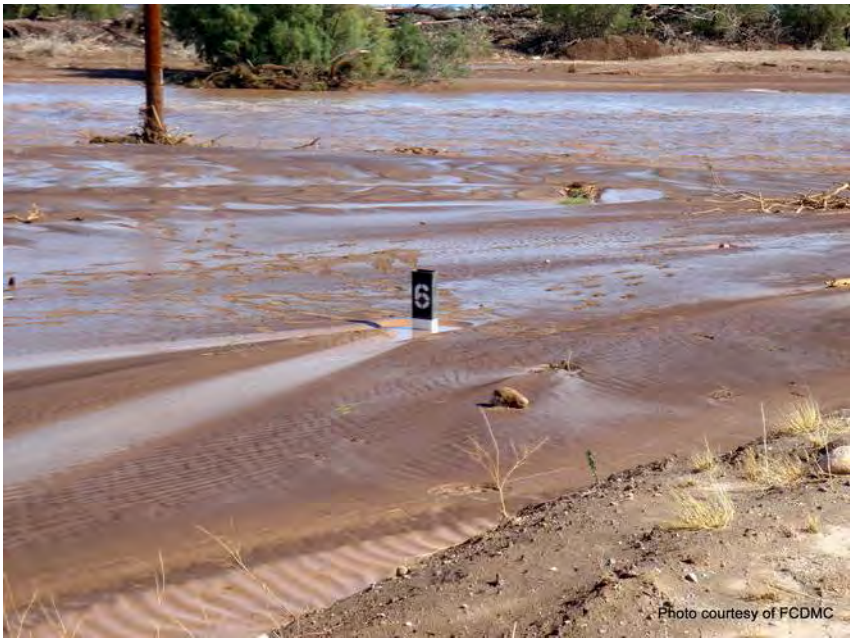
Sediment deposition at Tonopah Salome Highway
