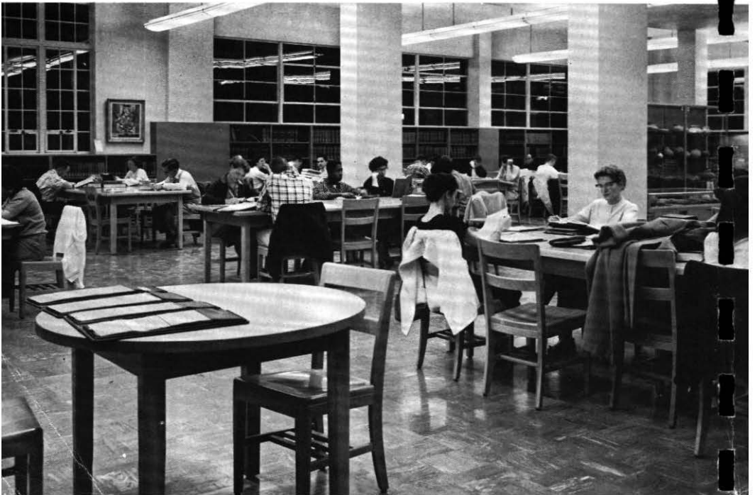
Matthews Library, now utilizing seven stacks, also provides spacious reading rooms. In addition to furnishing all library services, this building houses an extensive curriculum laboratory and the notable Collection of American Art.
