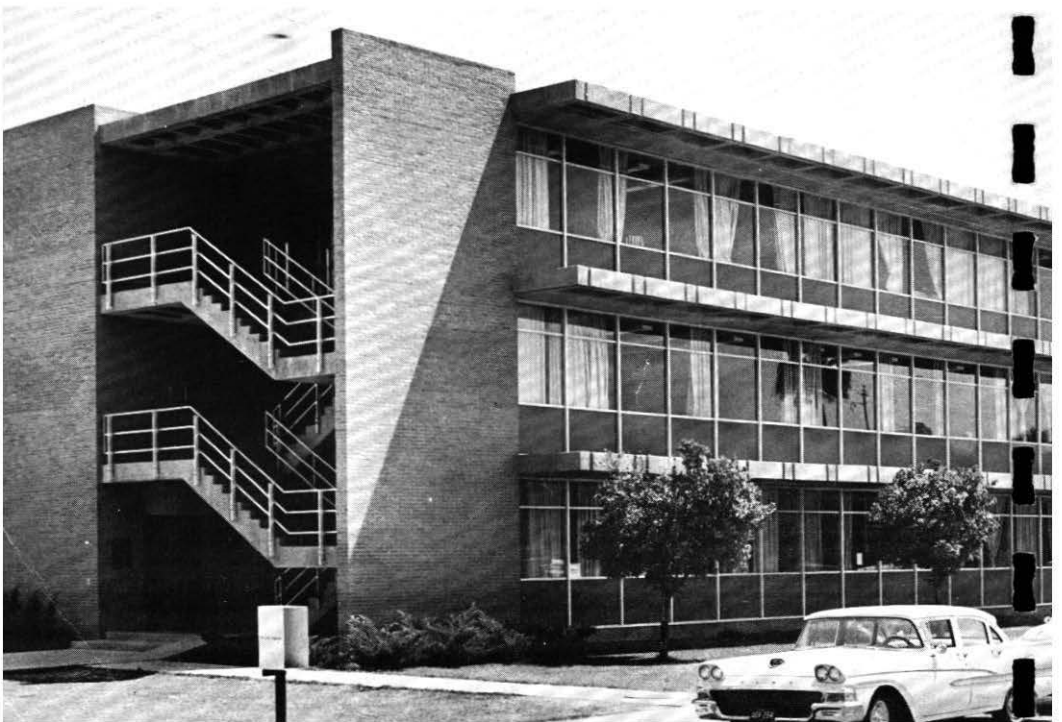
The three-story classroom wing of the new multi-unit Engineering Center is pictured above. Construction included the use of the lift-slab technique. Inner walls are of unfinished block and concrete.
