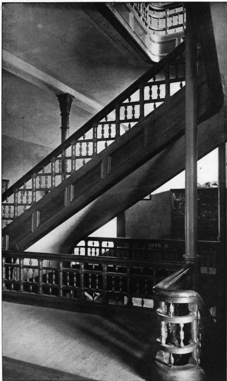
STAIRWAY IN NORMAL BUILDING
