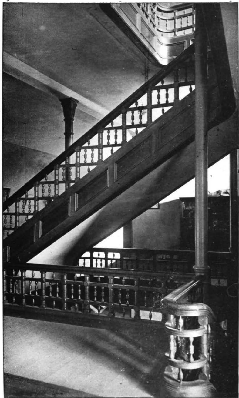
STAIRWAY IN MAIN BUILDING
