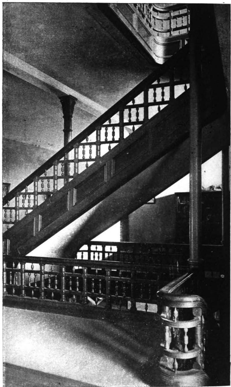
STAIRWAY IN MAIN BUILDING
