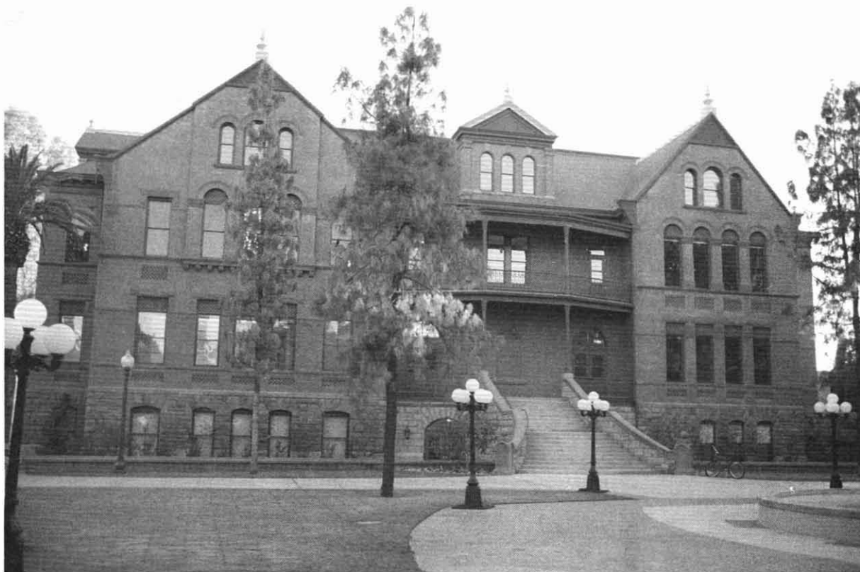
Old Main after the completed restoration of 2000.
